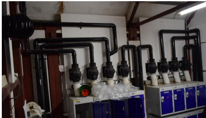
The system used at Jorvik Centre to produce and emanate smells on site (2018) fig 7.48
