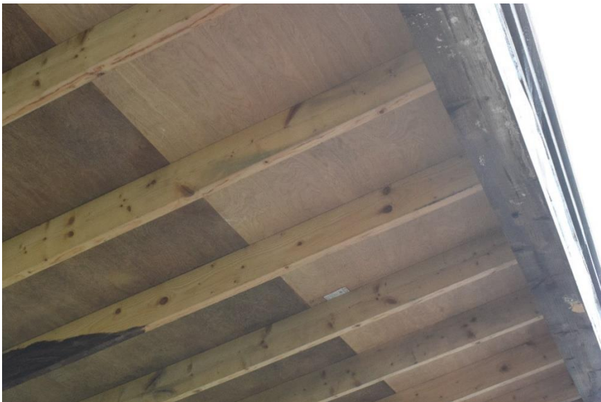
2x4's and plywood ceiling (2017) fig 5.49
