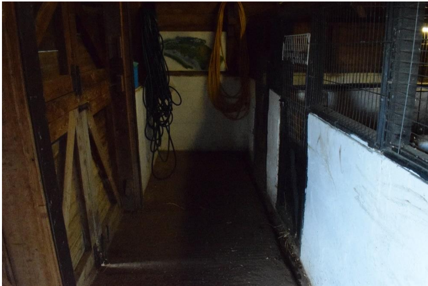
Farm building interior with concrete floor and other modern features (2017) fig 5.48
