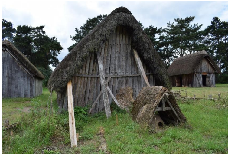
'The Oldest House' supported from collapse. West Stow, UK (2016) fig 3.4
