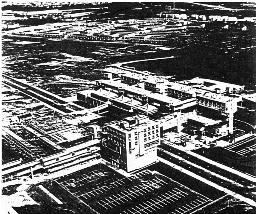
3-6. c) Cumbernauld: Town centre, only 1/5 of the proposed centre was completed.
