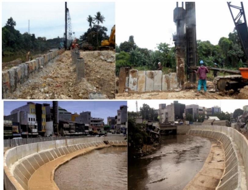
Figure 9. (Top photo) Construction process of concrete pile sheet installation on site (Bottom photo) Finished concrete embankment in Kampung Pulo, East Jakarta (Source: Documentation provided by National River Agency (BBWSCC))
