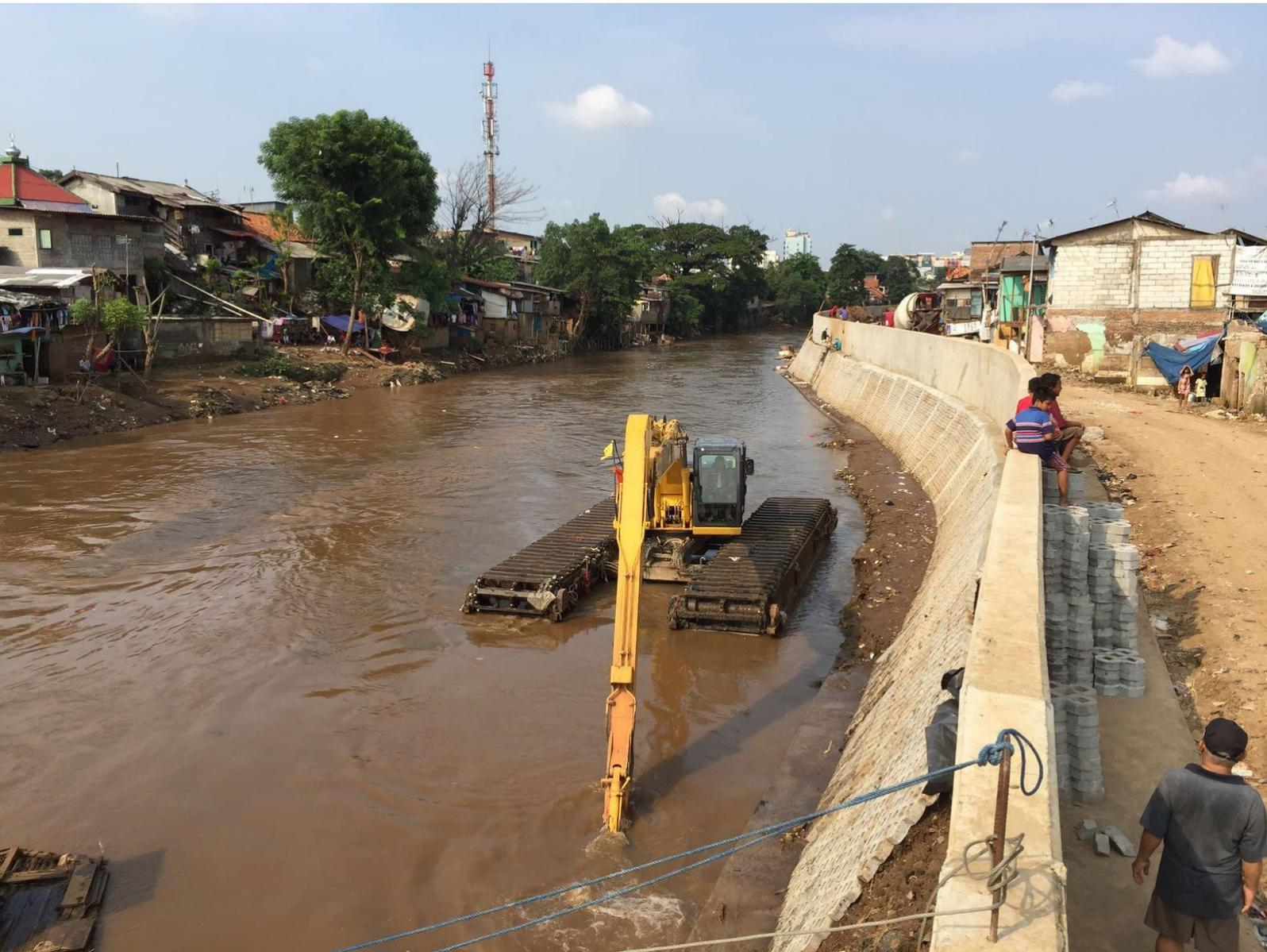
Figure 41. The Public Works Agency-employed contractor developing a concrete river terrain with inspection pathways in the right side at the end of 2015. (Source: the author's documentation)
