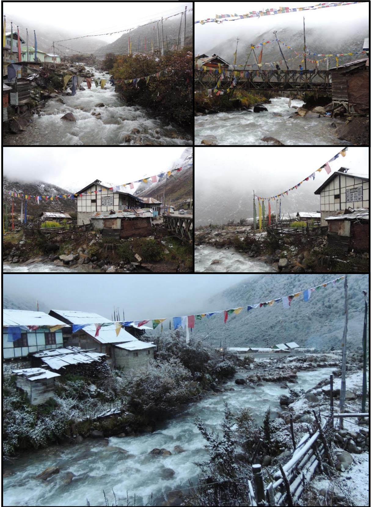
Fig 5.17. The GLOF-susceptible Jáchú River flows through Thánngũ, with high-risk properties (located less than 10 metres above the river bed) along both banks; the Army helipad and camp are seen on the left bank of the river at the far end of the bottom image (photo credit: Vaibhav Kaul, 2015).
