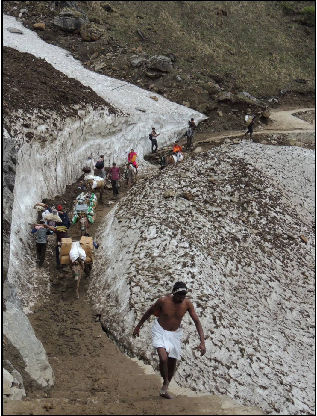
Fig 5.26. A section of the newly constructed post-disaster pilgrims' trail to Kédārñāth that has been carved through a perennial firn pack occupying a mountain torrent channel over which winter avalanches regularly slide (photo credit: Vaibhav Kaul, 2016)
