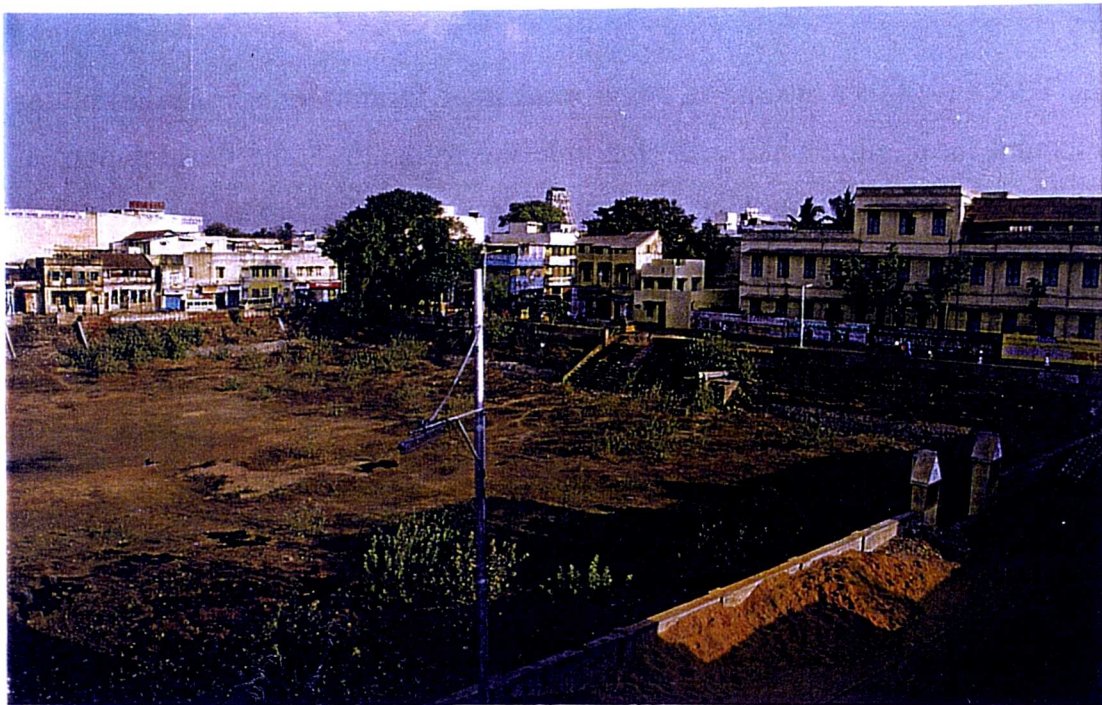
Figure 33 The dilapidated Kesavaperumal Temple Tank (bottom), the Kapaleeshwar Temple Tank (above) and other structures showing changing land uses in the Heritage Zone.
