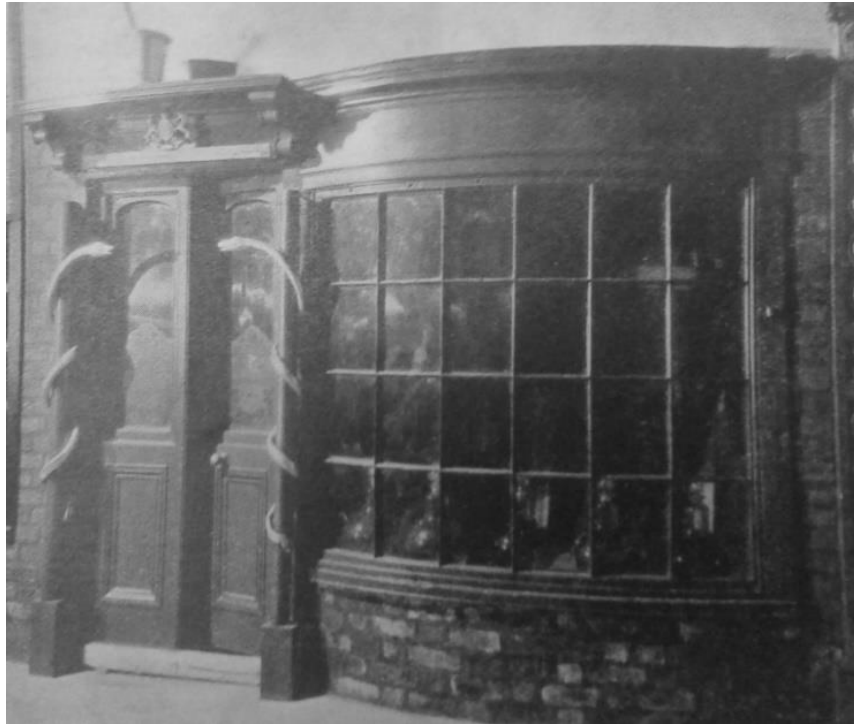
Figure 2.6: Window display of chemist's shop on the Old Times Street (1935) 134
