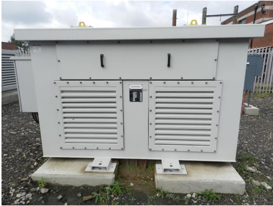
Fig. 4.9 A 2.1 MVA transformer used in WESS.
