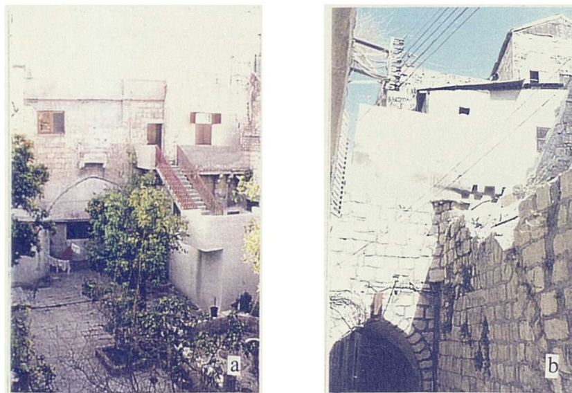
Fig. 4.7 (a): Cheap Building Materials are Replacing Stone the Traditional Material. (b): Additions to Old Buildings Spoiled the Image of the Traditional Settlements. Source: the author
