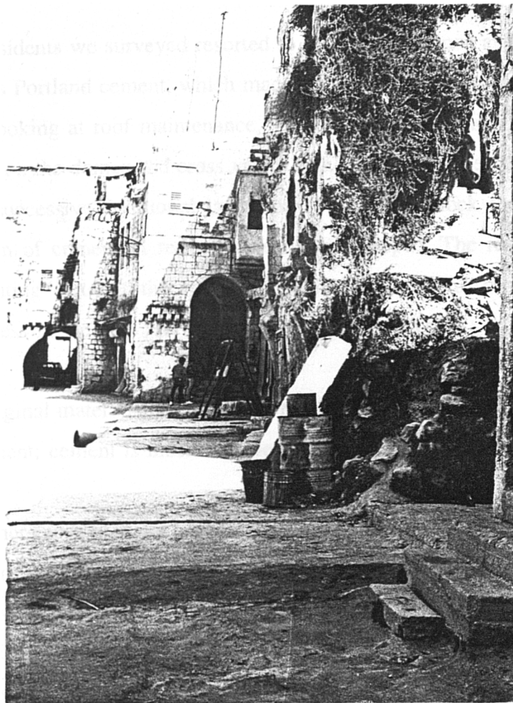
Fig. 7.16: Ruined Buildings are Side by Side to other Buildings of Good State of Repair. Source: Courtesy Mr Salim Jadallah, Nablus 1989.
