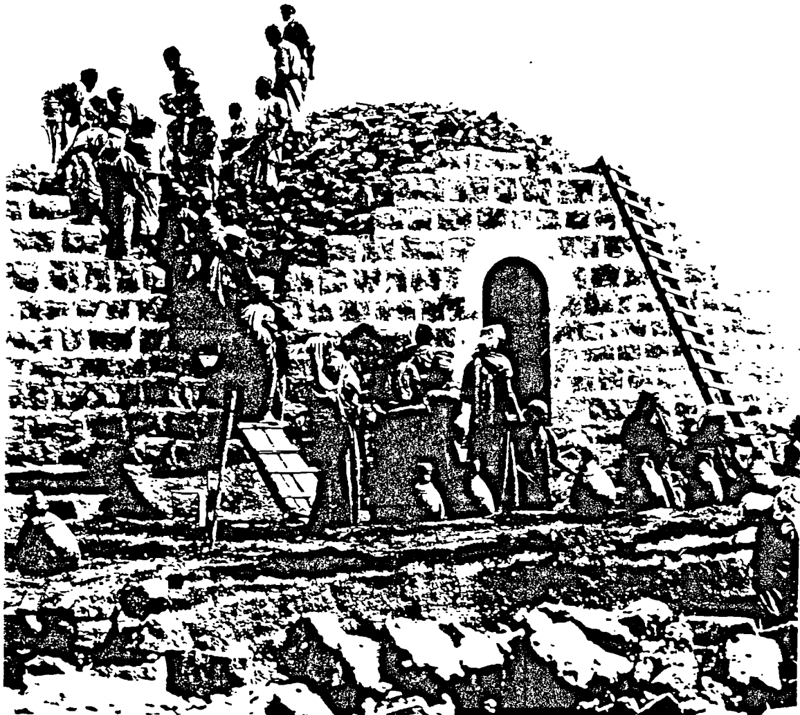
Fig. 2.1: Building a Stone House in a Palestinian Village by a Collective Effort. Source: Graham-Brown (1980: 37).
