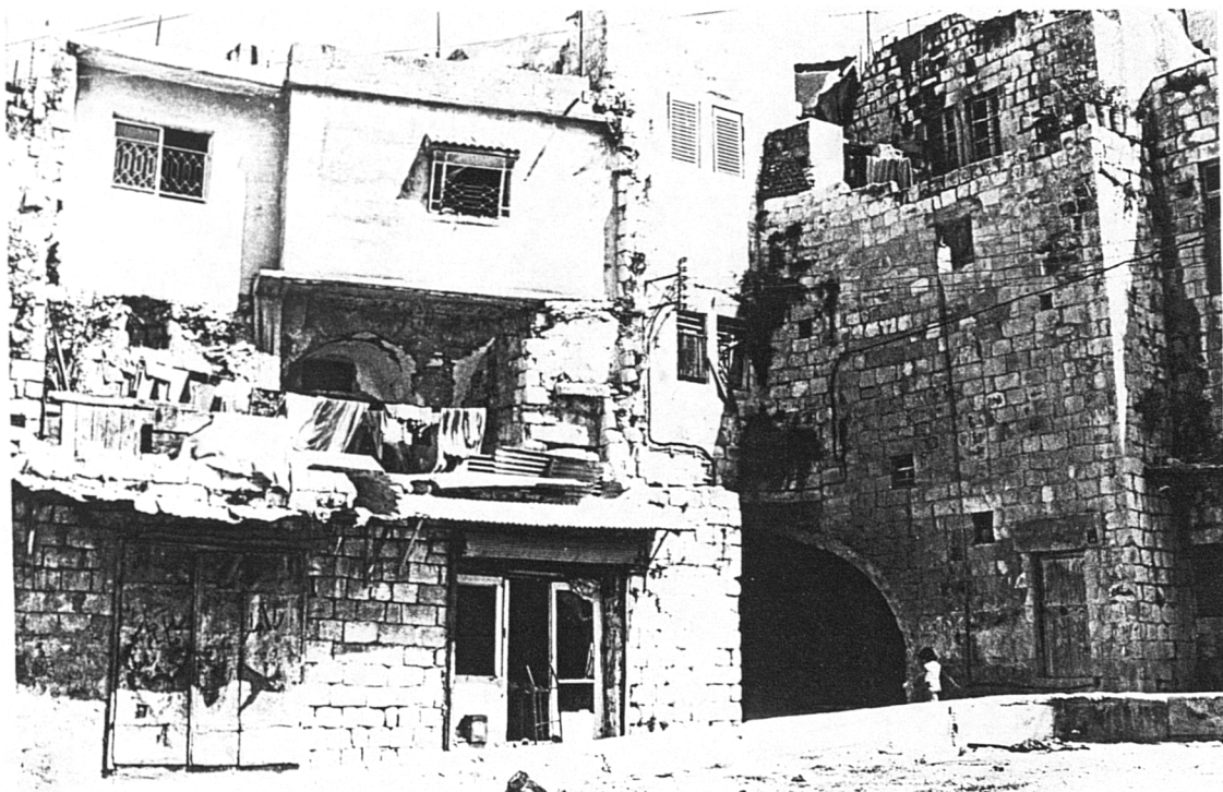
Fig. 7.17: Concrete and Concrete Blocks have become Main Building Materials in Old Nablus Source: The Author
