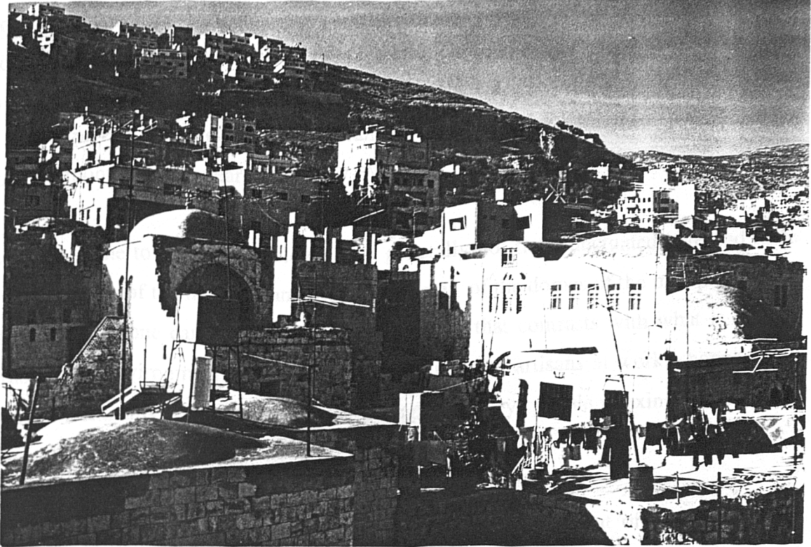
Fig. 7.4: Stone Dome Roofs are a very Characteristic expression of the Houses of Old Nablus. Source: Courtesy of Mr. Rami Shaksheer, Nablus 1992.
