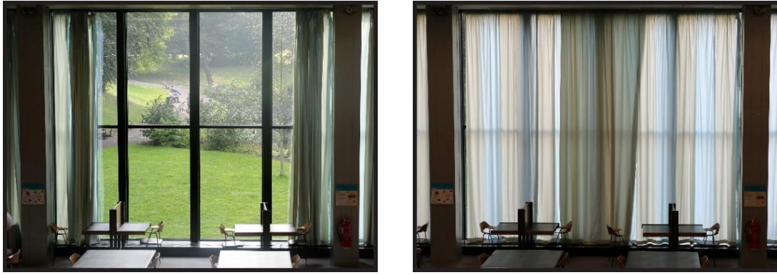
Figure 3.6. Shading position is limited to fully open (left) and fully closed (right). Automated control system does not allow the occupant to adjust shade positions, thus eliminating the uncertainty attributed to occupant control of shading devices.
