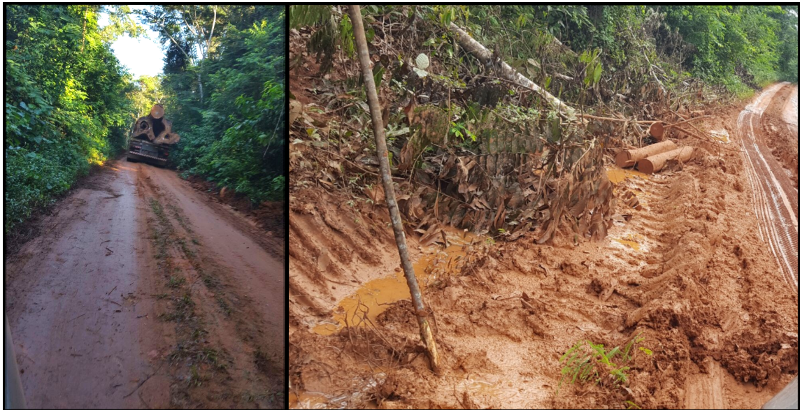
Figure B.2: Soil physical impacts observed in the field. Main road with visible soil compaction(left) and road borders with evident scarification by tractors (right)
