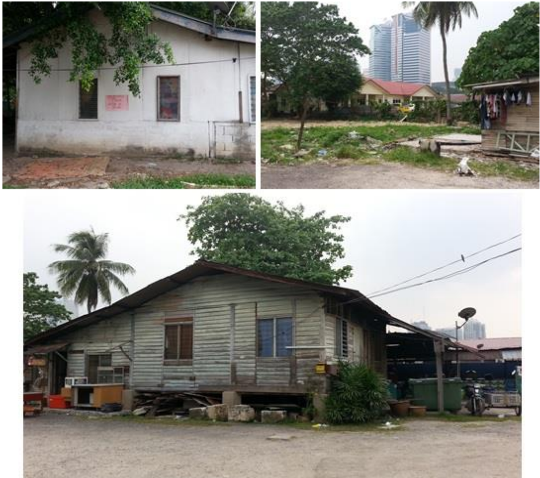
Figure 3.10: Example of a few derelict properties in Kampong Bharu
