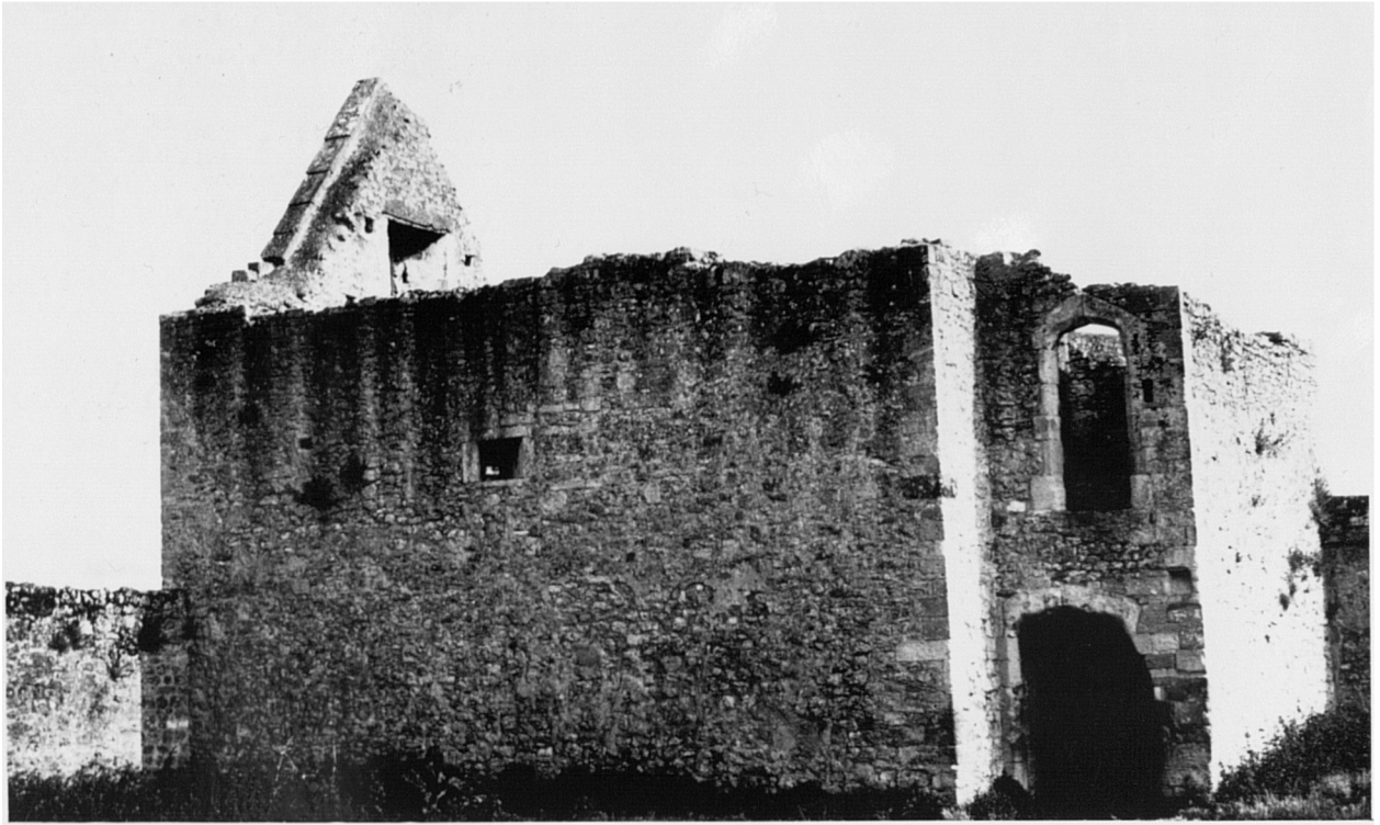
36 Godstow chapel (Oxfords): the structure was two-storeyed at its west end, and abutted a structure to the north from which a squint allowed observation.
