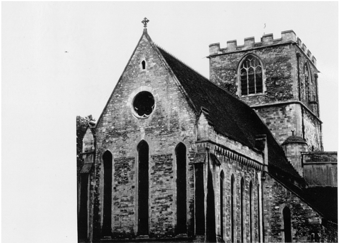
37 The church of St Radegund's, Cambridge, retains thirteenth century lancet windows.
