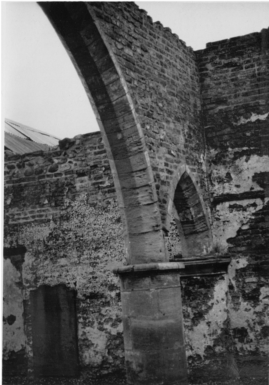
5 Nunkeeling ruined church (N Humbs). Detail of medieval nave arcade reset as chancel arch.
