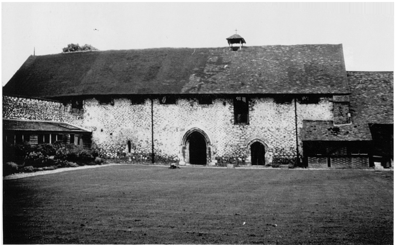
31 East range Burnham: groundfloor sacristy, chapter-house, parlour and warming house, with dormitory over.
