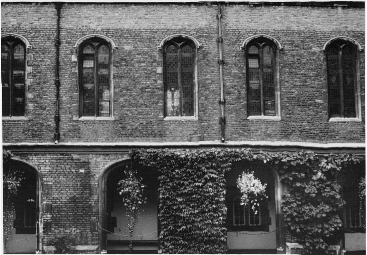
32 Two-storey refectory at St Radegund's, Cambridge (Jesus College).
