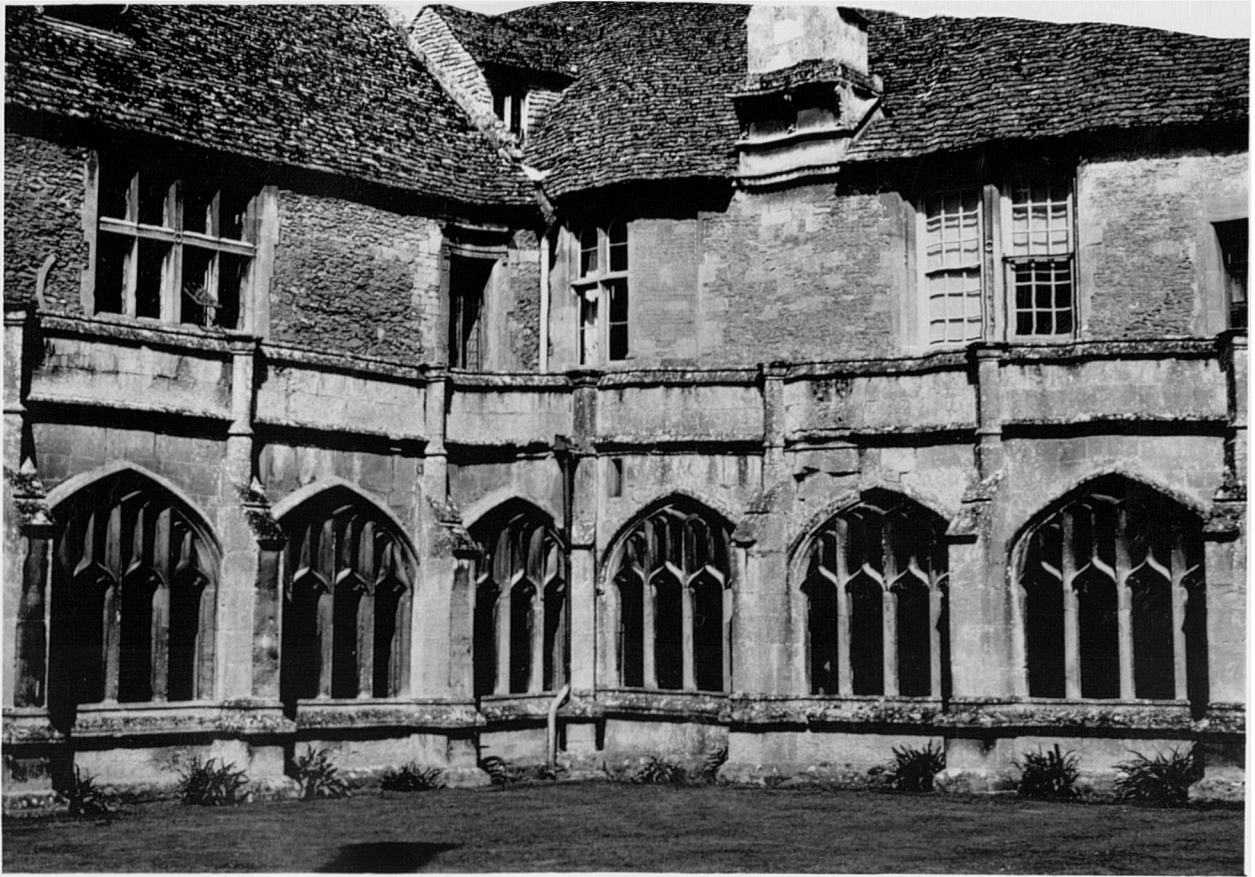
18 The free-standing cloister at Lacock (Wilts) was reused as the ground floor of the later house.
