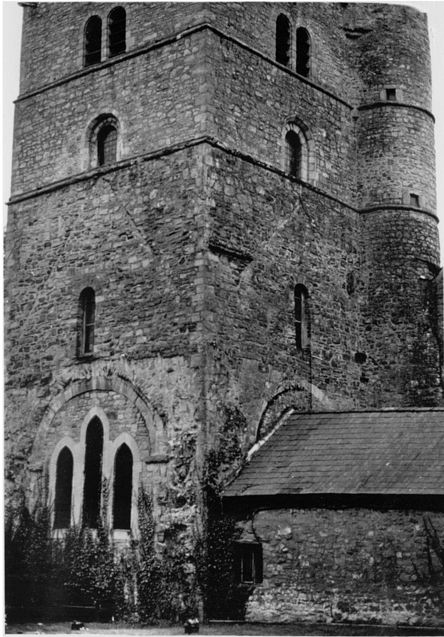
20 Usk church (Gwent). In the eastern face of the original crossing tower may be seen the roof line of the demolished chancel, and the blocked archway to the eastern arm of the nuns' church.
