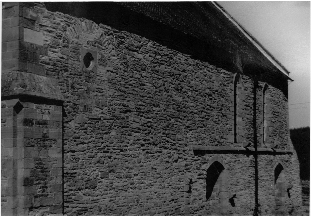
26 Blocked doorway to a western gallery from the west range at Aconbury (Herefords).
