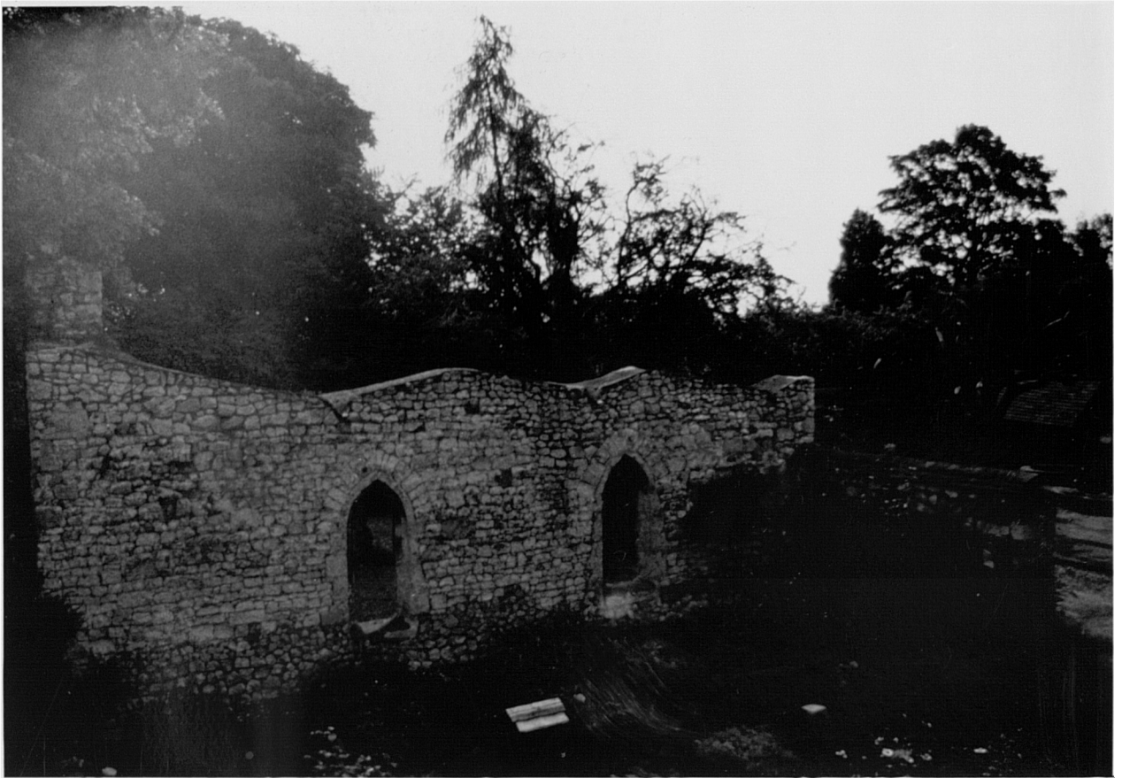
34 Burnham infirmery hall from north.
