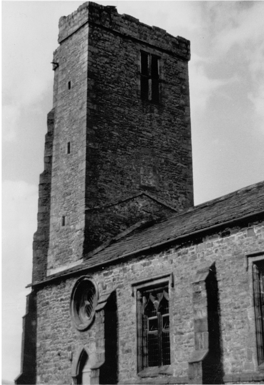
27 The rebuilt church at Marrick (N Yorks) retains evidence for a blocked doorway in the east face of the tower, and a reset trefoil (possibly for lighting a gallery) over the south door.
