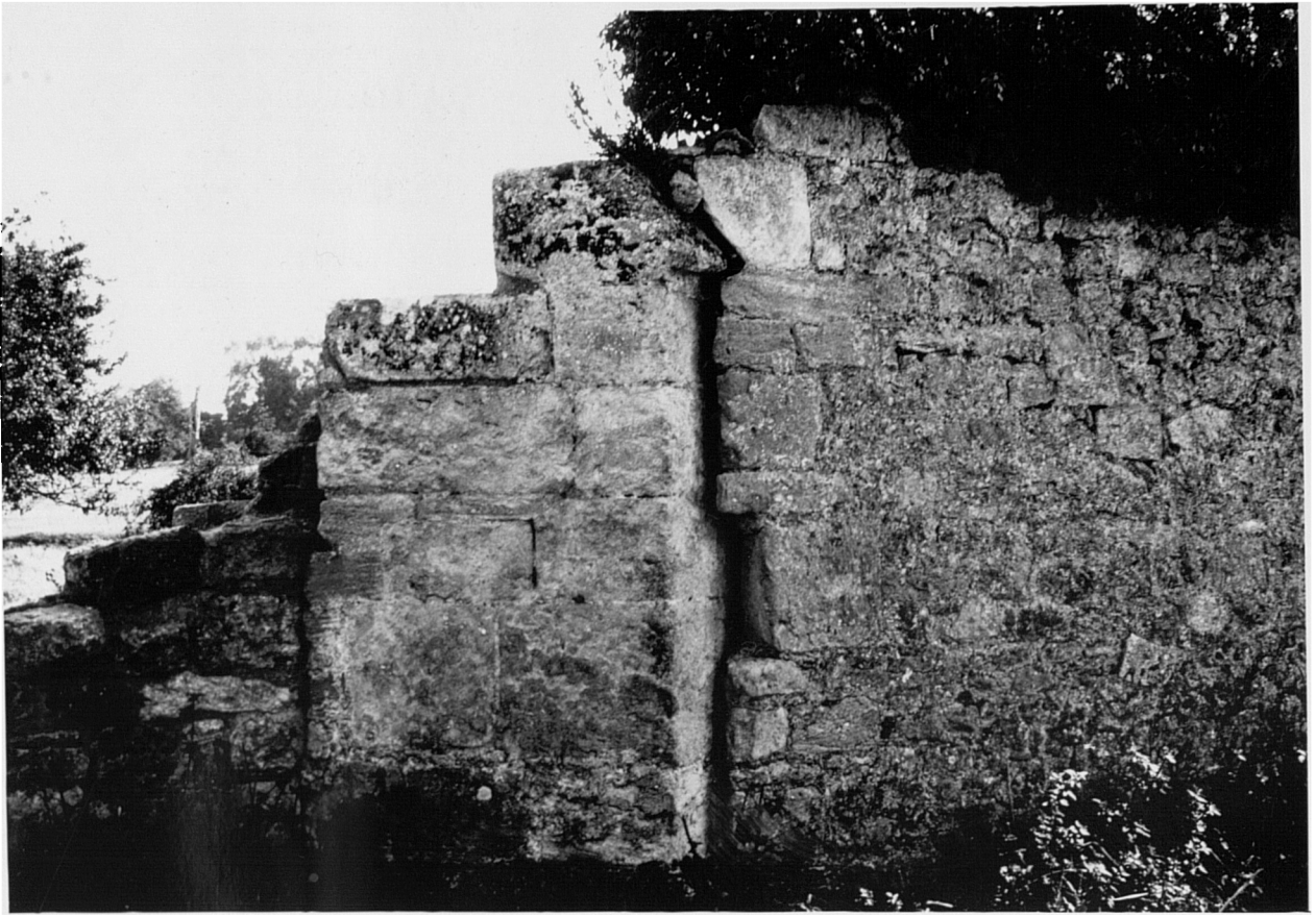
40 An extant butterss at Godstow, where the third range abutted the enclosure wall to the outer court.
