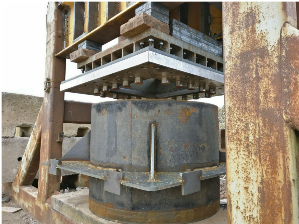
Figure 3.17: As built picture of Appliqué apparatus mounting bushings
