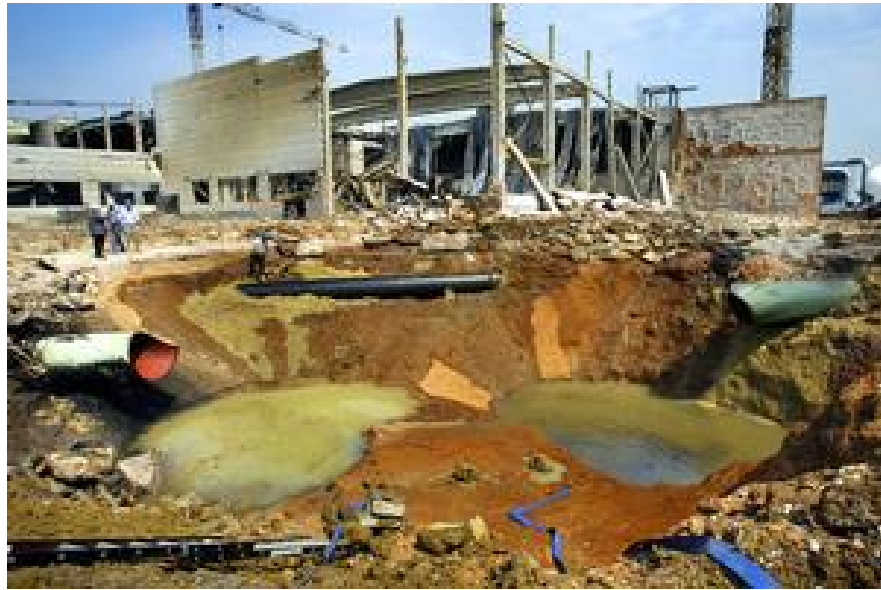
Figure 1.6: Photograph showing the crater resulting from the explosion of the gas leaking from the Ghislenghien pipeline rupture on 30th July 2014. The ends either side of the 11 m section which was ejected in the ignition are visible, as is the damage to surrounding buildings and the rubble created. Image courtesy of Associated Press.
