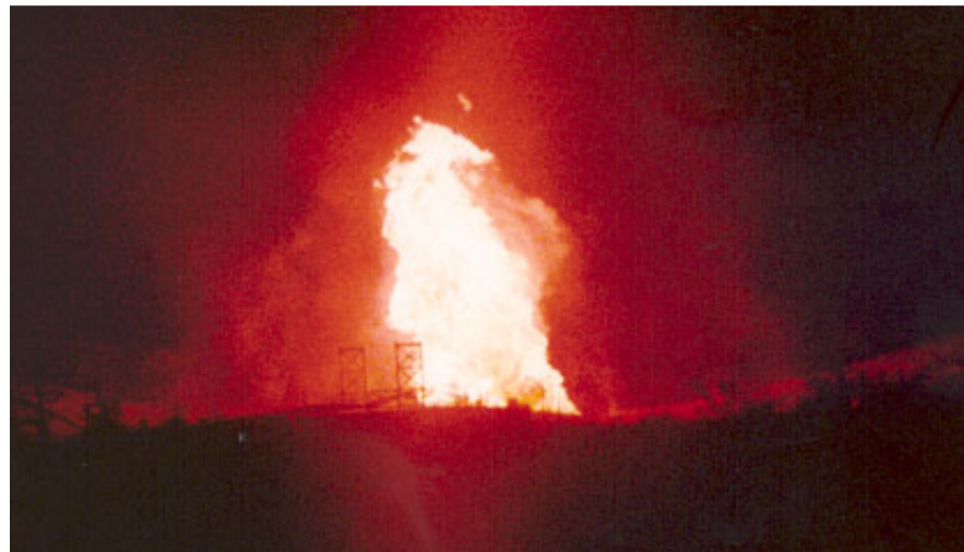
Figure 1.8: Photograph showing fire due to ignition of gas leaking from a pipeline rupture in Carlsbad, New Mexico on 19th August 2000. The pipeline river crossing suspension supports can be seen in the foreground. The ignition resulted in 12 fatalities and approximately $1 million in property damage. [5].
