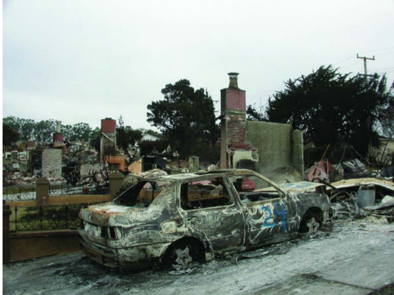
Figure 1.14: Photograph showing the destroyed houses and a burnt out car in the aftermath of ignition of gas leaking from a pipeline rupture in a residential area of San Bruno, California on 7th September 2010 [6].
