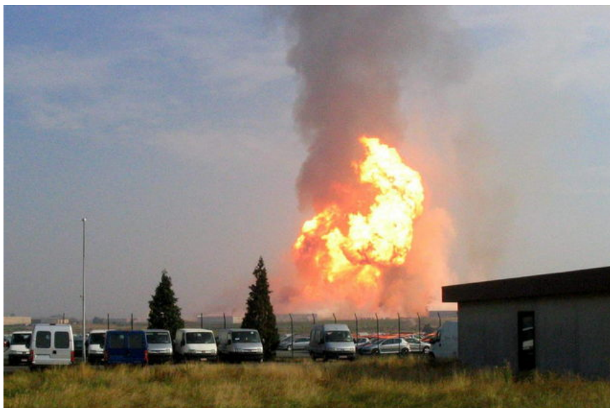
Figure 1.5: Photograph showing the approximately 150 m high flare resulting from the ignition of the gas leaking from the Ghislenghien pipeline rupture at approximately 9 am on 30th July 2014. The incident resulted in 24 fatalities, 132 serious injuries and significant property damage in the vicinity. Image courtesy of Belga Image.
