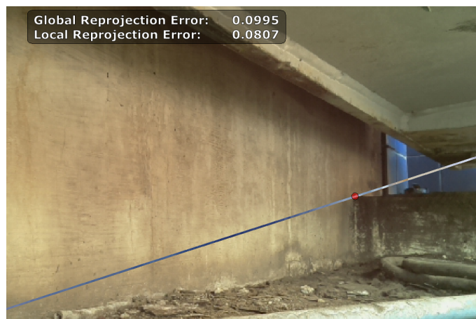
(iii): Selection of control points for scaling
