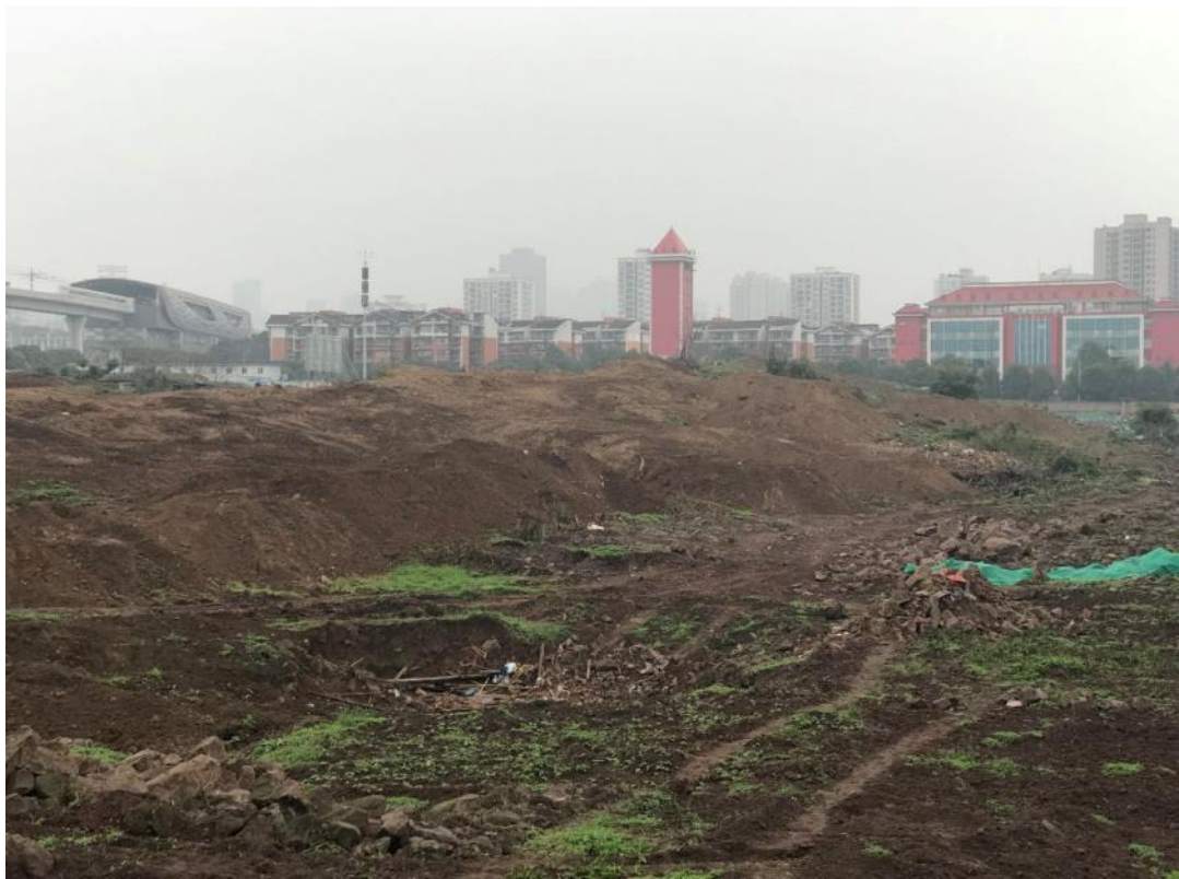
Figure 50: The kongdi being prepared for construction in February 2018. Source: WeChat.
