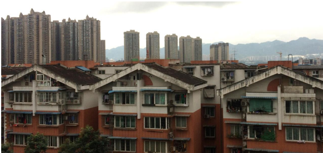
Figure 35a & 35b: Two perspectives on illegal constructions on top storeys of resettlement housing. Source: author.
