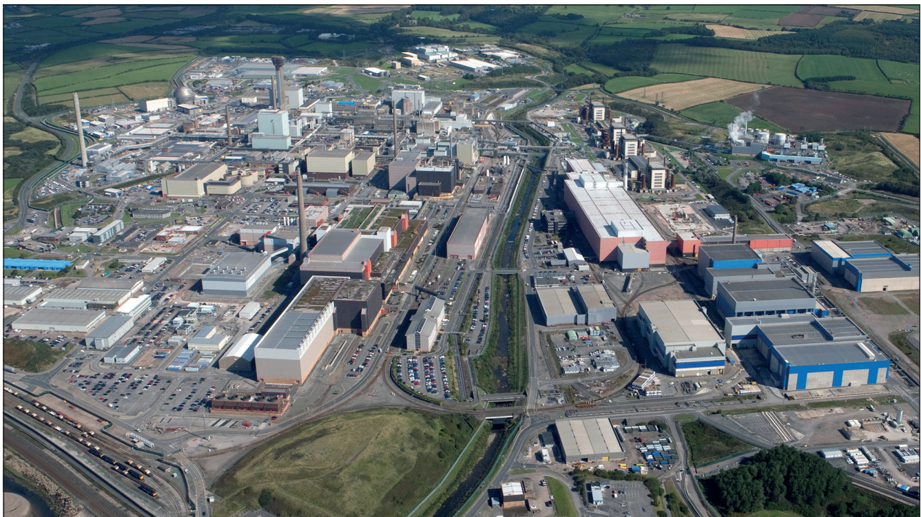
Figure 3. Decommissioning costs at Sellafield are intertwined with fuel-reprocessing costs, making analysis complex (courtesy Sellafield)
