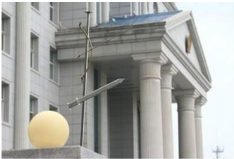
Figure 77. Despite the central government’s tight control, feng shui was carried out on the roof of a local court building in Changchun, Jilin province, aiming to spare the court from being interrogated by the procuratorate. (Source: People’s Daily Online , < http://politics.people.com.cn/GB/1025/13216723.html > [Accessed on 09 May 2017].)
