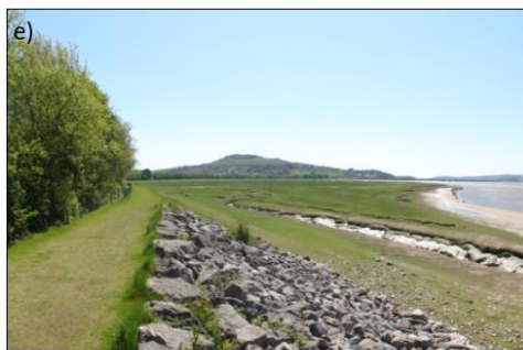
Earth and rock embankment to reduce erosion and flooding
