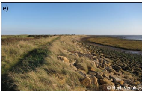
Earth and rock embankment to reduce erosion and flooding
