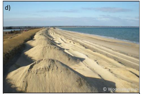
Beach "nourishment" through redistribution of sand, to replace lost beach material and help reduce erosion
