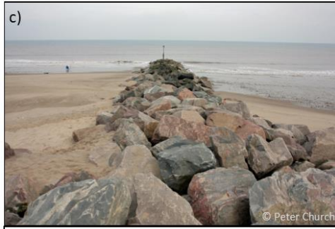
Rock groynes to encourage build-up of beach material and absorb wave energy
