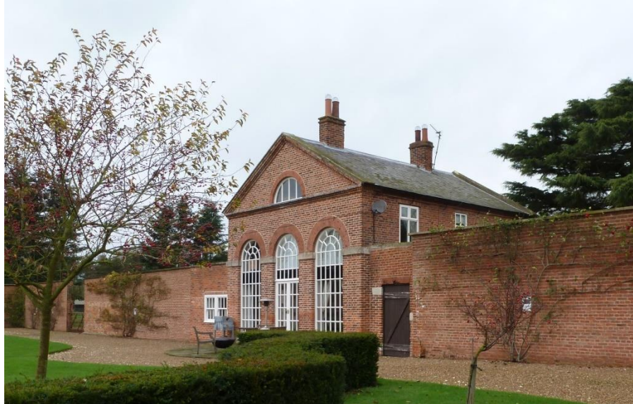
FIGURE 12: THE SURVIVING ELEMENTS OF THE STOVE COMPLEX, NOW CONVERTED TO A FORMAL GARDEN AND LODGING. THE TWO SMALL GREENHOUSES ARE CLEARLY PRESENT, WITH THE AREA WHICH WOULD HAVE HOUSED THE STOVE IN BETWEEN (AUTHOR).
