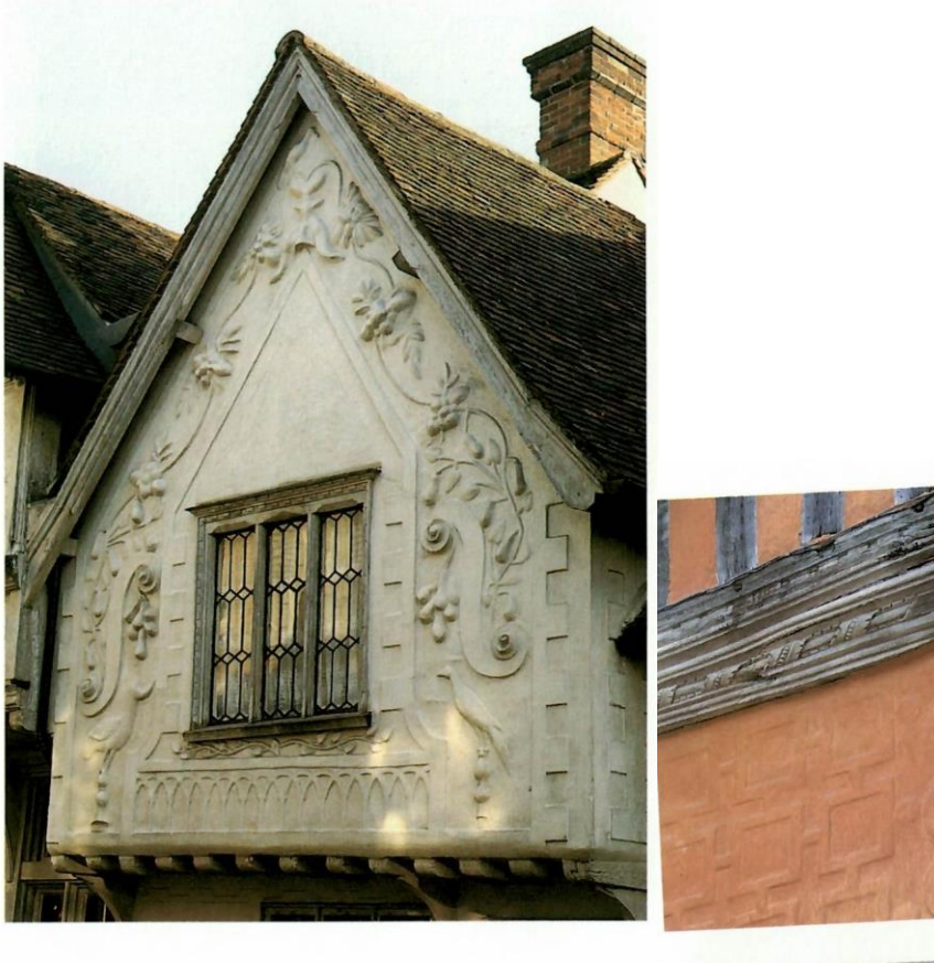
Figure 18: Houses in Saffron Walden and Lavenham showing timber-framed construction, including pargetting on the left. Source: Mowl, Elizabethan and Jacobean Style , 42-43.
