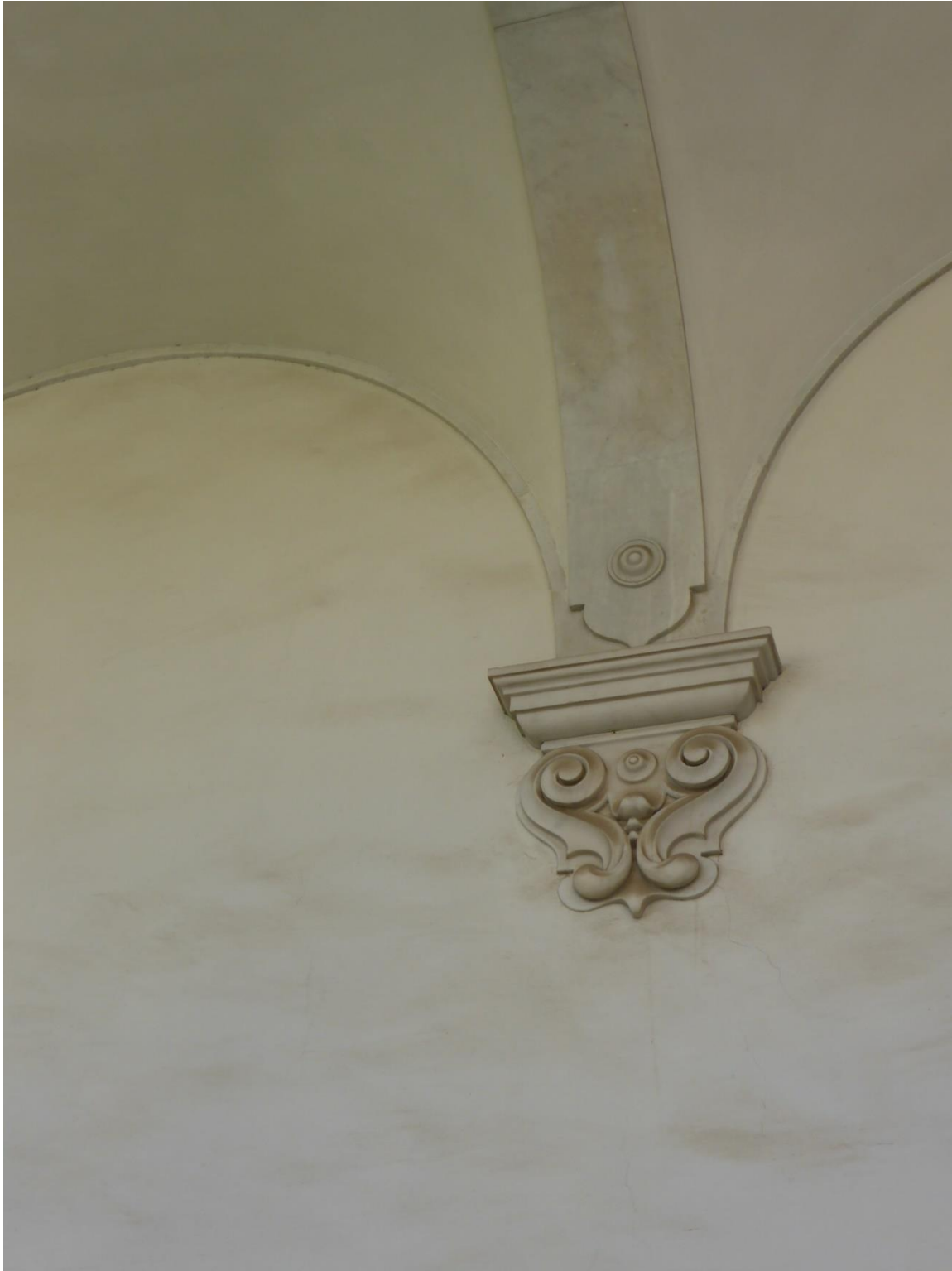
Figure 110: Detail showing the elaborate console of the responding arches of the Great Cloister walks, Certosa di San Martino. Source: author's own photograph.
