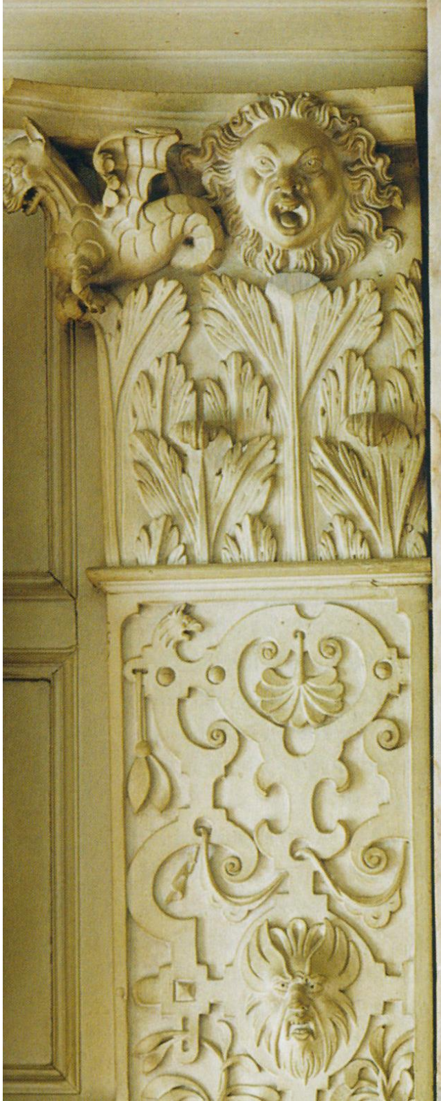
Figure 97: Detail of main pilaster order, Great Chamber wainscot, Knole, Kent. Volutes are substituted by sea creatures and the rosette by a grotesque mask/sun badge. Another mask on the shaft of the pilaster below. Detail of Figure 92.
