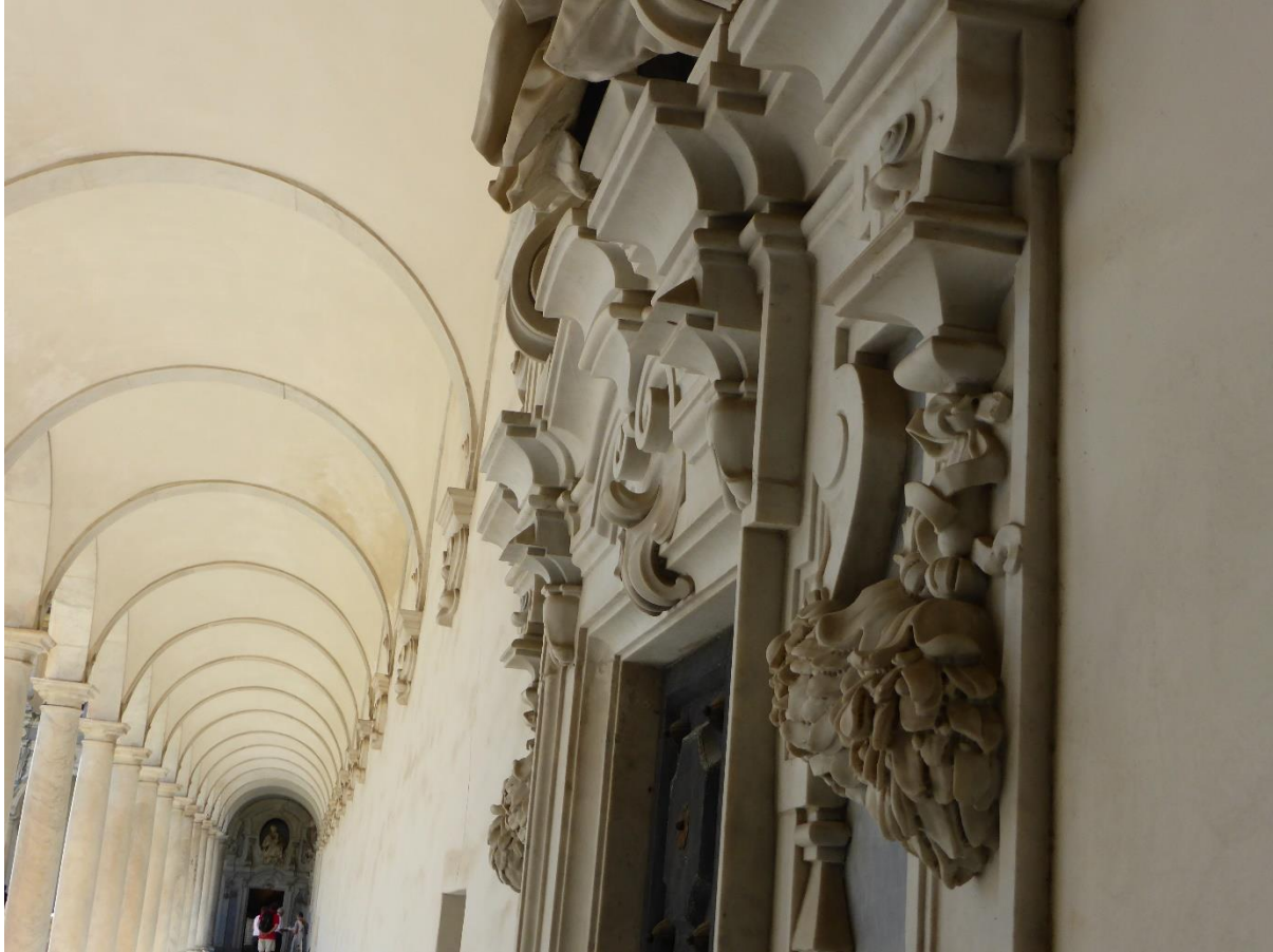
Figure 141: Profile view of door 7 (bust of Saint Januarius) in the Great Cloister of San Martino. The sharp cutting and layering of the marble fortifies and thickens the corner. Note the door with bust of Nicola Albergati in terminating the arcaded vista in the background. Source: author's own photograph.
