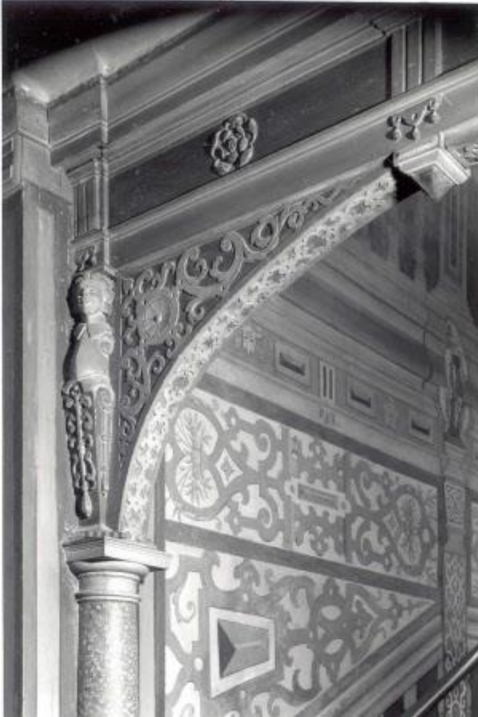
Figure 12: Painted Stair, Knole. Detail of carved decoration of the lower landing arcade. See high relief term figure, strapwork spandrel decoration and carved roses in the frieze. Source: National Trust Images.
