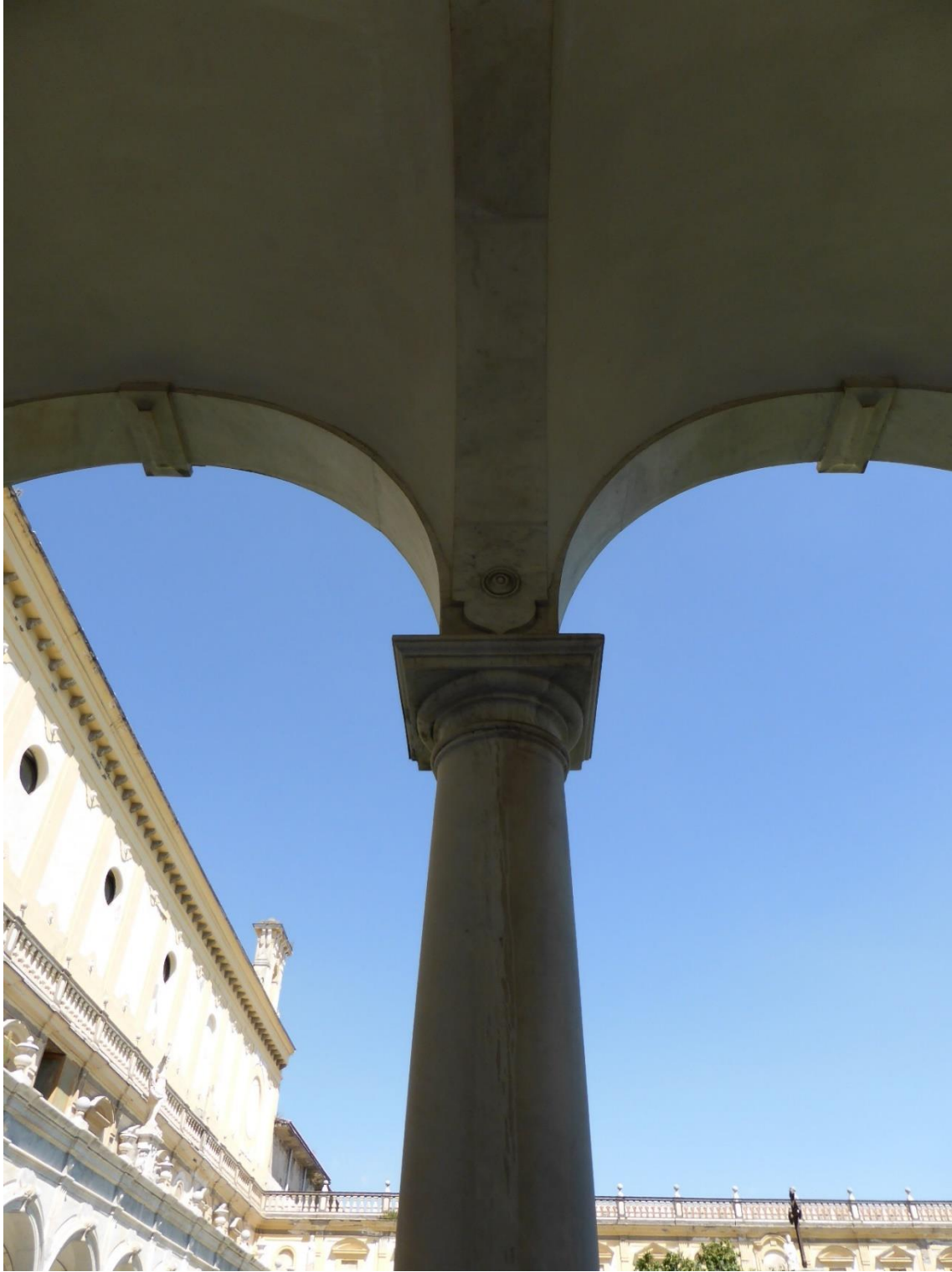
Figure 111: Detail of Cosimo Fanzago's 'ornaments' of the Great Cloister, Certosa di San Martino, showing the flourish finishing the rib of the responding arches above the capital of the order. Source: author's own photograph.
