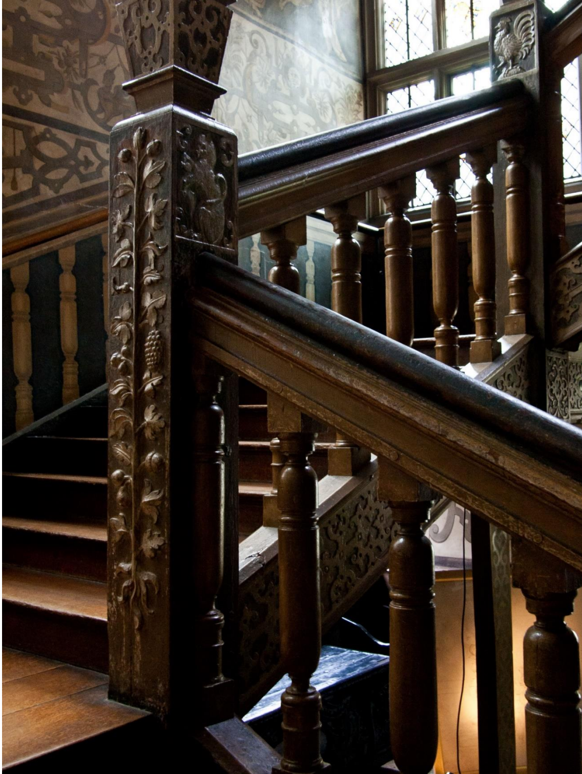
Figure 9: Painted Stair, Knole. Detail of newel post, including high-relief vegetal carving, and low-relief strapwork carving of the upper portion and stair rail.
