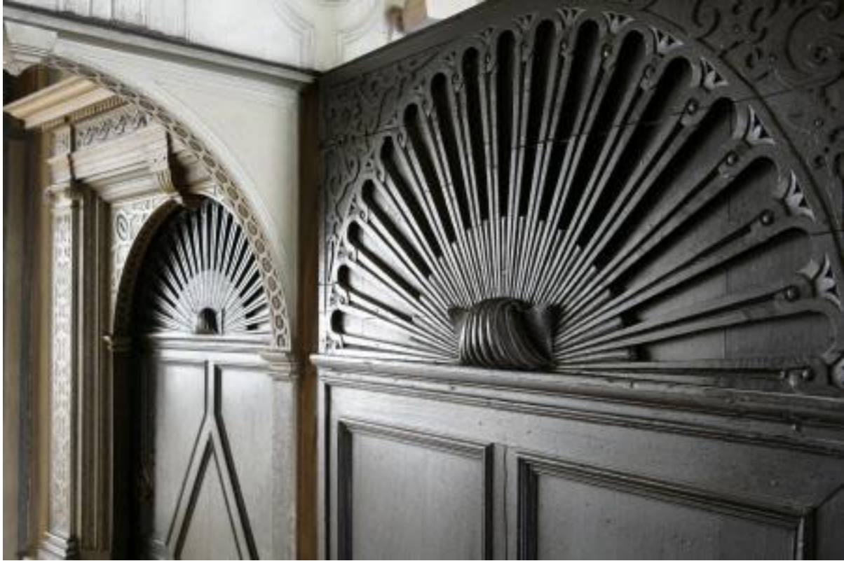
Figure 11: Door from Great Chamber, Knole House, to the Painted Stair. See details of strapwork carving in the doorframe. Source: National Trust Images.
