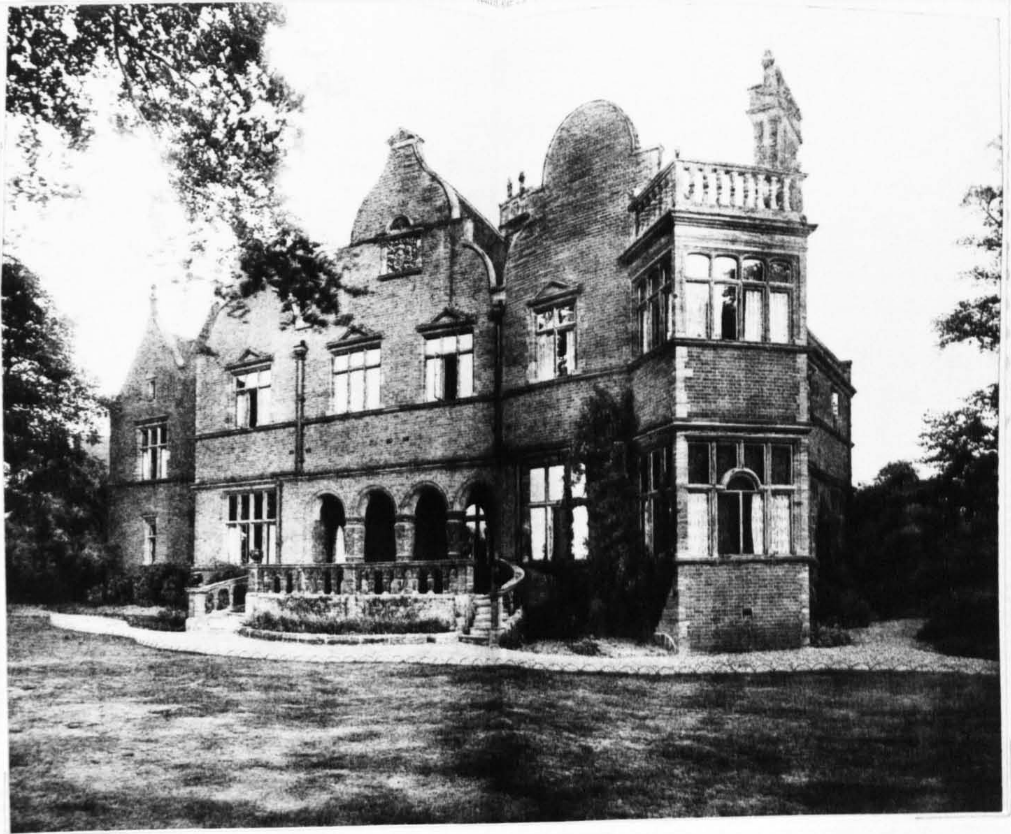
196 George and Peto, Tudor House, Hampstead, London NW3, C.1882, Exterior (A 23 March 1894); Cat.no.54
