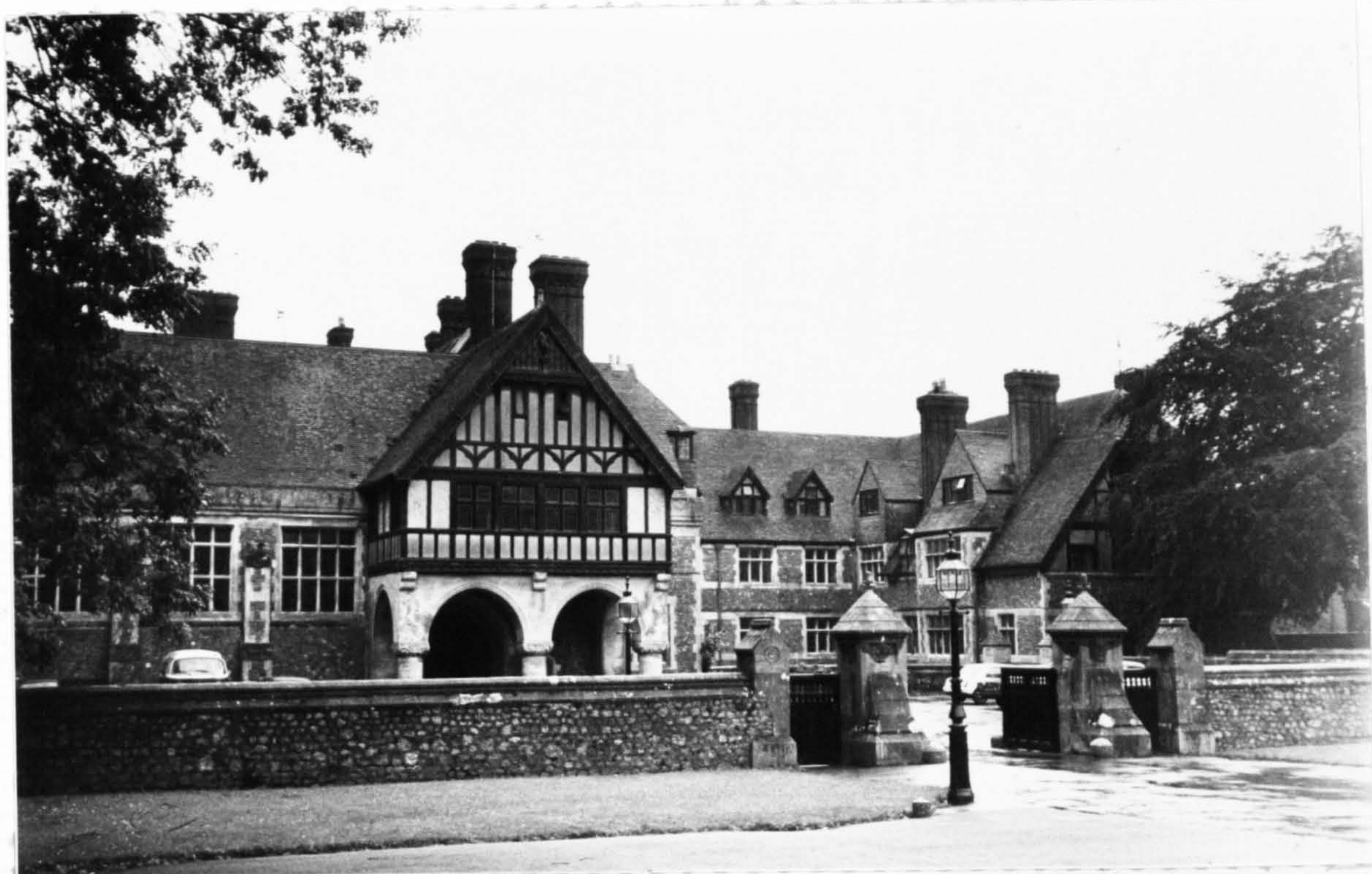
15 George and Vaughan, Rousdon, Devon, 1874-83, North Entrance Front; Cat.no.17D
