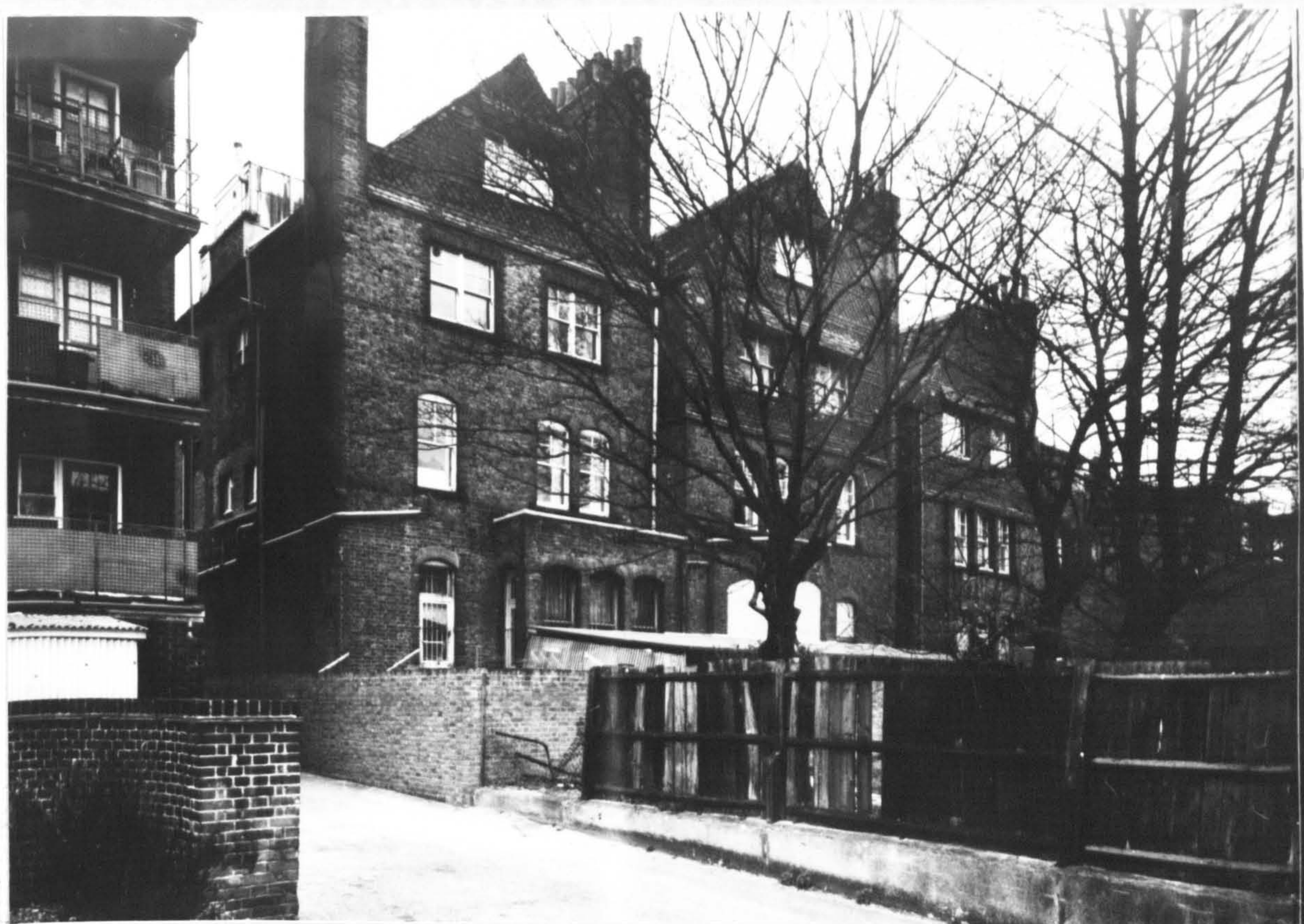
62 George and Peto, Hambly Houses, 412, 414 & 416 Streatham High Road, Streatham, London SW16, 1877, Rear Elevations; Cat.no.28
