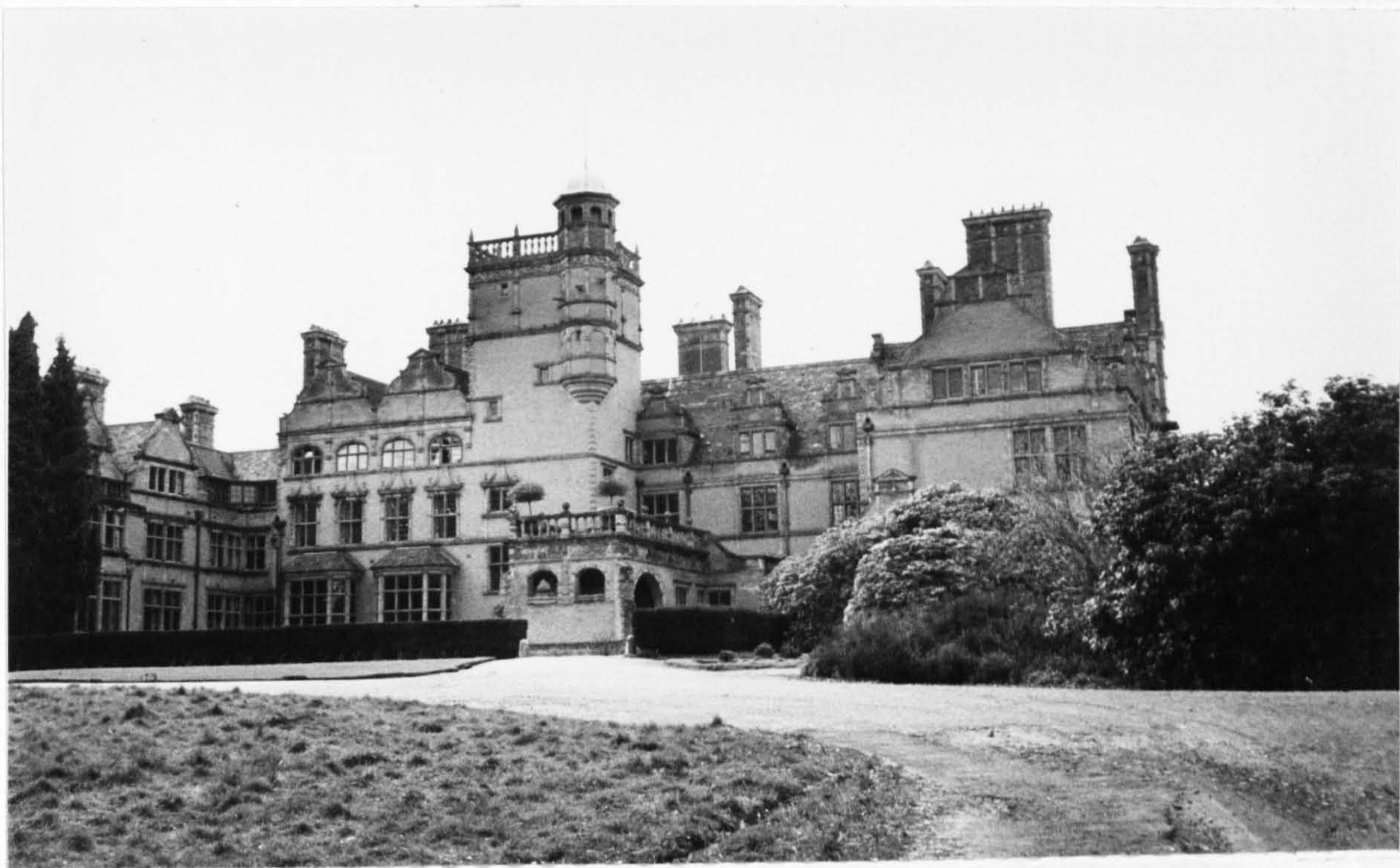
183 George and Peto, Buchan Hill, near Crawley, Sussex, 1882-83, Entrance Front; Cat.no.50
