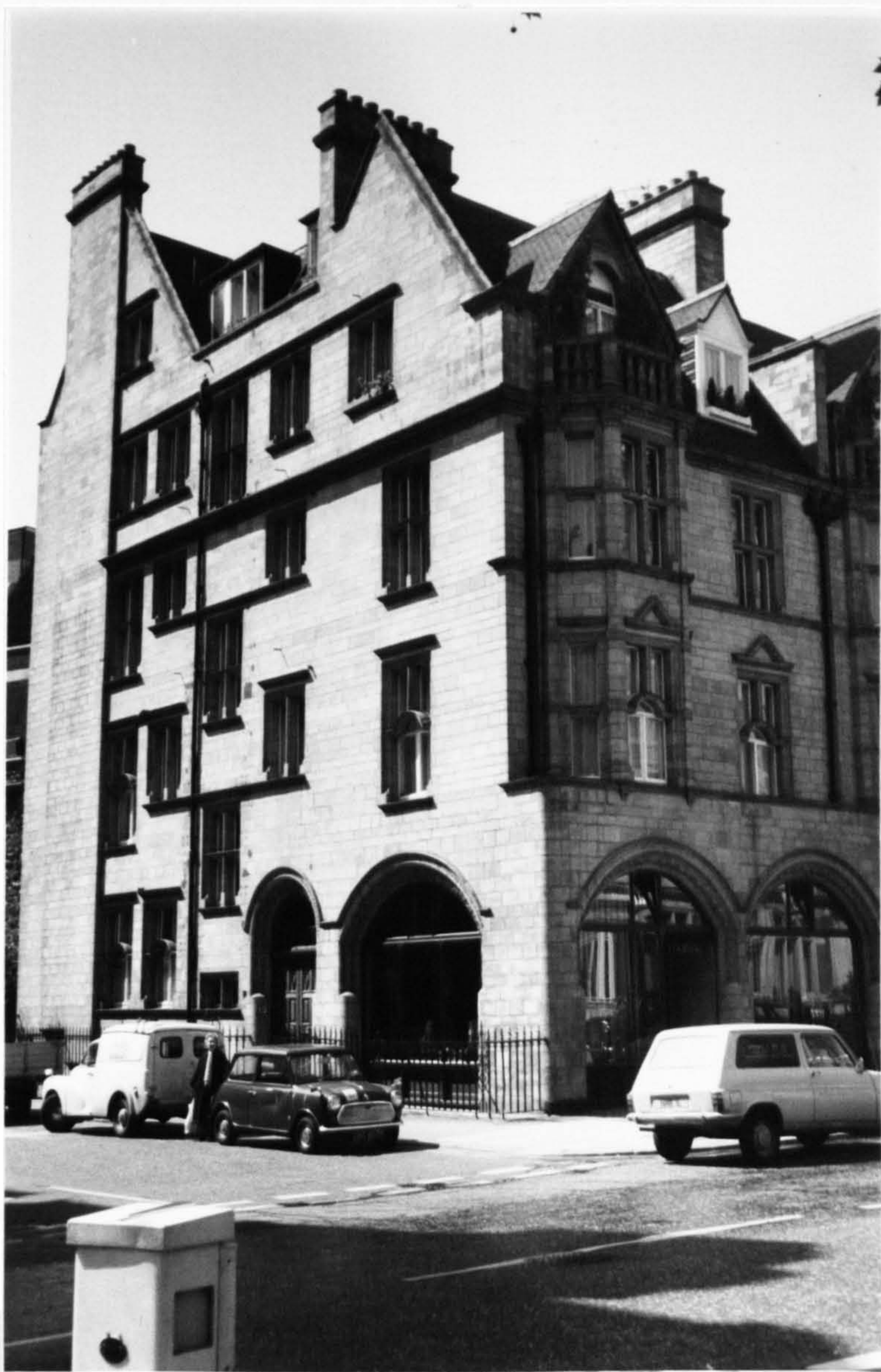
151 George and Peto, 112-113 Mount Street, London W1, 1891-92, Street Frontage; Cat.no.75C
