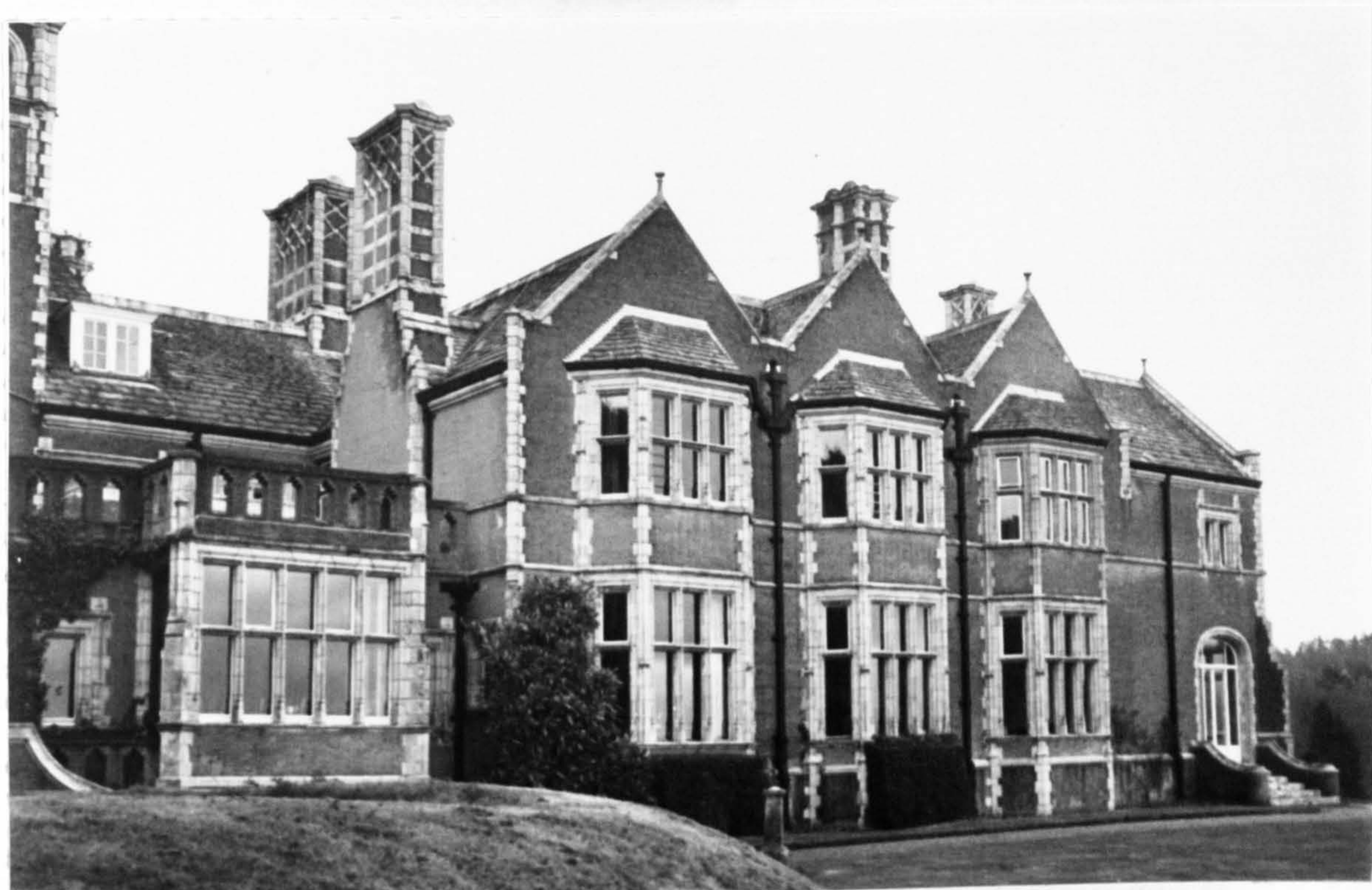
164 George and Peto, Woolpits, Ewhurst, Surrey, 1885-88, South Front, from the South-west; Cat.no.77
