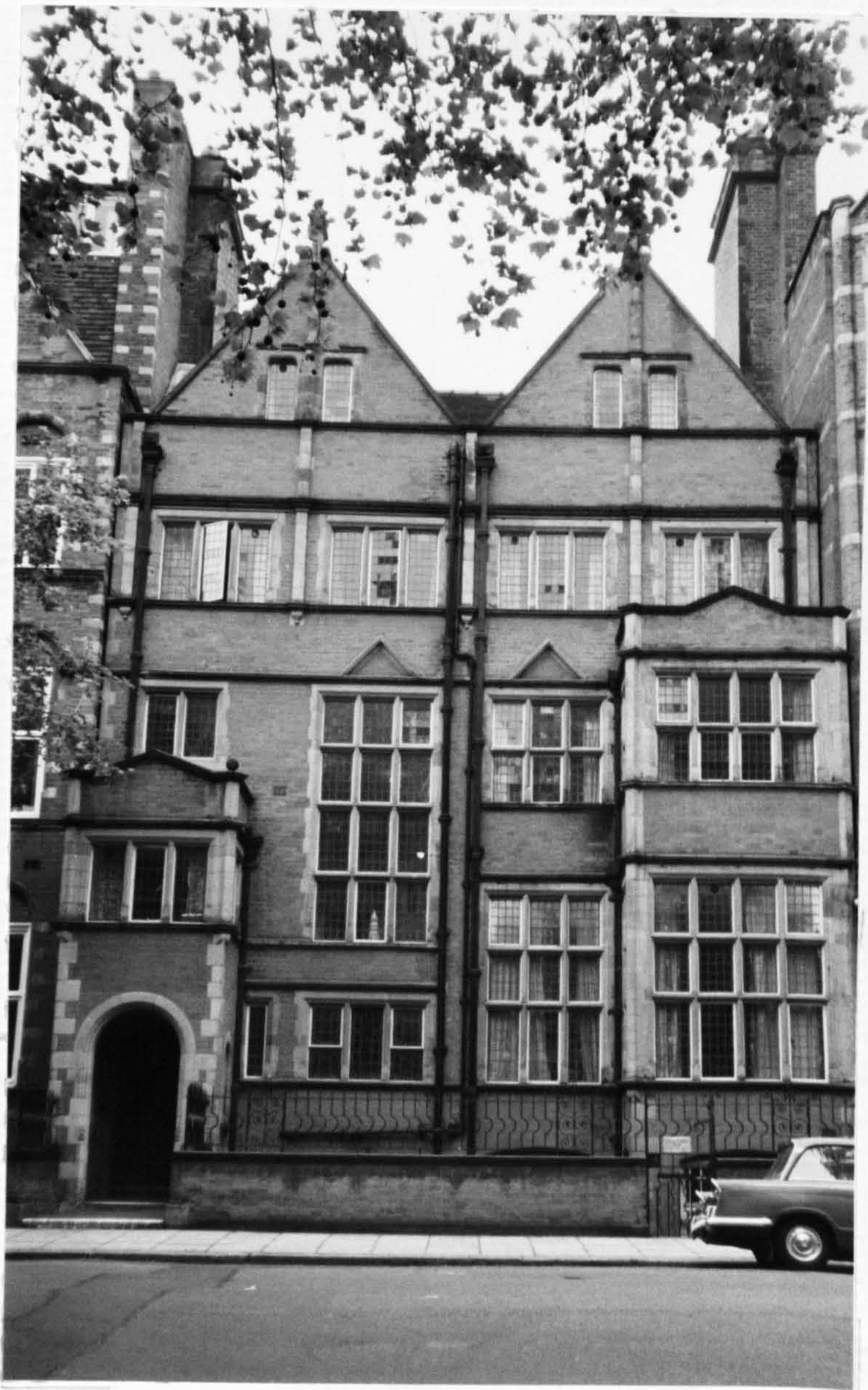
142 George and Peto, 17 Collingham Gardens, London SW5, 1887-88; Cat.no.61M
