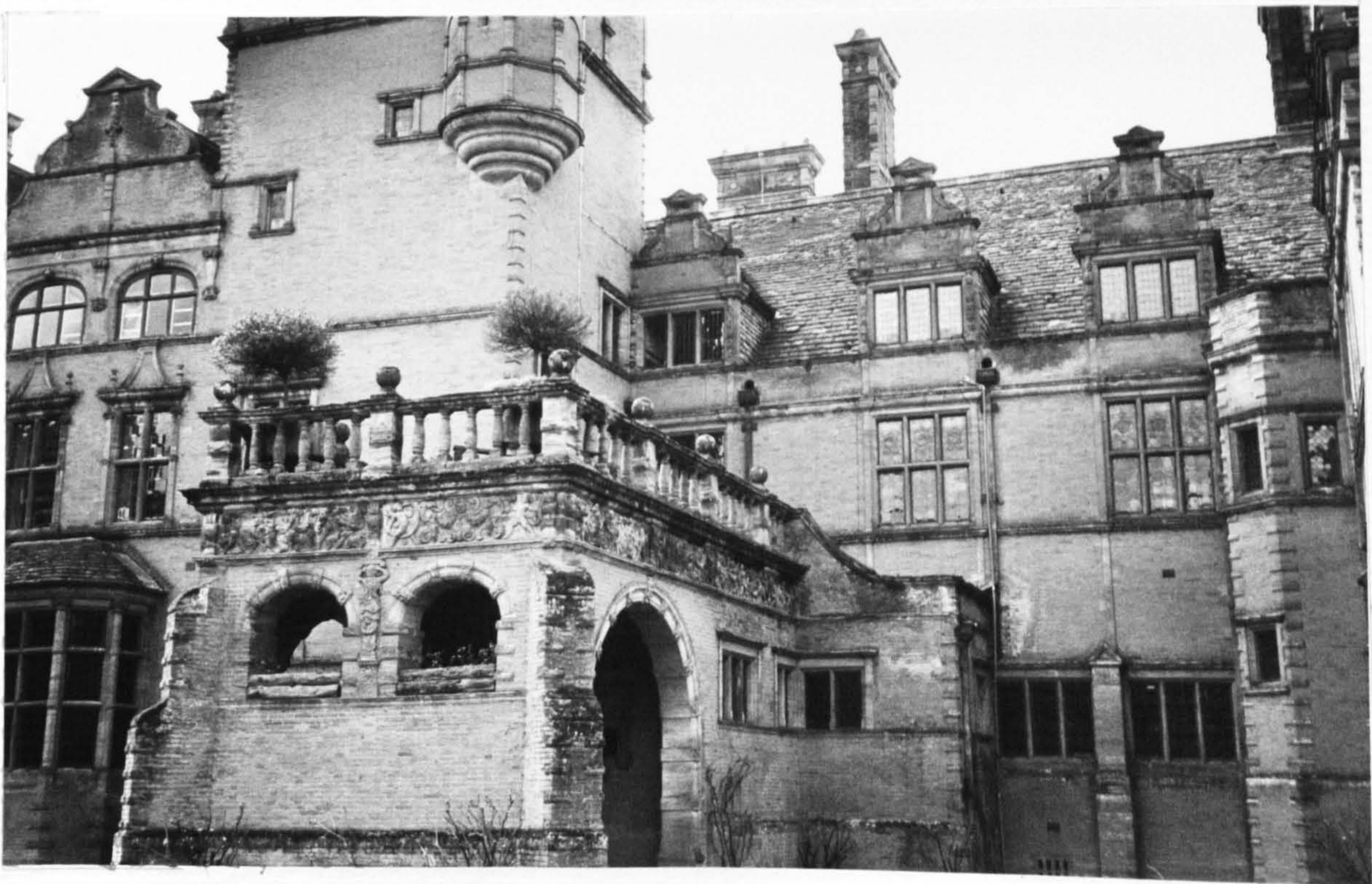
182 George and Peto, Buchan Hill, near Crawley, Sussex, 1882-83, Detail of Entrance Front; Cat.no.50
