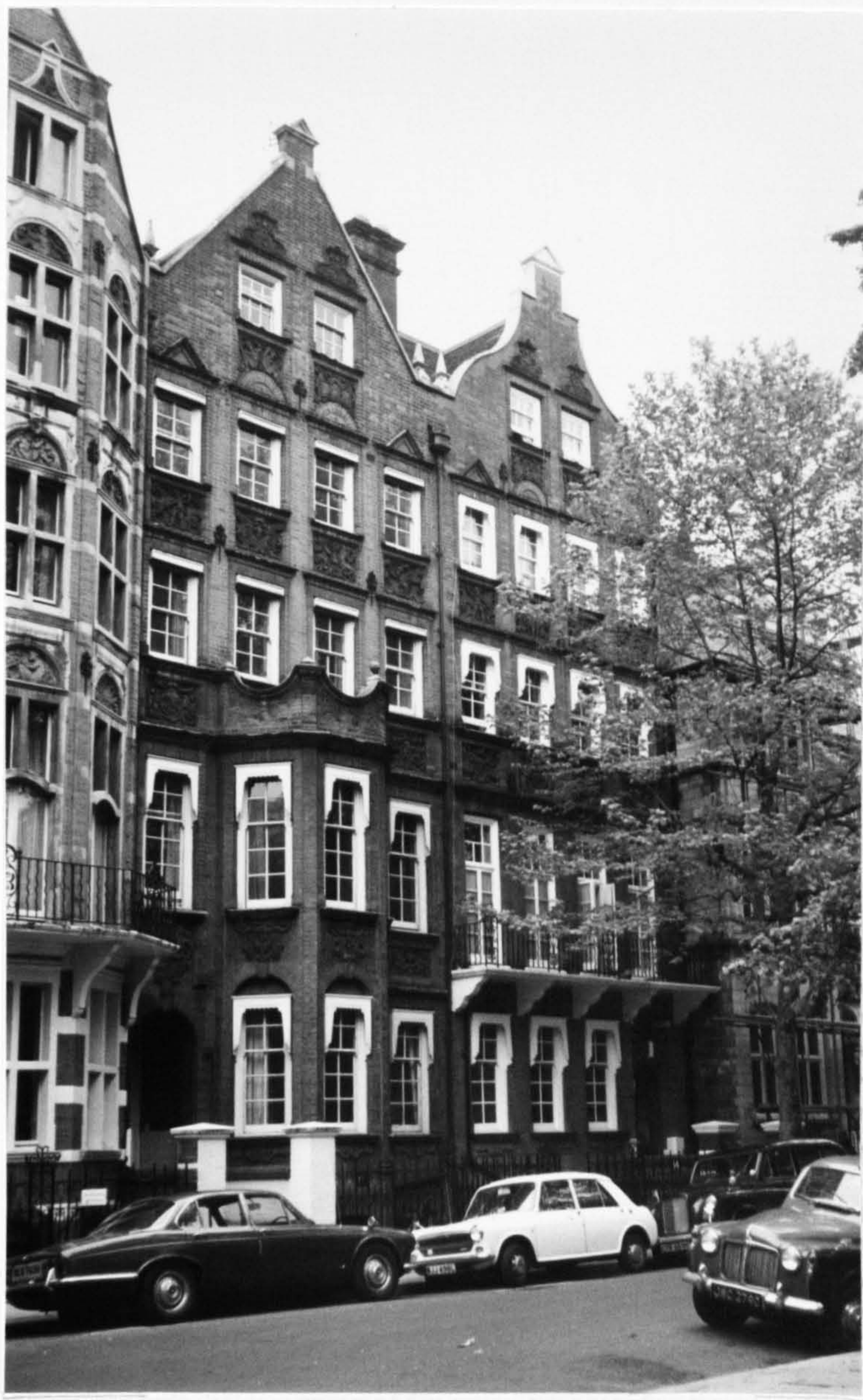
140 George and Peto, 14 & 15 Collingham Gardens, London SW5, 1886-87, Street Fronts; Cat.no.61L
