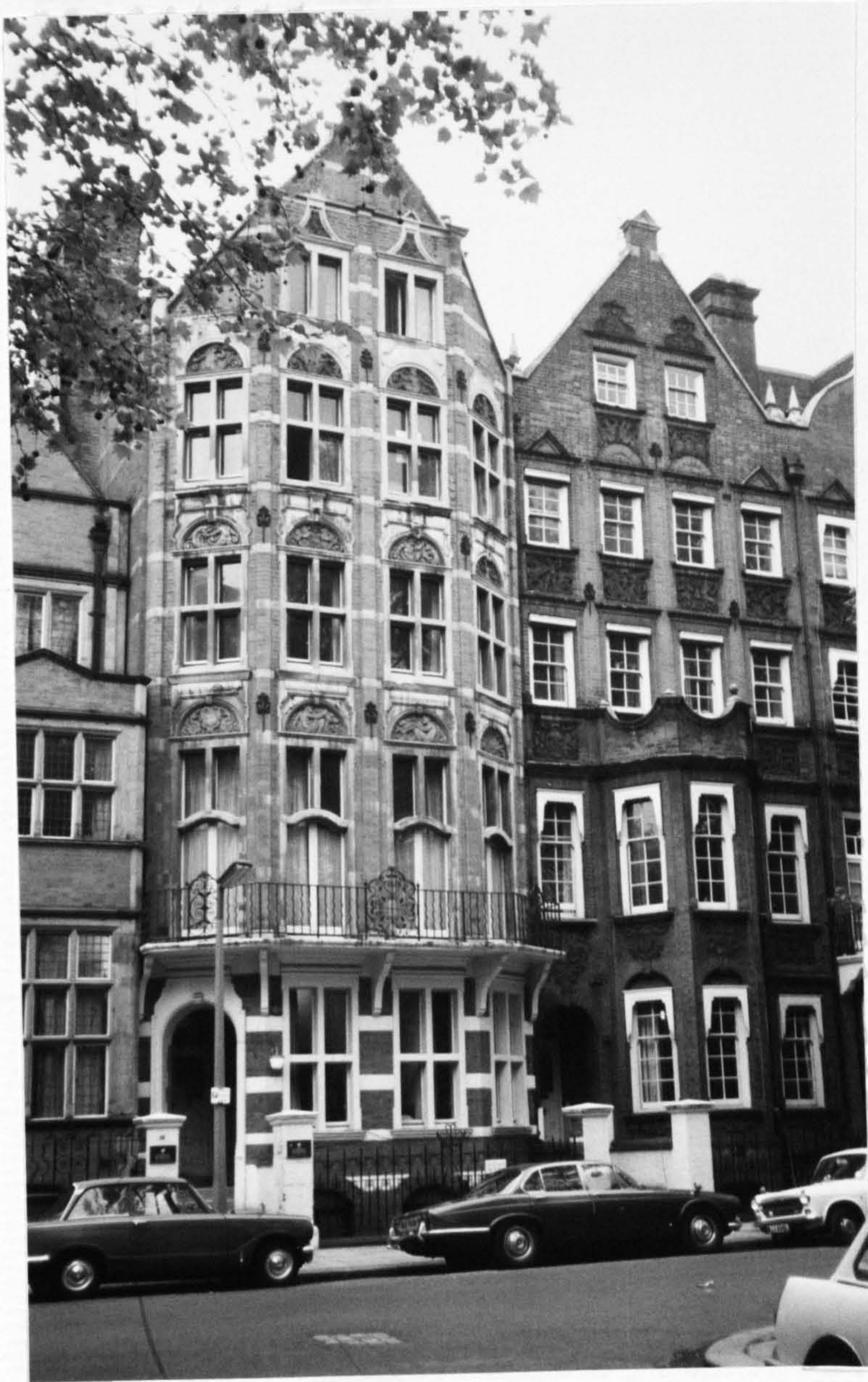
141 George and Peto, 15 & 16 Collingham Gardens, London SW5, 1886-87, Street Fronts; Cat.no.61L
