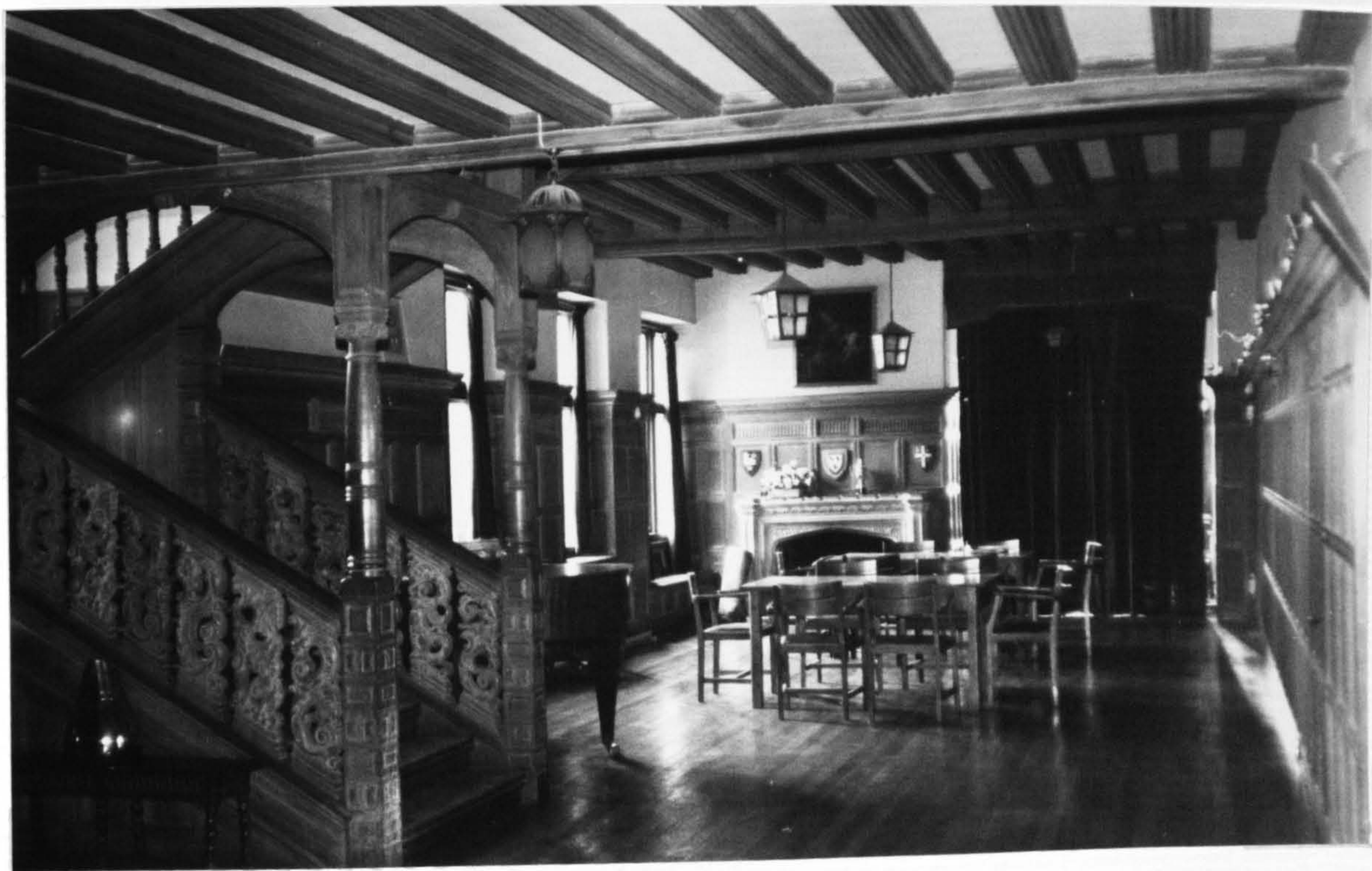
167 George and Peto, Woolpits, Ewhurst, Surrey, 1885-88, Hall and Staircase; Cat.no.77
