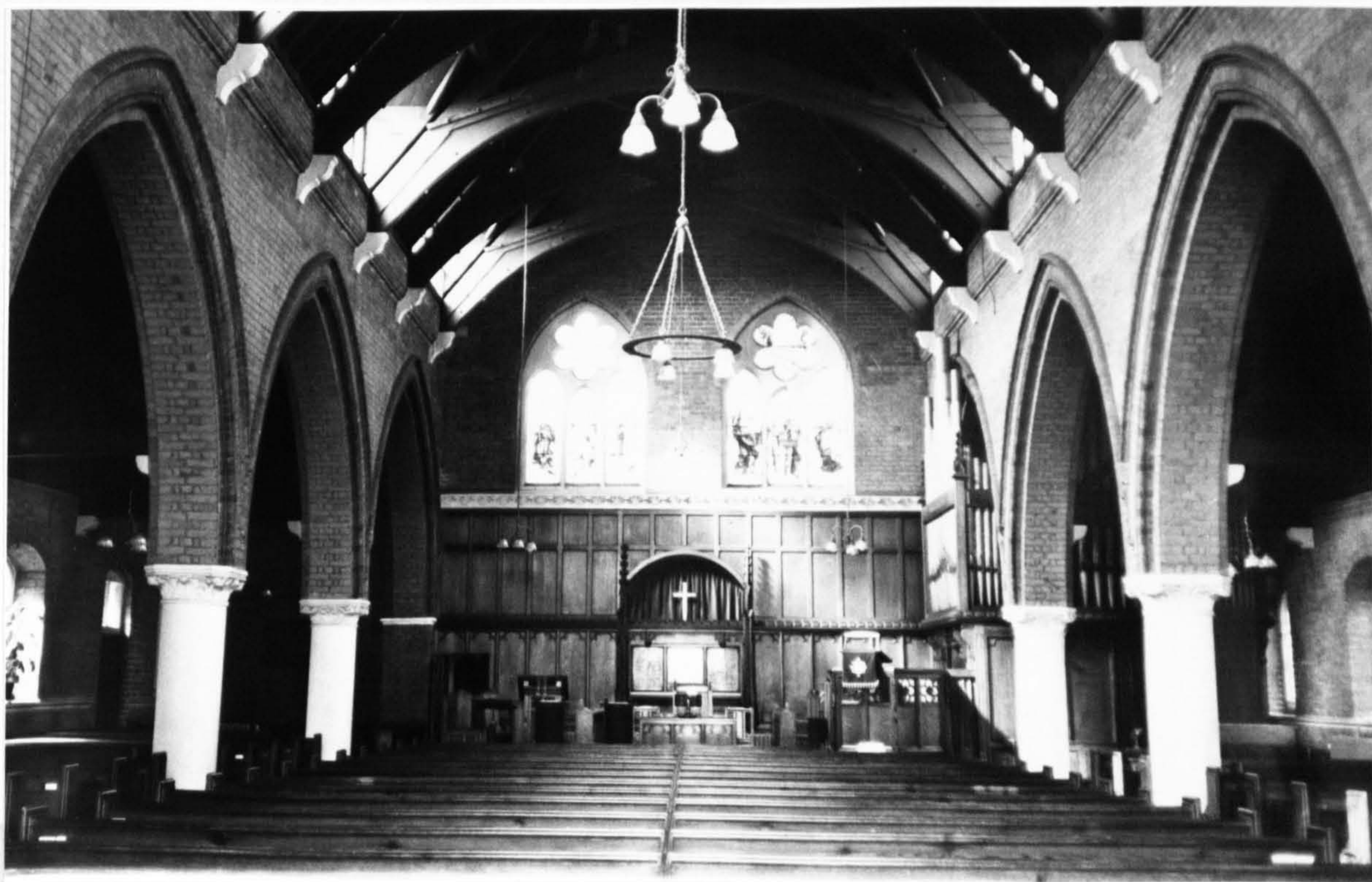
60 George and Peto, Trinity Presbyterian Church, Angles Road, Streatham, London SW16, Interior, 1876-77; Cat.no.25
