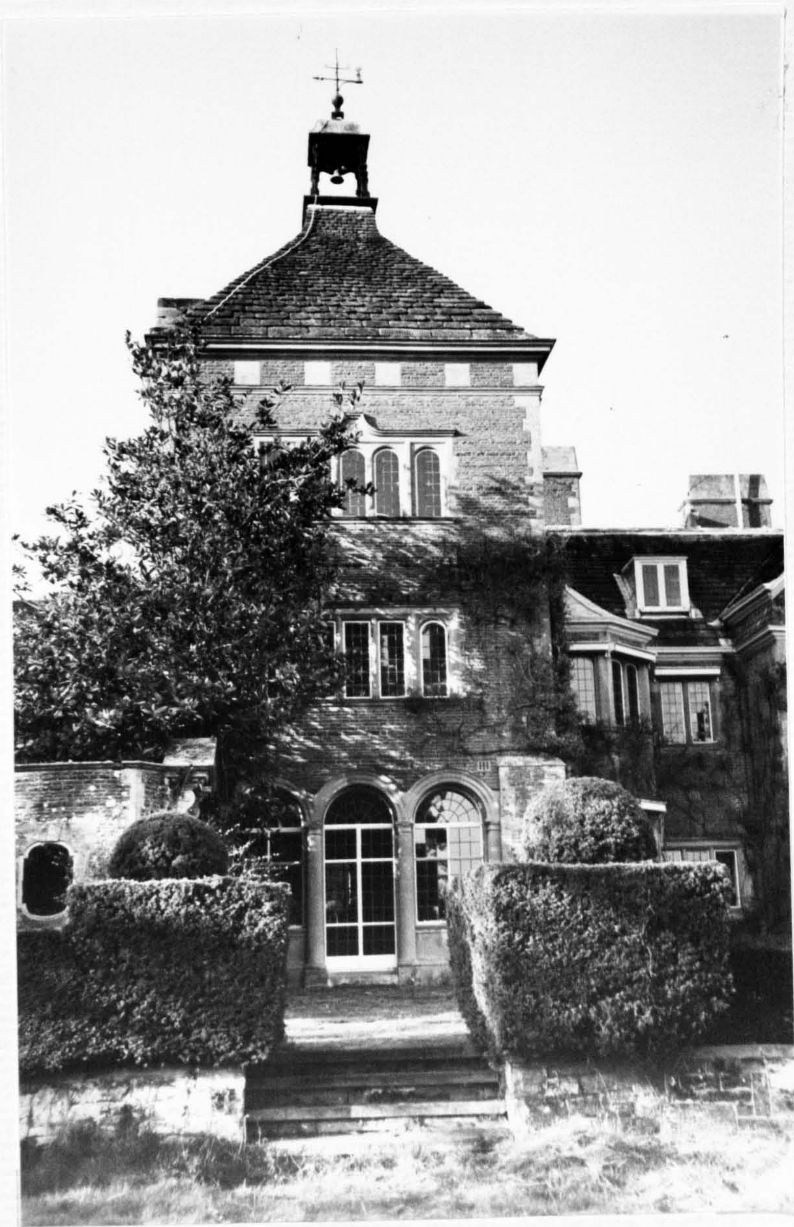
209 George and Peto, Sedgwick Park, Horsham, Sussex, 1886, 1903-04, Tower, 1903, Garden Front; Cat.no.83
