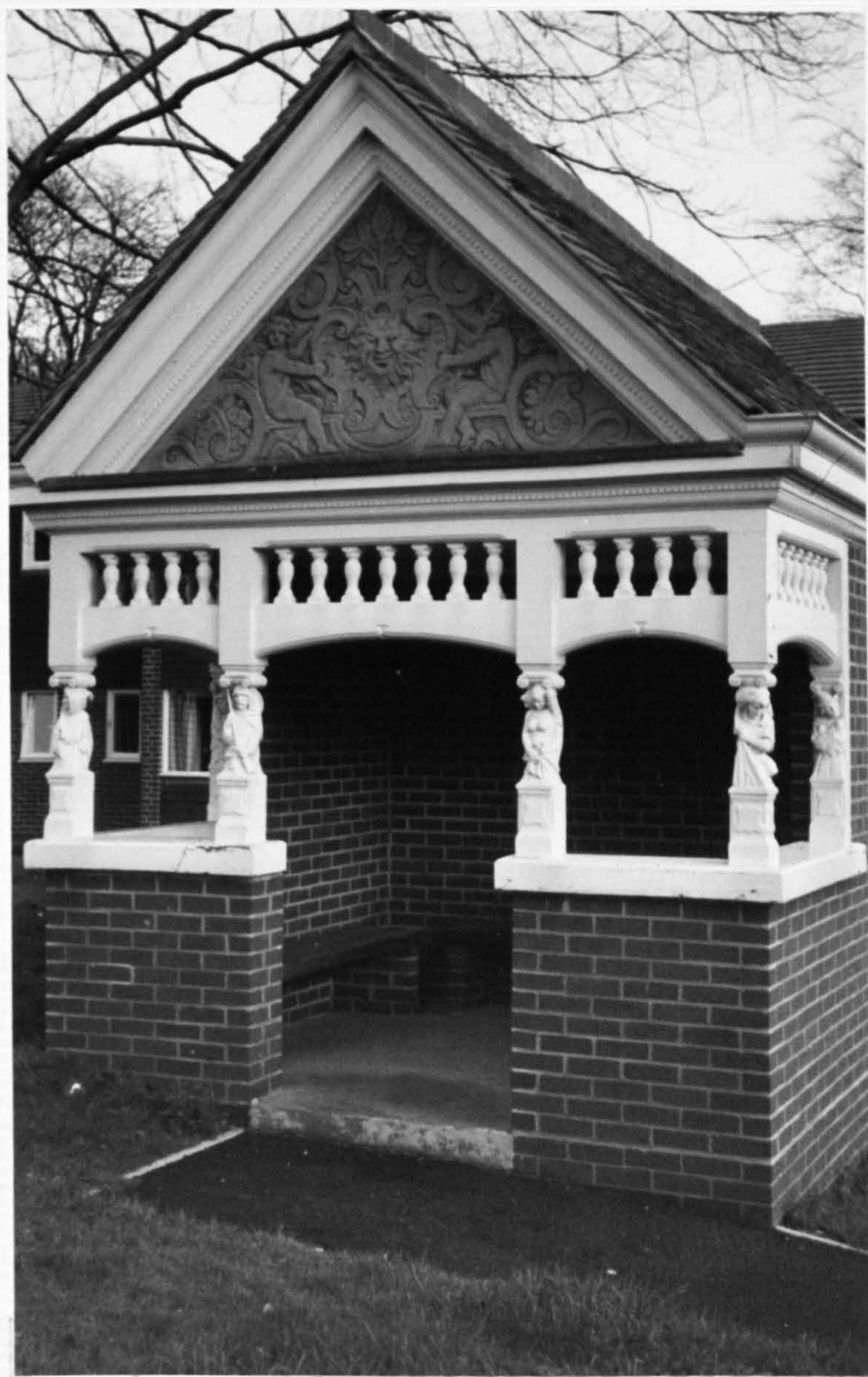
86 Original Details of Almshouses, Guildford, Surrey, 1878-79 (Cat.no.27D) incorporated into a Garden Seat, 1971
