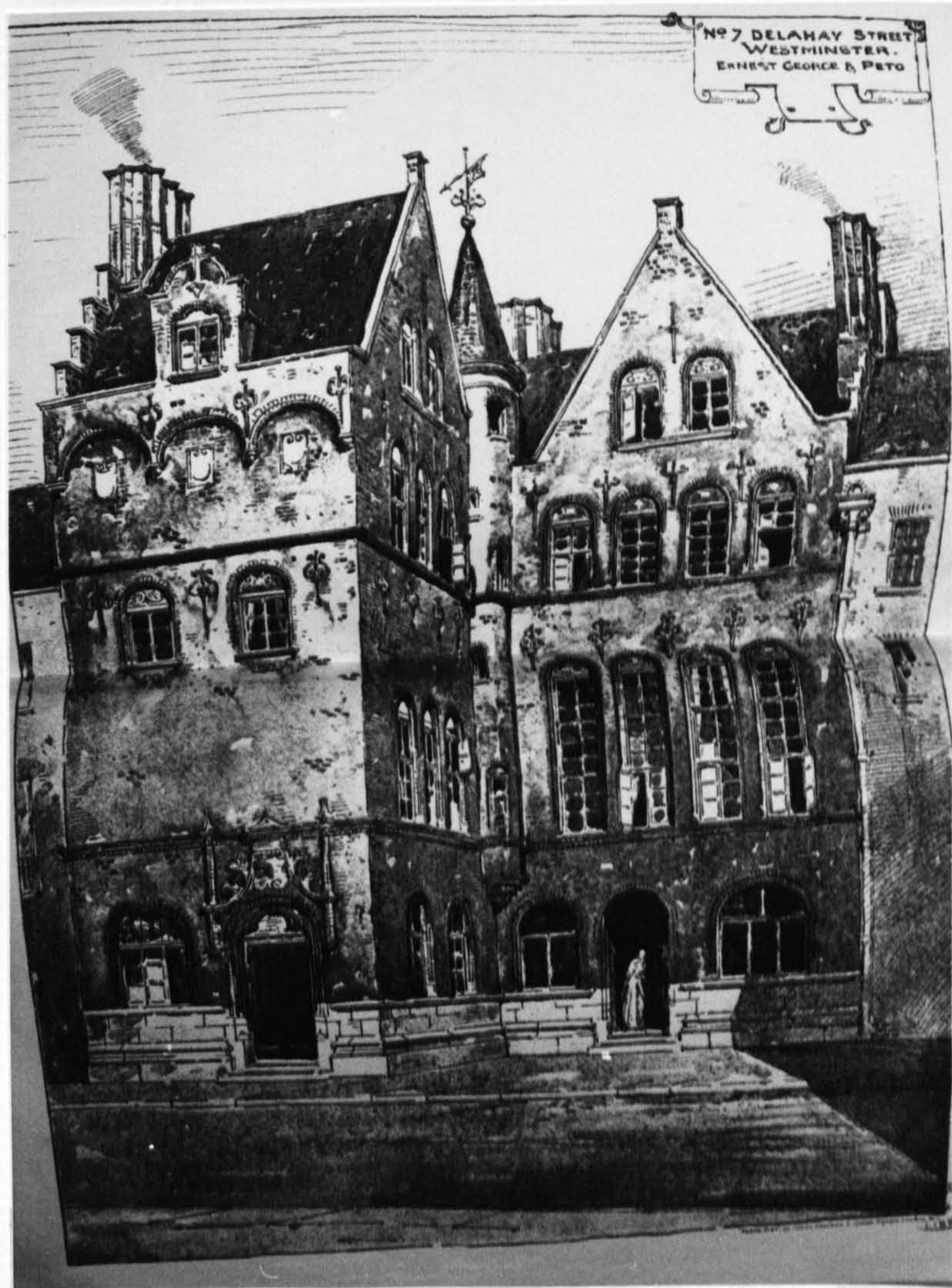
231 George and Peto, 7 Delahay Street, Westminster, London, 1892-93, now demolished, Perspective of Street Front (BN 19 May 1893 p.667); Cat.no.136
