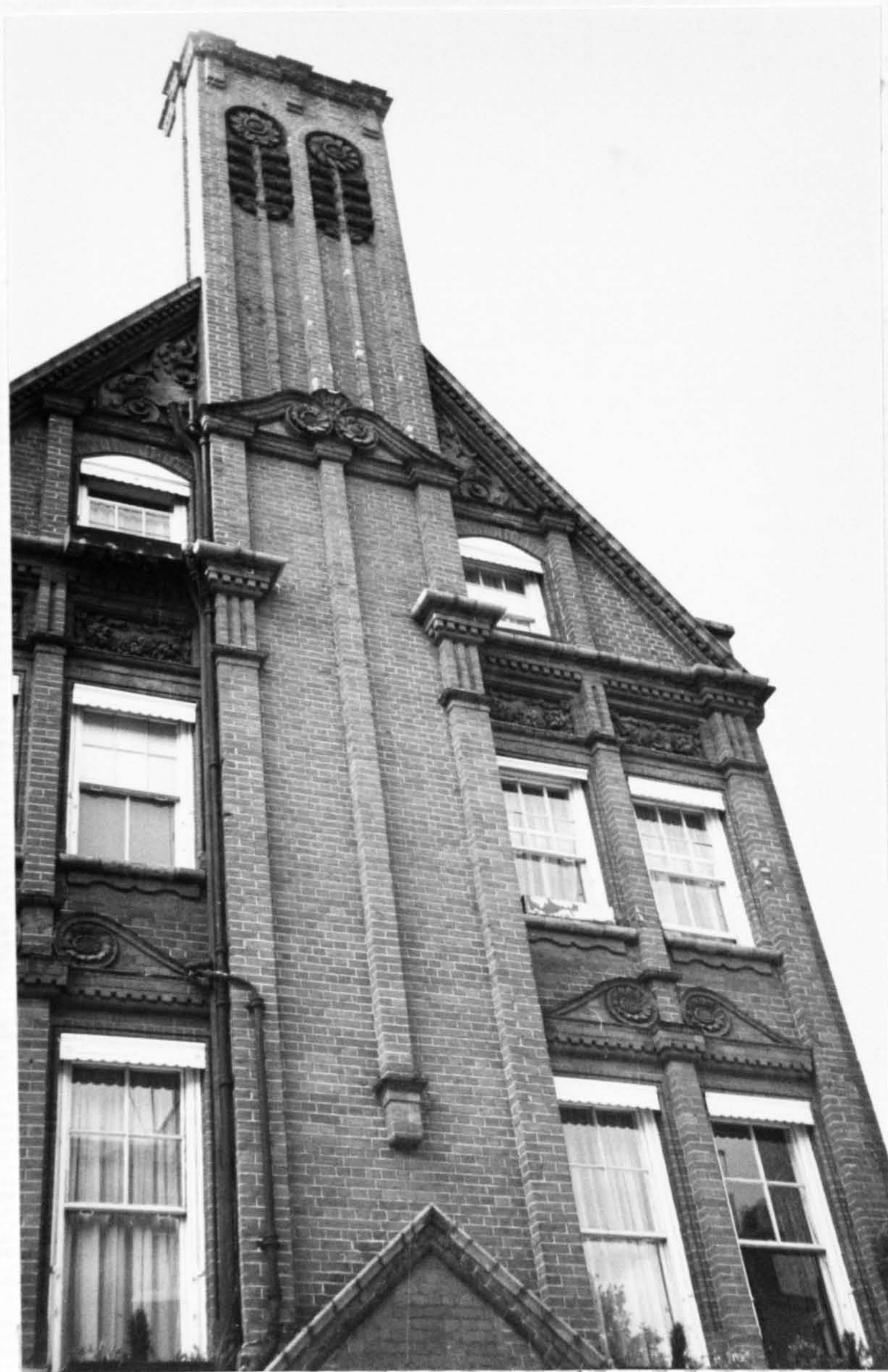
53 George and Peto, Premises for Messrs Thomas Goode & Co., 17 South Audley Street, London W1, 1876, Detail of Brick Decoration; Cat.no.22B
