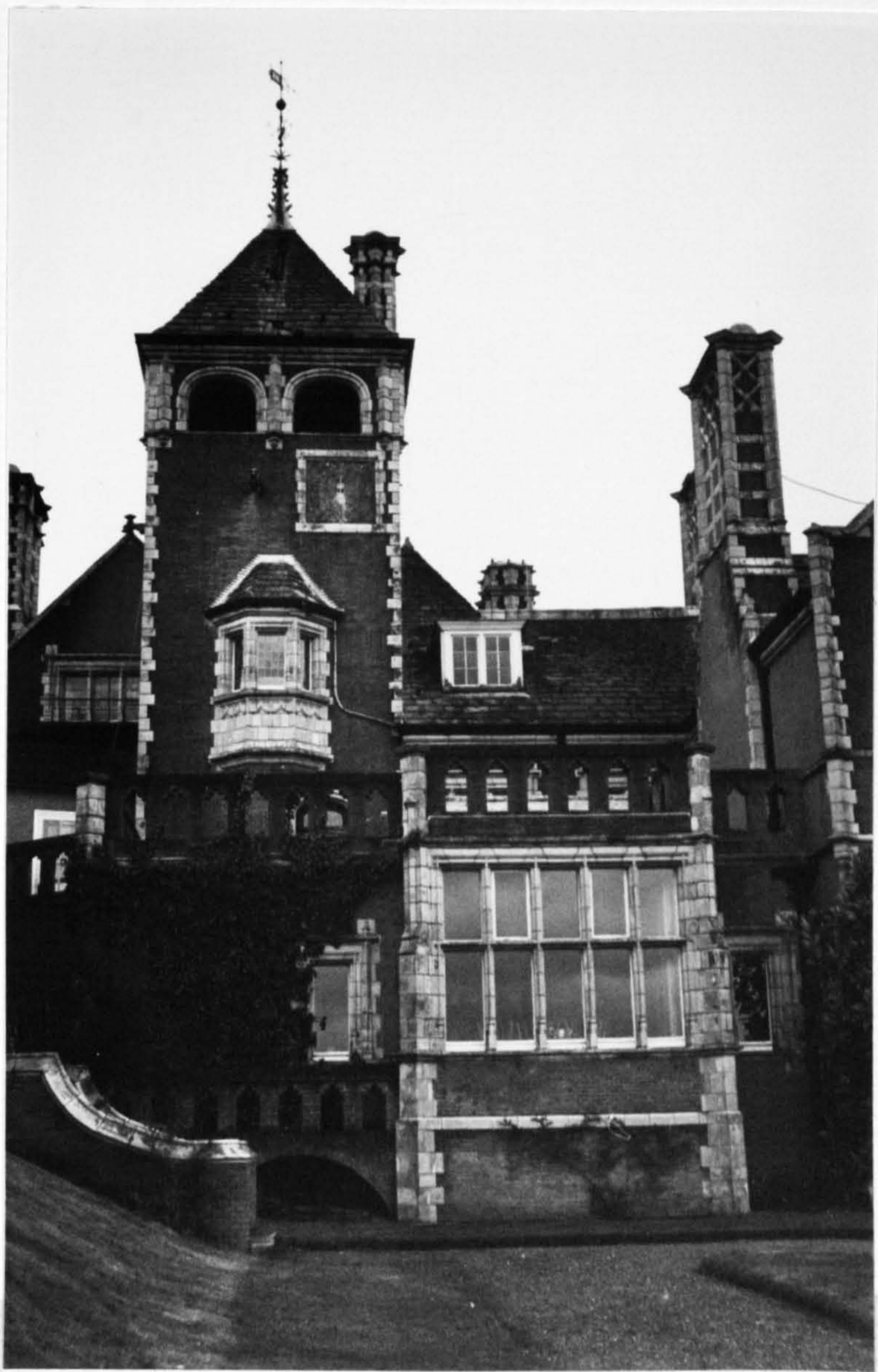
165 George and Peto, Woolpits, Ewhurst, Surrey, 1885-88, Tower, South Front; Cat.no.77
