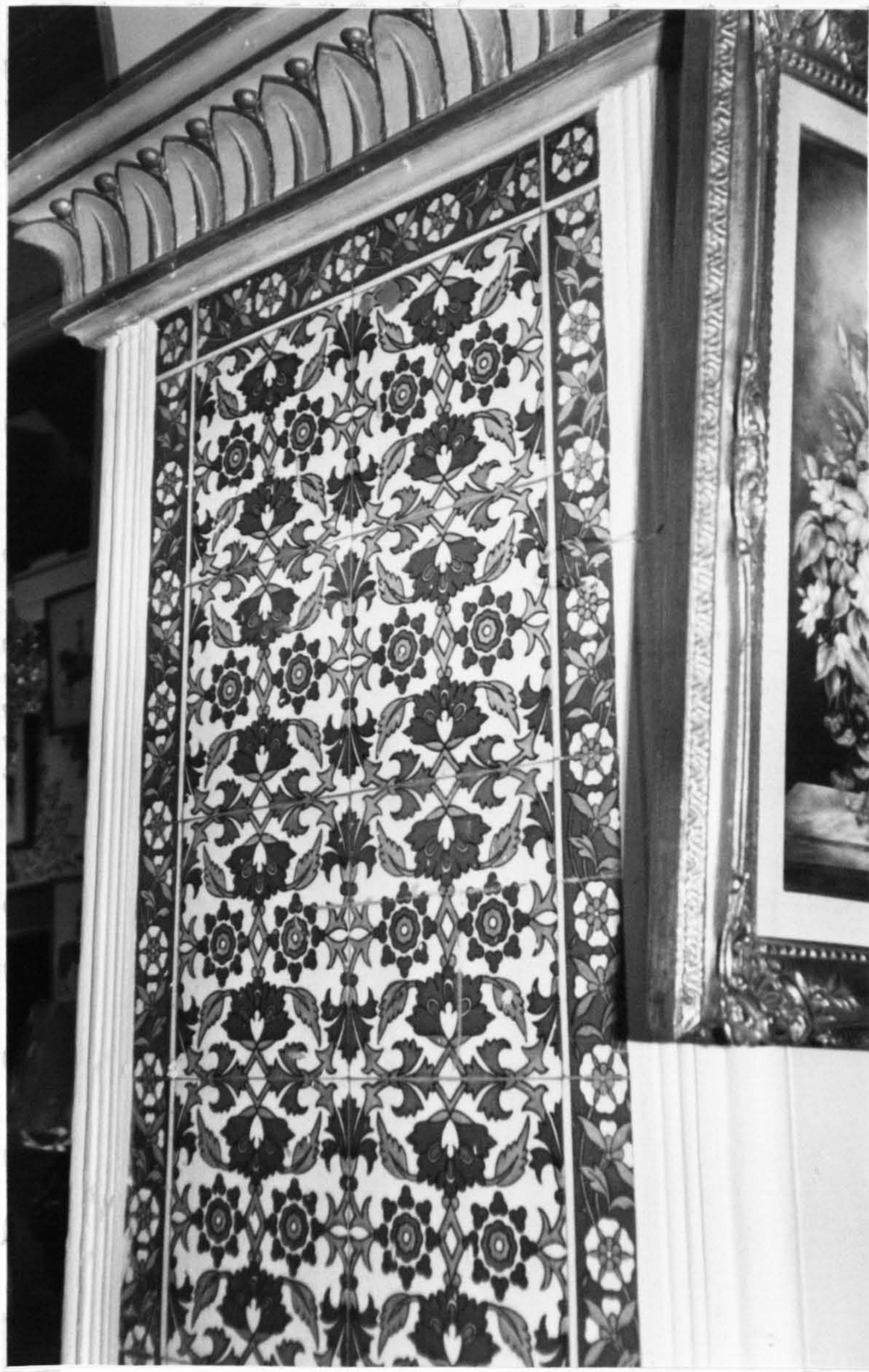
55 George and Peto, Premises for Messrs Thomas Goode & Co., 17-22 South Audley Street, London W1, 1875-76, Interior, Detail of Minton Hollins Tiles on Pillar; Cat.no.22A
