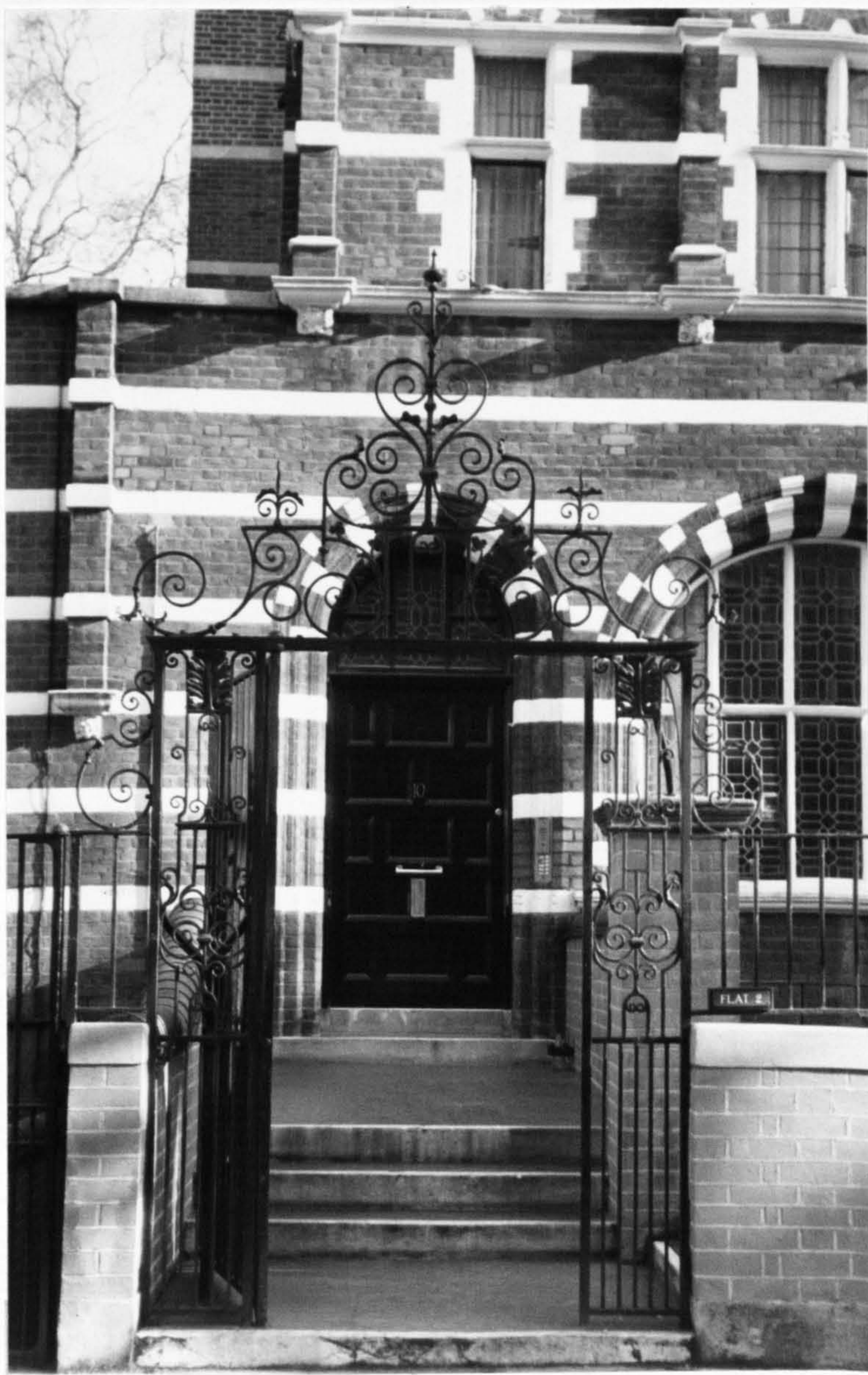
135 George and Peto, 10 Collingham Gardens, London SW5, 1884-85, Entrance; Cat.no.61H
