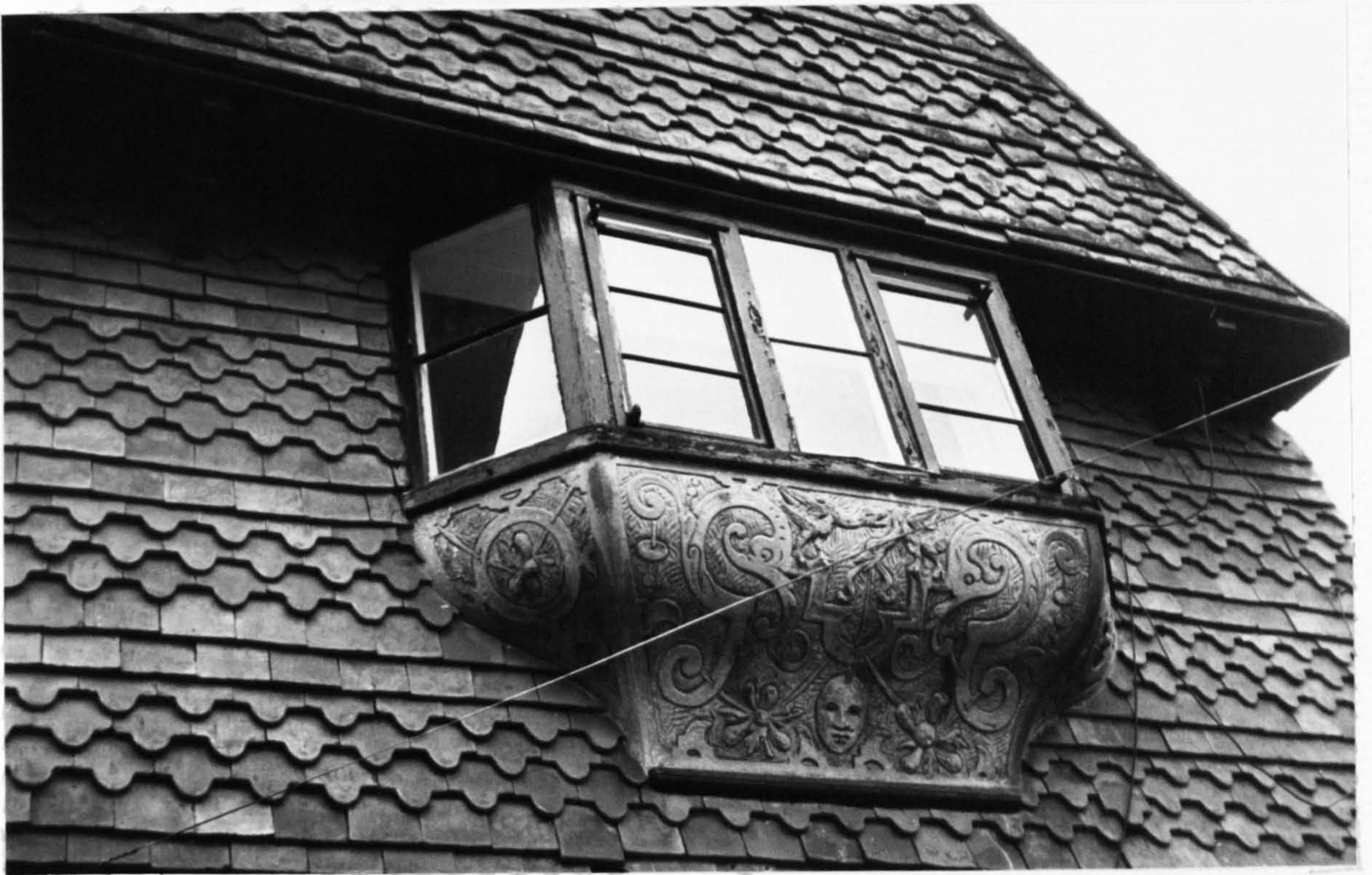
33 George and Vaughan, East Lodge, Rousdon, Devon, 1873, Detail; Cat.no.17B
