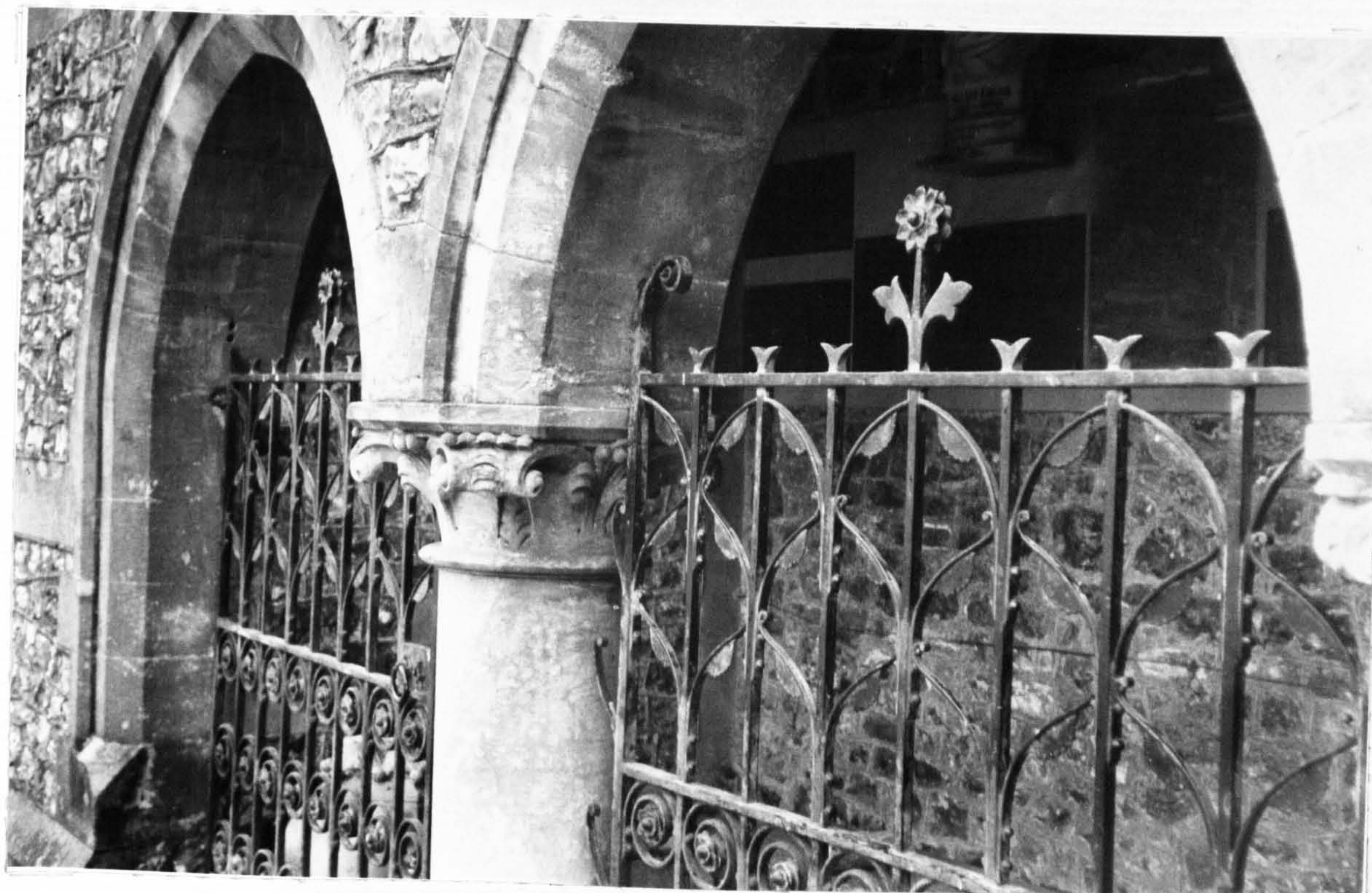
29 George and Vaughan, St. Pancras Church, Rousdon, Devon, 1872-74; Detail of Ironwork; Cat.no.17A
