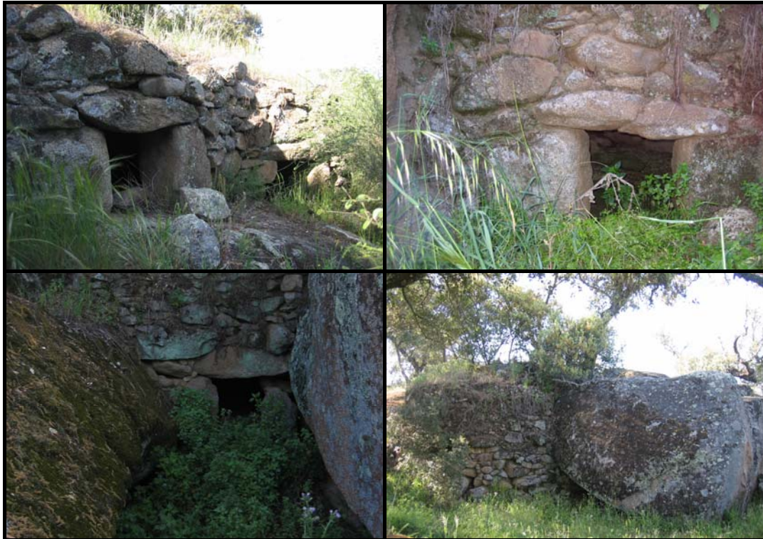
Figure 6.13: Stone-built parideras or breeding spots, possibly dating earlier than the 20th century. Granitic boulders are incorporated in the structure, saving useful smaller stones and labour.
