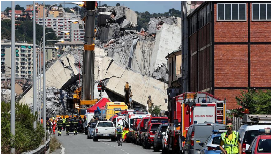
Figure 1-1 Collapse of the Morandi Bridge in Genoa, August 2018
