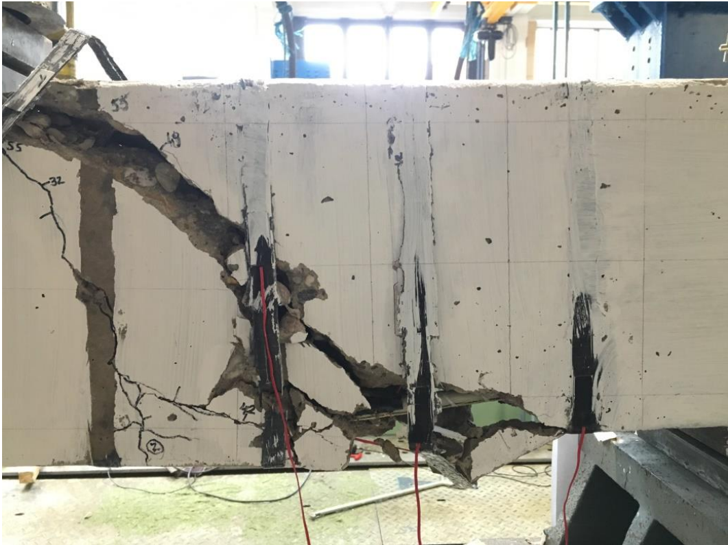
Photo 13 Shear failure of GB63
