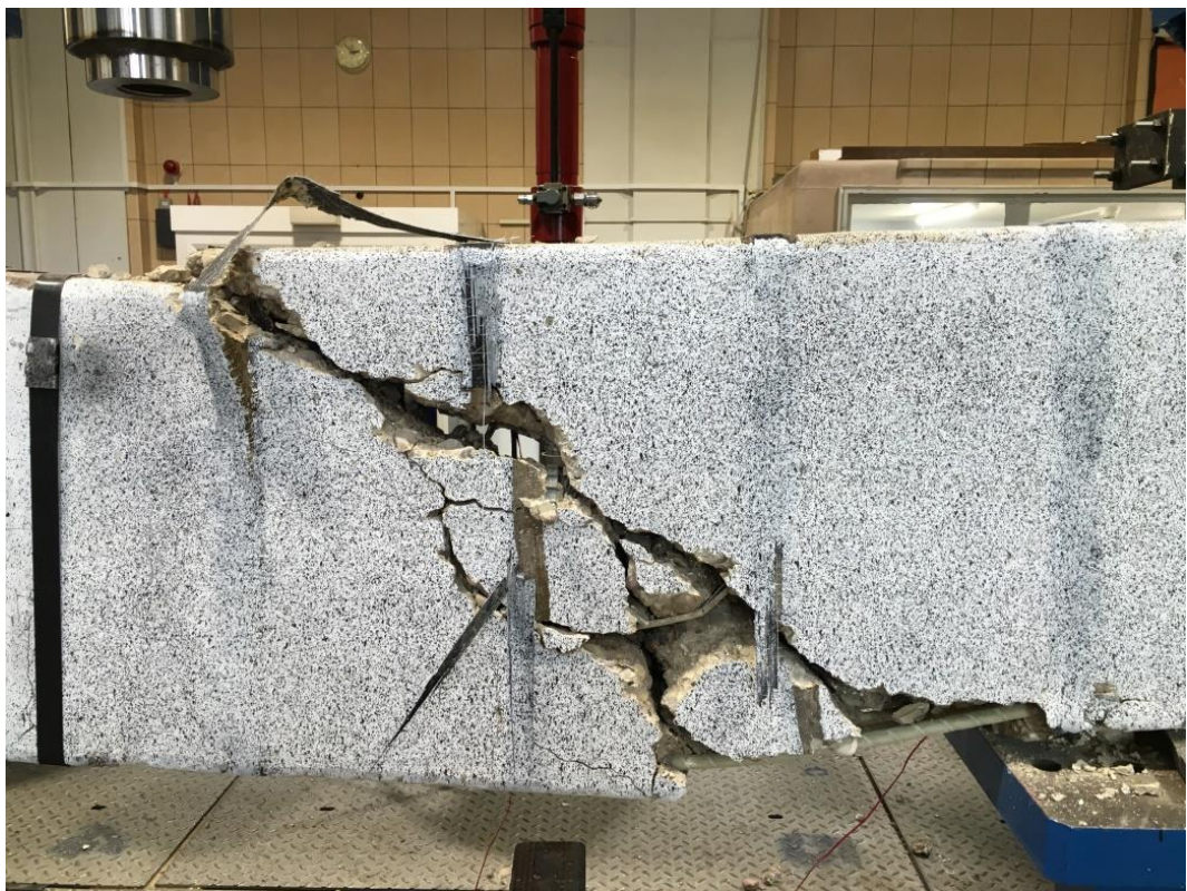
Photo 20 Shear failure GB61 (DIC side)
