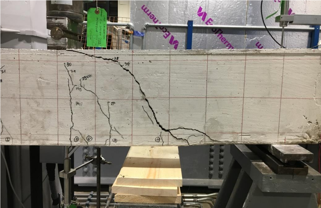
Photo 1 Shear failure in GB58-0
