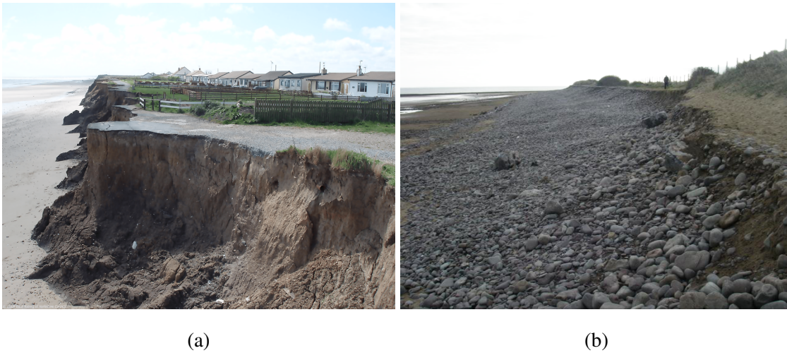
Figure 1.1: Cliff erosion at Ulrome, East Riding of Yorkshire (left panel). Source: Channel Coastal Observatory [55]. Coastal erosion at Minehead, Somerset (right panel). Source: Channel Coastal Observatory [50].
