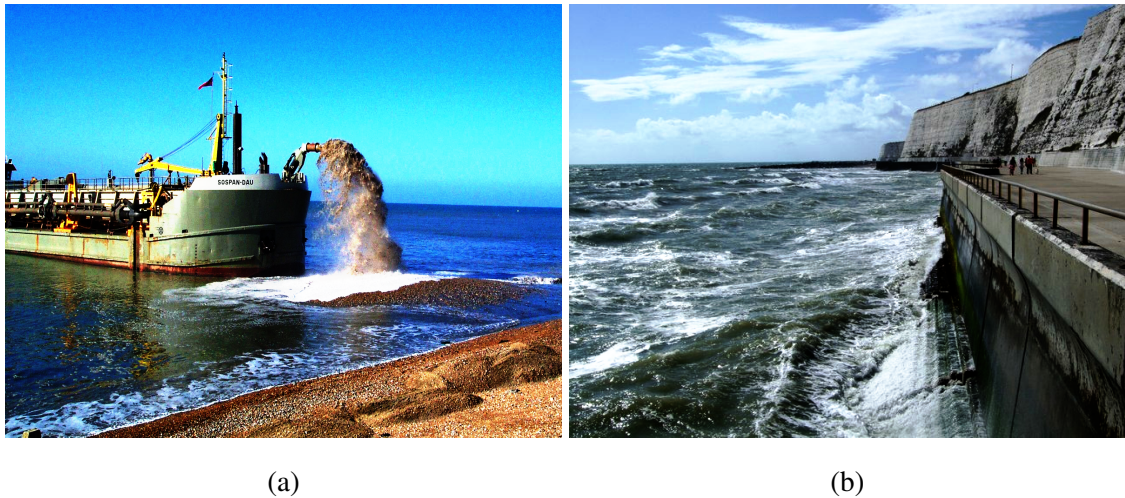
Figure 1.2: Beach re-nourishment, Pevensey bay (left panel). The dredger is located as close as possible to the beach and is pumping sediment to the beach through the tube. Source: Pevensey Coastal Defence Ltd [49]. Rough seas near Saltdean, Brighton (right panel). Seawall, built in 1933 to protect the coastline as part of the Undercliff Walk. Source: The Geograph, Britain and Ireland project [32].
