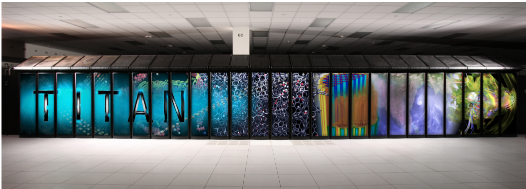
FIGURE 1.5: TITAN Supercomputer at Oak Ridge National Laboratory[15].
