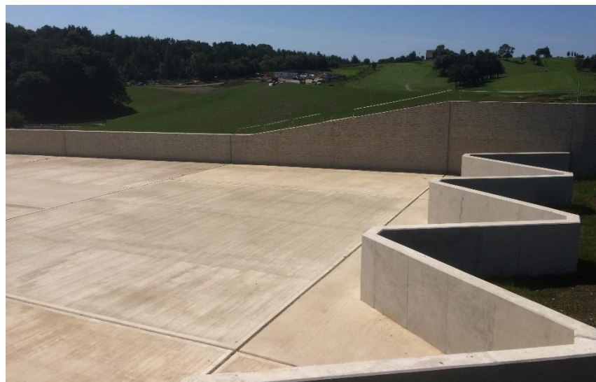
Figure 5.4: View of the labyrinth weir from the left hand side of the scheme
