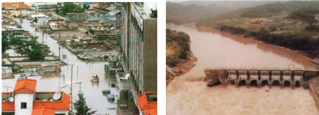
Figure 6.7 Submerged Paju in Gyeonggi province and collapsed Yeoncheon dam
