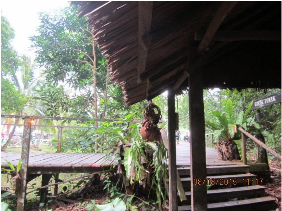
Figure 4.52: The stairs beside the Penan Hut leading to the plankwalk (the main pedestrian pathway). (Photo: J. Chieng; August 8, 2015)
