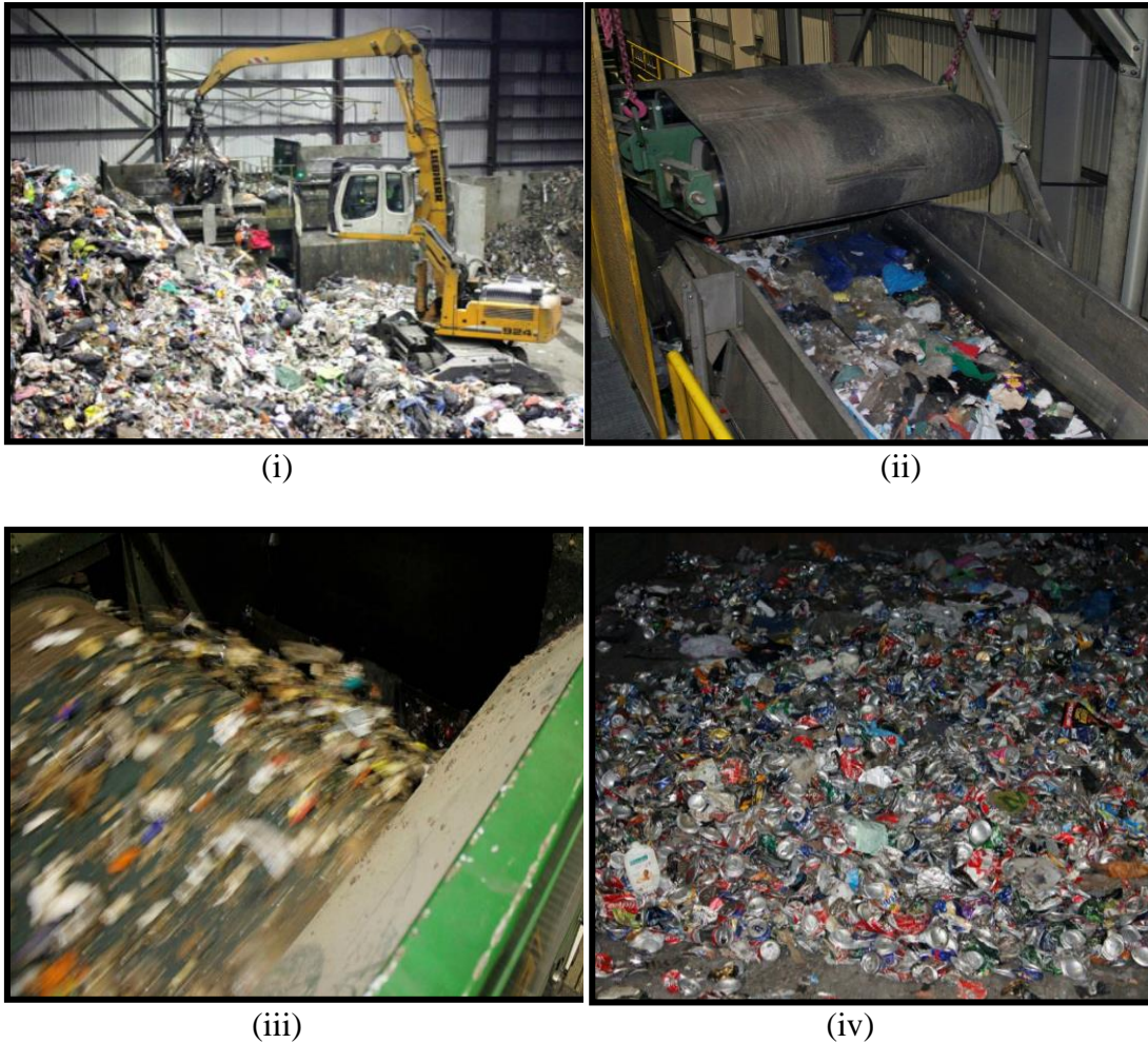
Plate 3. 3: The waste facility showing (i) the grab loader feeding the shredder, (ii) the over-band magnet, (iii) waste in the eddy current separator, and (iv) the non-ferrous bay(AWM, 2011).
