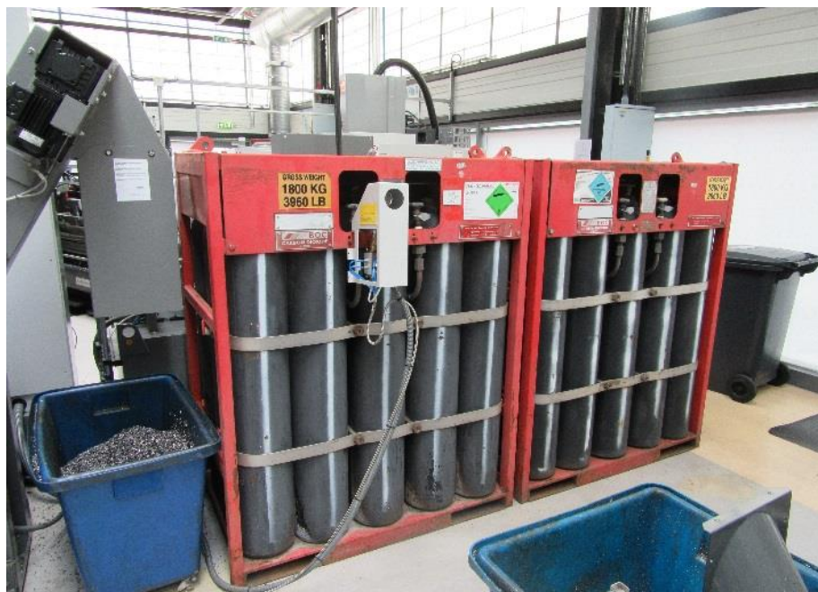
Figure 3-24. Twelve high-pressure (near 62 bar) cylinders connected in series containing liquid carbon dioxide.
