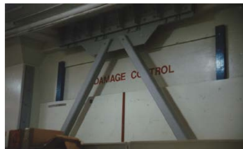
Fig.2.10Diagram of viscoelastic damper[93] Fig.2.11Viscoelastic damper in a civil building [94]
