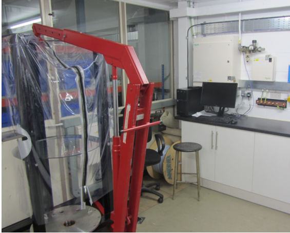
(a) Maintenance frame and control PC
