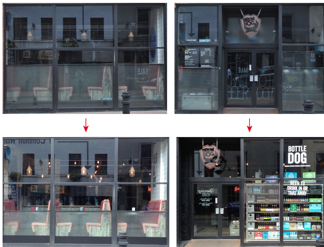
Figure 71 – Changes made to Bar 1.1 and 1.2 on walked side of Street 4; before on top, after below
