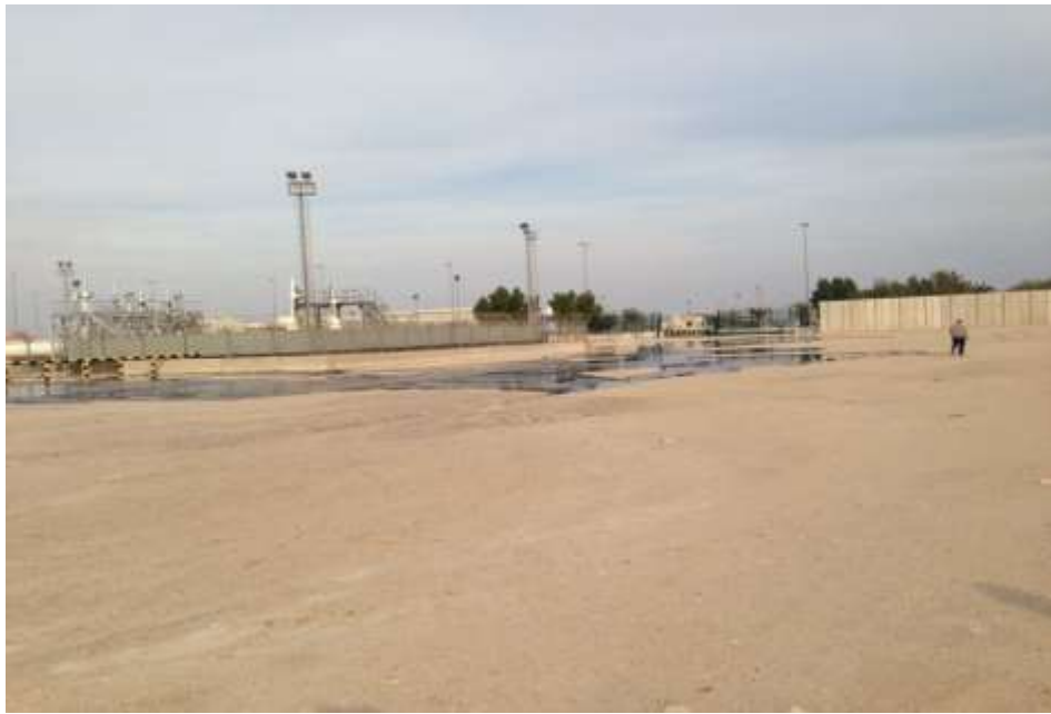
Figure 1-3: Gasket Failure leak in Cross-Over Manifold, Kuwait Oil Company (Original/Fieldwork).
