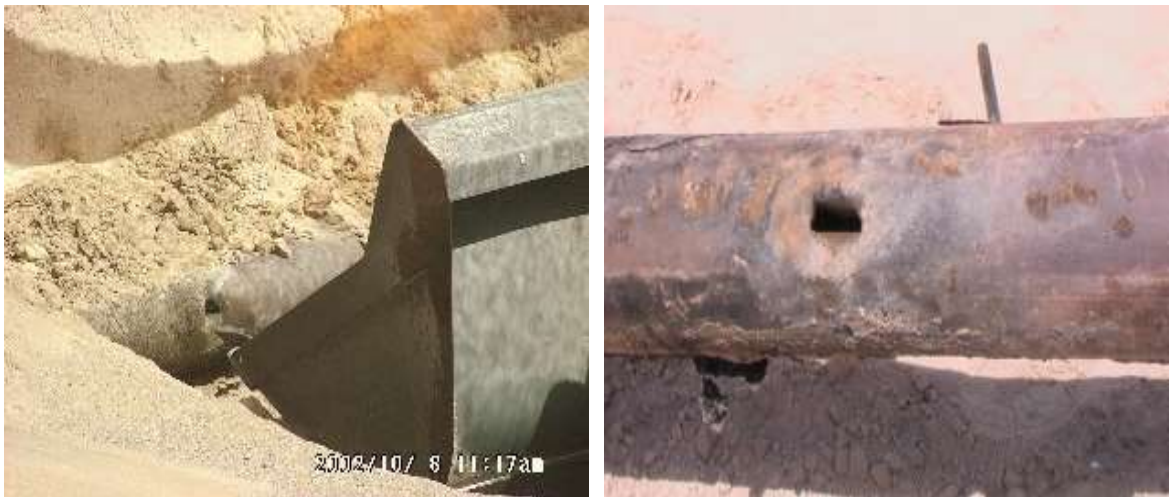
Figure 1-5: Third party damage by excavator on GC-20 HP Gas pipeline [6].
