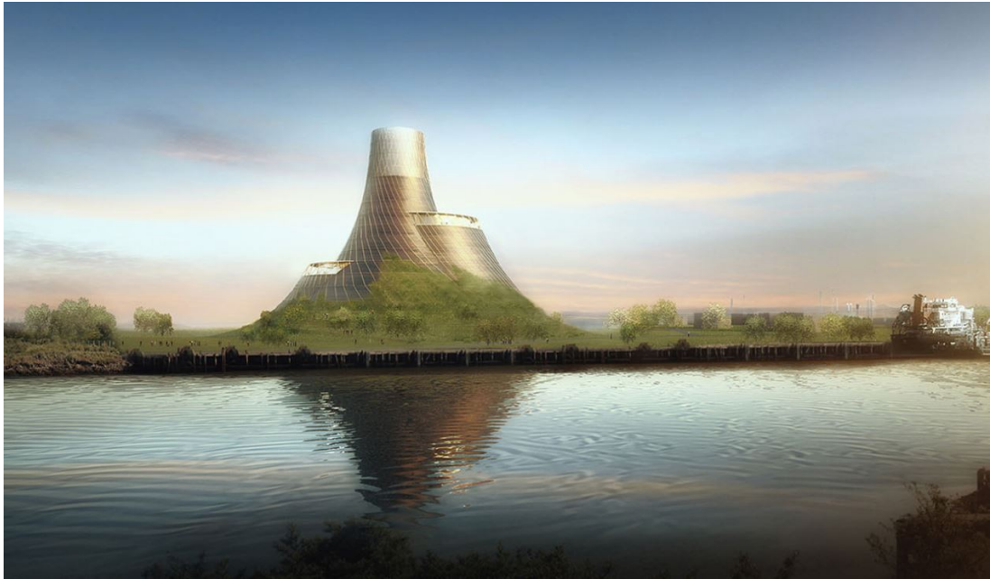
Figure 1 New infrastructural architectures: BEI Teesside waste-to-energy facility (credit: Heatherwick Studio).
