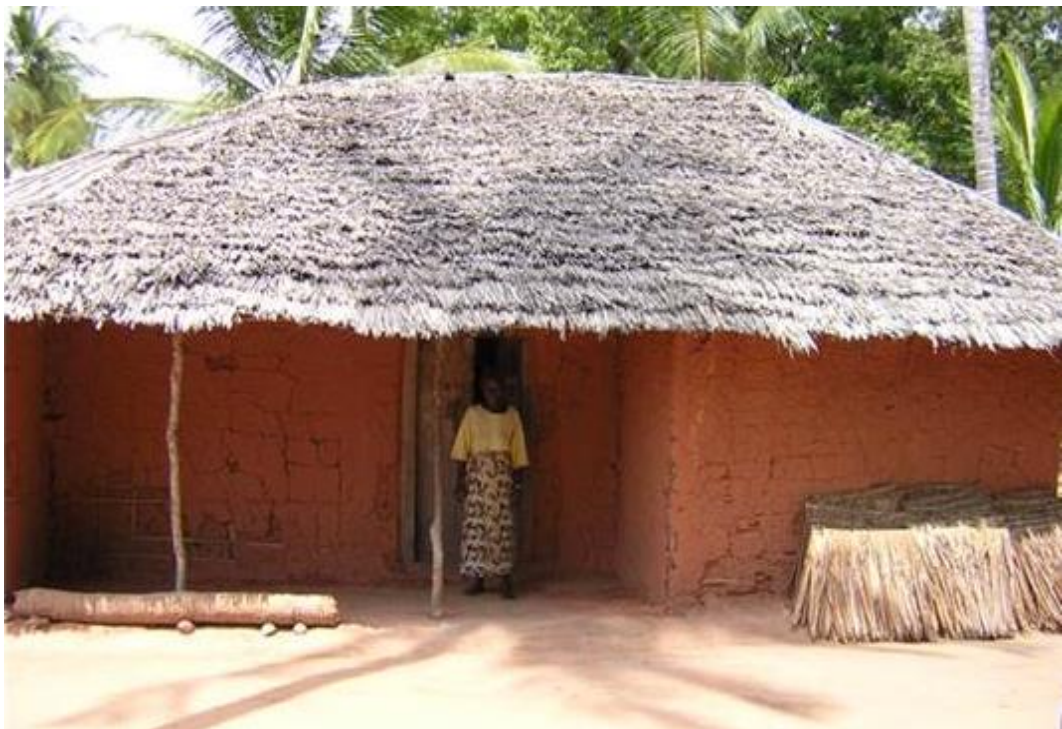
Figure 6 Modern Wattle and Daub structure at Kilwa. Image courtesy of S. Wynne-Jones
