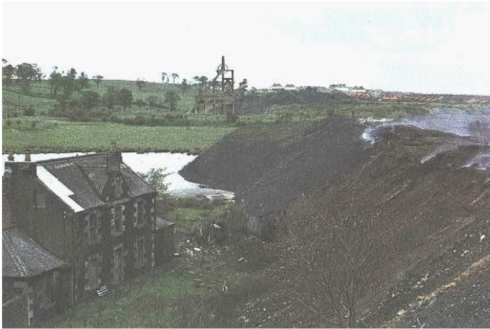
Figure 2.2. Derelict mining land and burning spoil heap at Glenraig, near Lochgelly, Fife in the 1960s (Michael Martin collection, used with permission). The structure in the background is now incorporated in Lochore Meadows Country Park.
