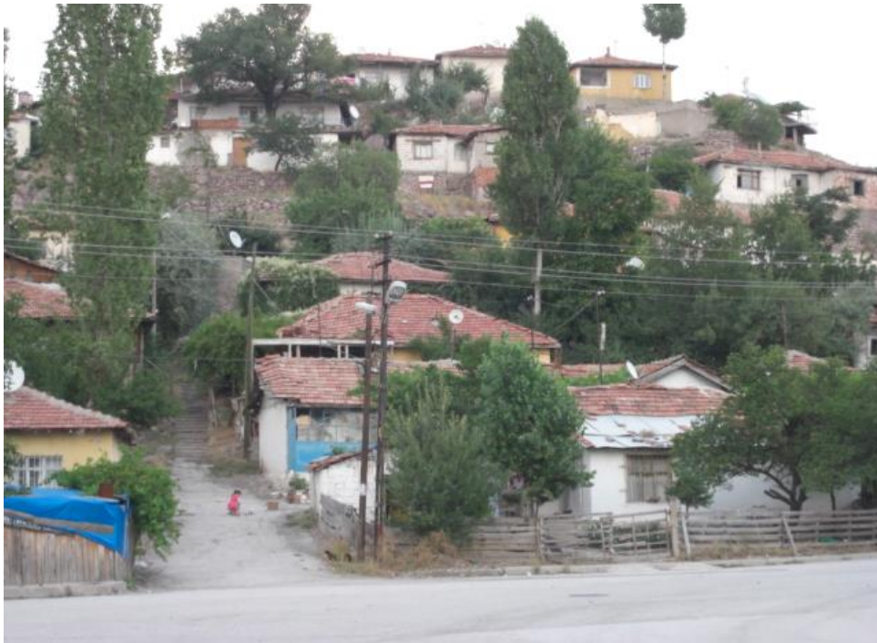
Figure 9-6: Gecekondus and gardens before the demolition in Baspinar neighbourhood. Source: Sinan Akyuz (2016)
