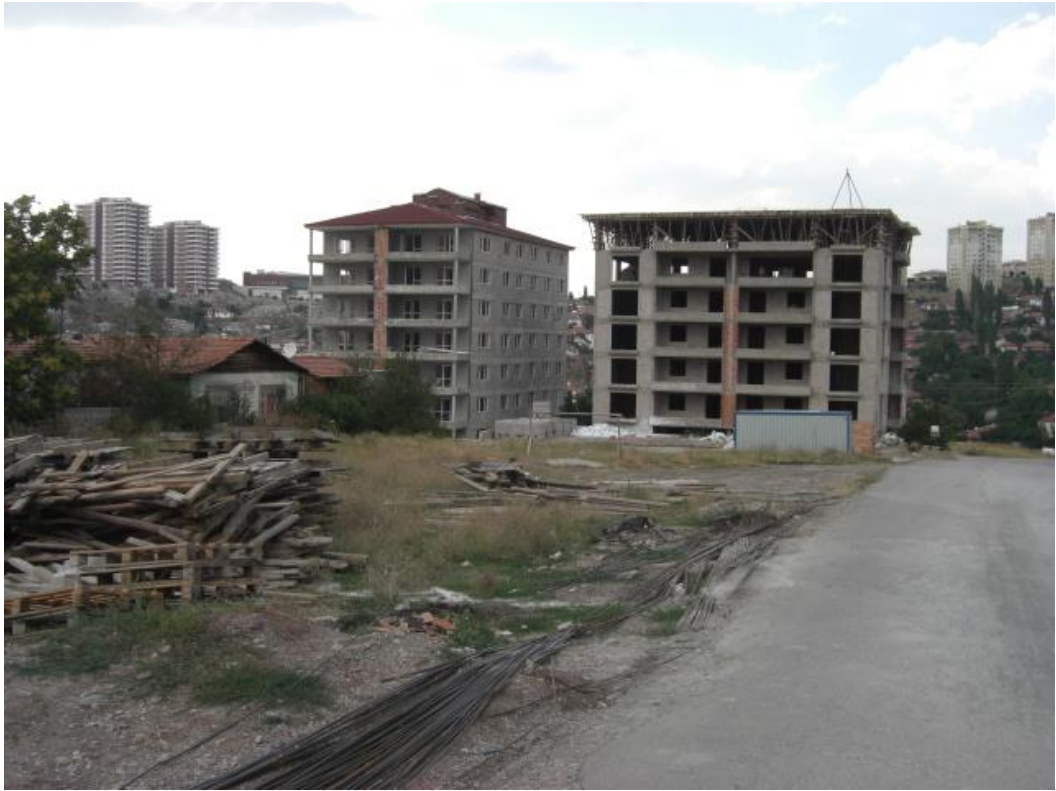
Figure 9-10: Newly constructed flats in Baspinar Neighbourhood, through IDP.
