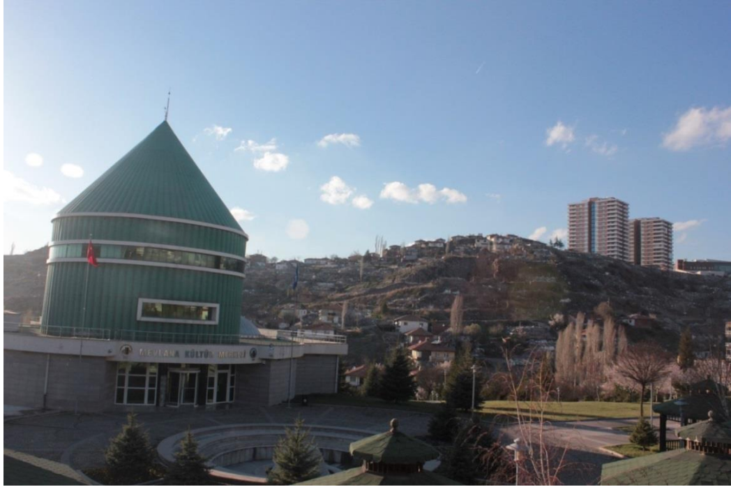
Figure 9-8: Demolished Gecekondus in the Baspınar Neighbourhoods in the distance, on hillside. Source: Sinan Akyuz, 2016
