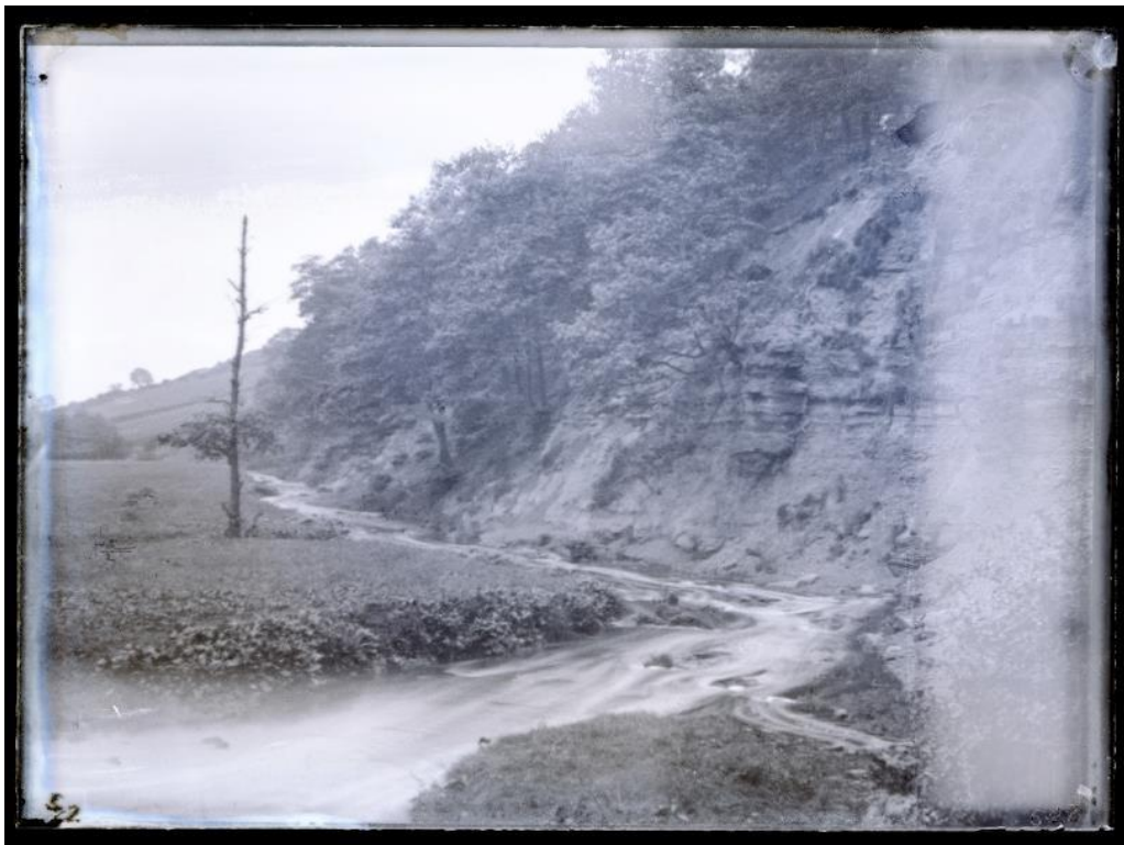
Figure 95 - Headingley, Beck Street, 1888, by Godfrey Bingley
