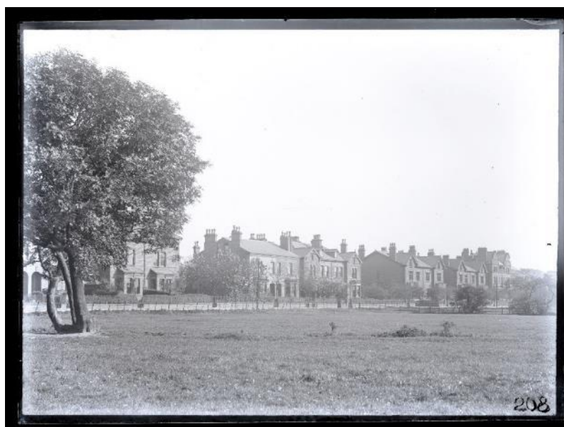
Figure 46 - Cardigan Road from field, near Kirkstall Lane (1887) by Godfrey Bingley
