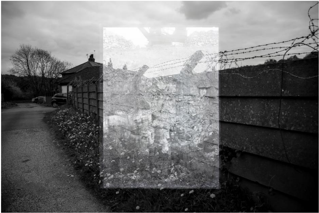
Figure 43 - Quarry Valley (Projection) 1905-2017
