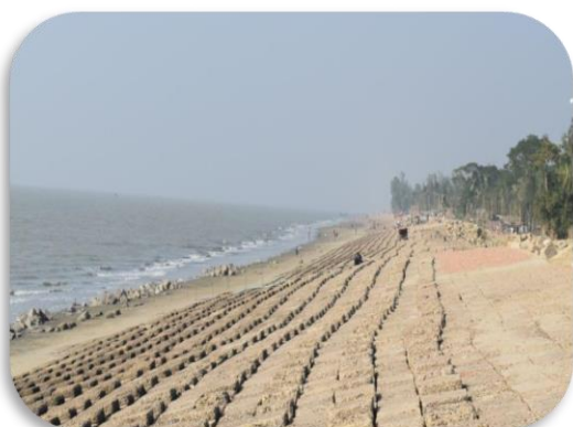
The hard defence structure at Kutubdia island in the eastern coastal zone substantially reduced erosion.
