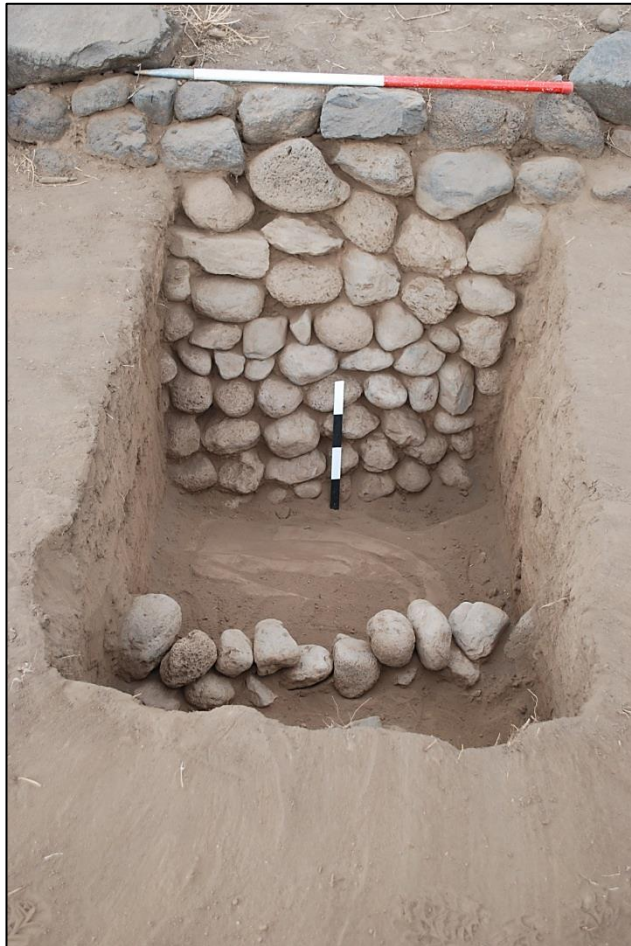
Figure 11: Primary terrace wall (in the background of the image) showing several courses of construction, while in the centre of the image, courses of the irrigation canal wall can be seen. The primary terrace wall functioned both for sediment capture and as one wall of the irrigation canal that ran in front of it.
