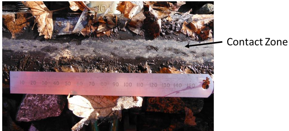
Figure 105- Photo of railhead showing leaf layer contamination at braking point
