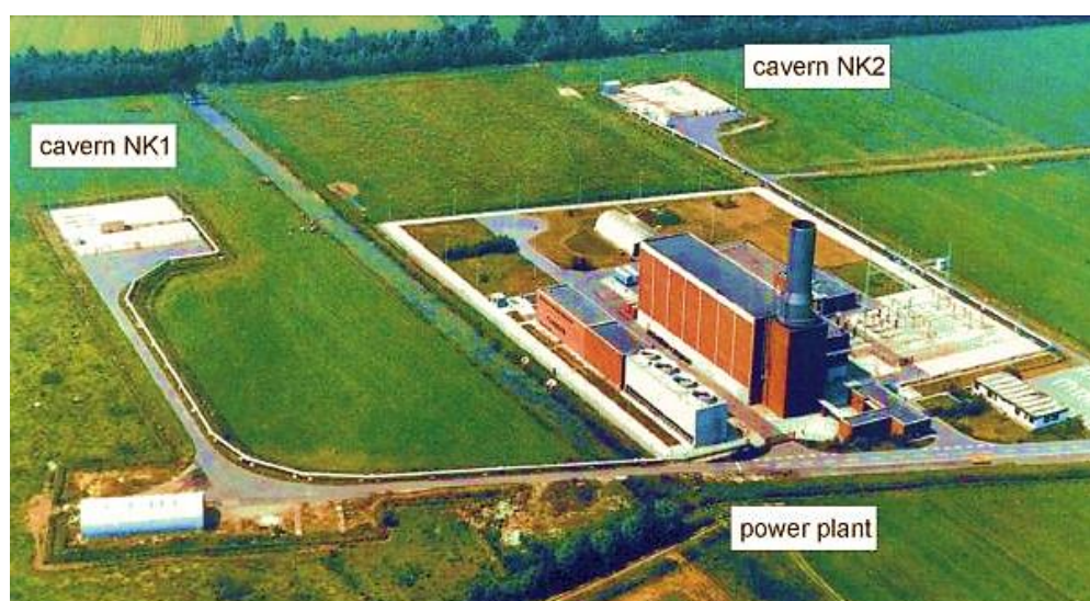
Figure 2-9. The Huntorf CAES plant in Germany (Bullough, 2004).
