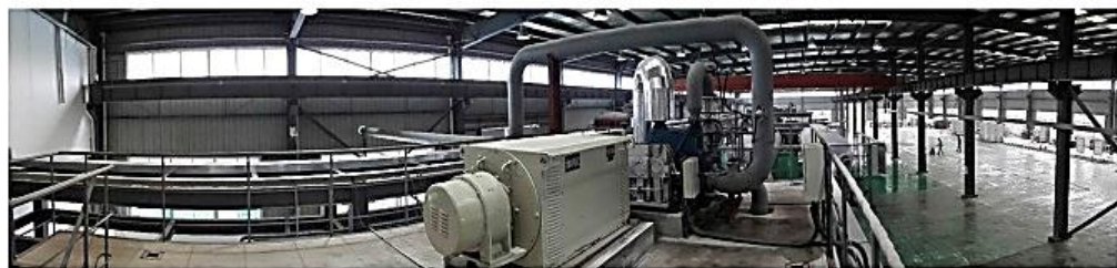
(b) Side view of the pilot plant
