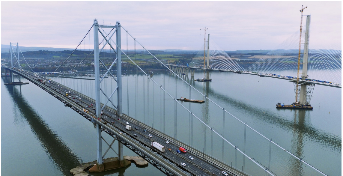
Figure 1.2: The Forth Road Bridge (front) alongside the Queensferry Crossing Bridge (back), image downloaded from https://www.theforthbridges.org/forth-road-bridge/ .
