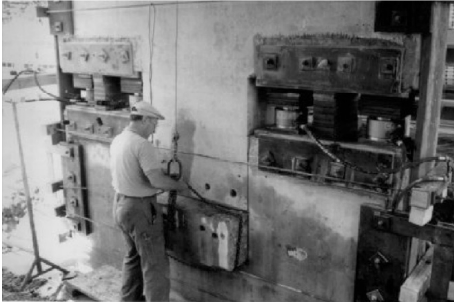
Figure 3.3: The hydraulic system used for settling the pier [119].
