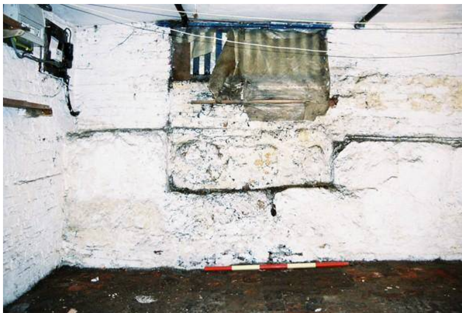
Fig. 113 2 Precentors' Court, north wall with the blocked doorway and flagstones on the floor.
