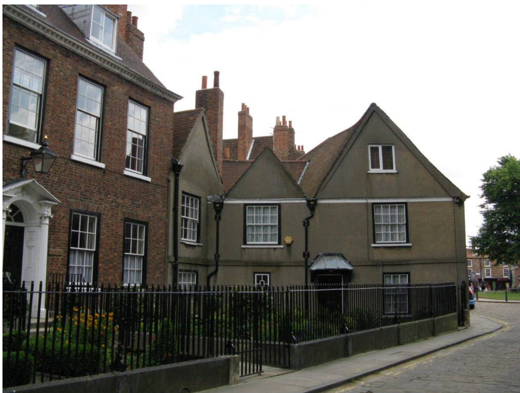
Fig. 33 N. 4 Minster Yard. The Mansion of Langtoft, from the north, looking at the medieval high-end wing.
