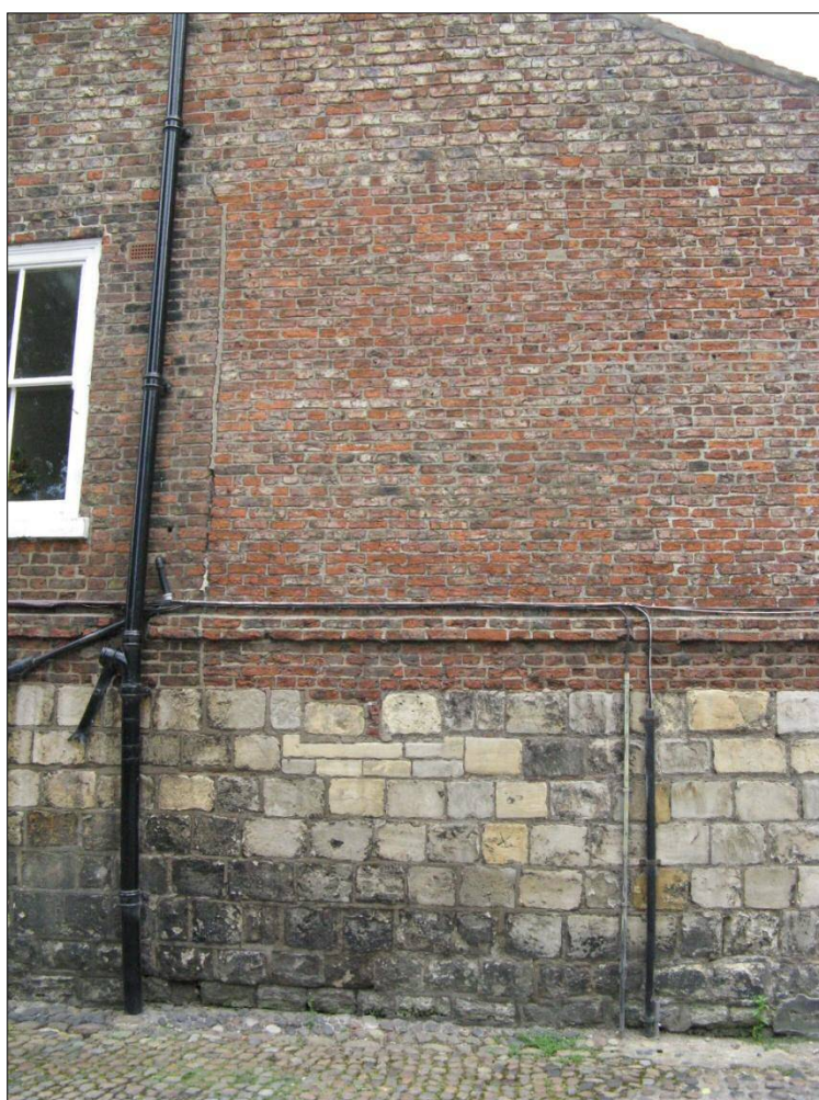
Fig. 38 17 th C redevelopment and later developments on the medieval service range of the mansion of Langtoft.
