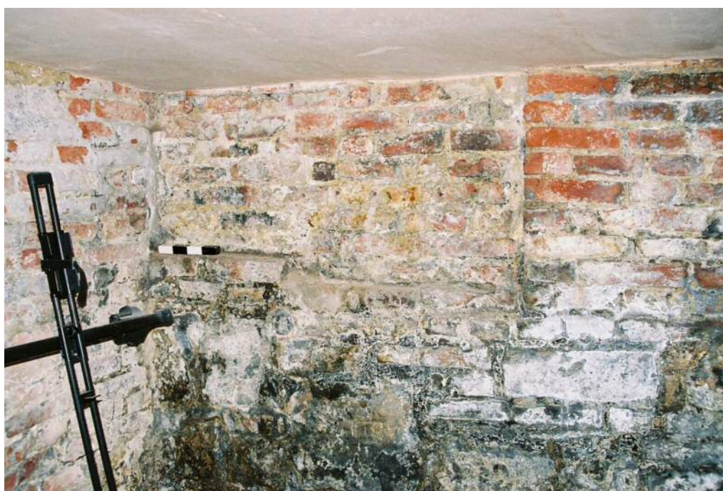
Fig. 120 3 Precentor's Court, north wall, detail with blocked window.
