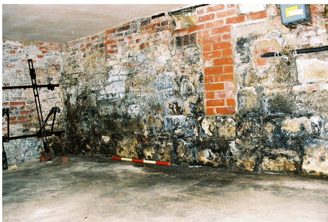
Fig. 118 3 Precentor's Court, north wall.
