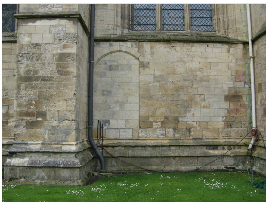
Fig. 58 Bay six of the northern aisle, showing the blocked doorway.
