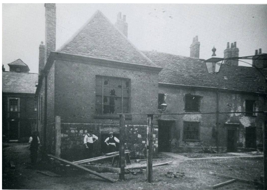
Fig. 18 The Subdeanery from the south-east, being demolished in advance of construction of Purey Cust hospital, 1913 ( YAYAS published in Buttery, Vanished Buildings , p. 10). Showing the great chamber, the hall range (however, the portico or stair tower had been demolished) and the service end with a fireplace.
