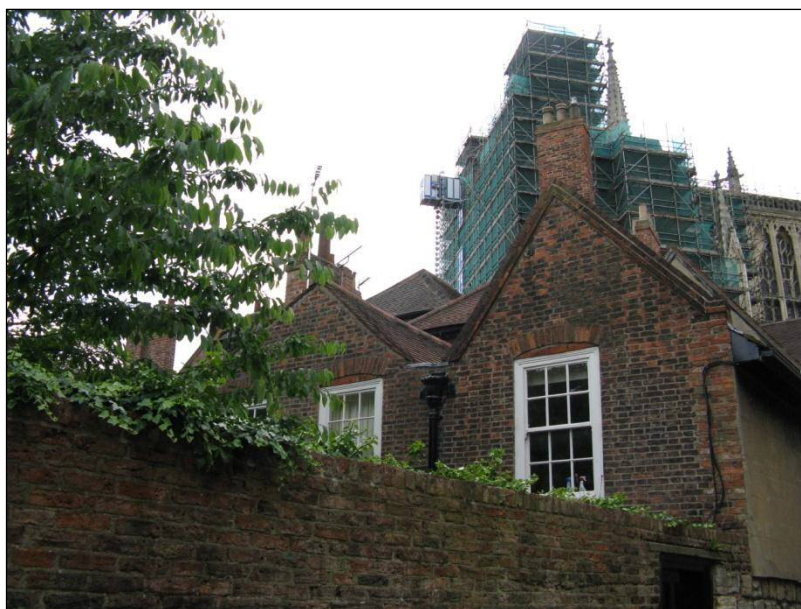
Fig. 40 N. 3 Chapter House Street, showing the early 17 th C cross wing on the left.
