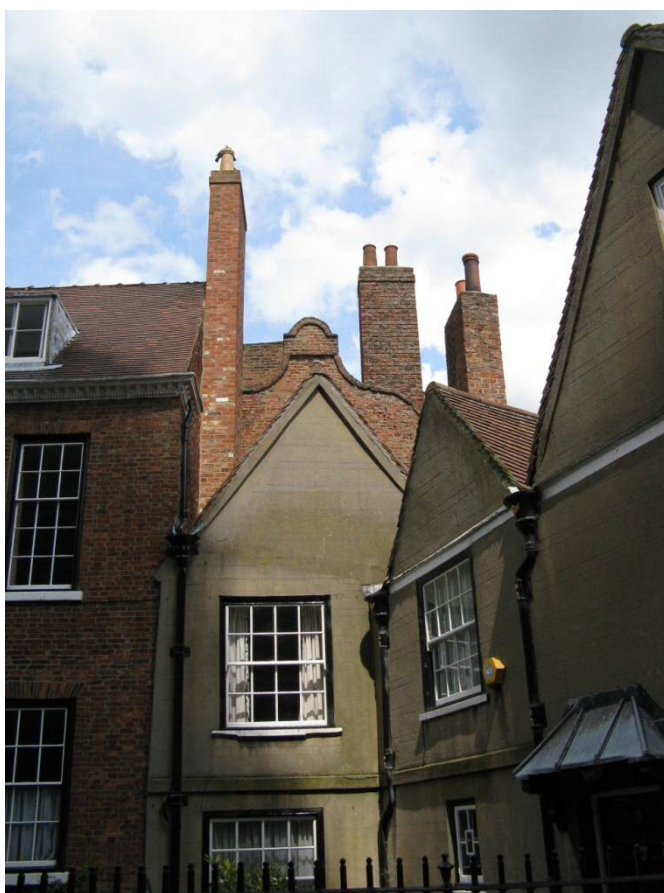
Fig. 35 17 th C Dutch gable on the hall wing of the Mansion of Langtoft.
