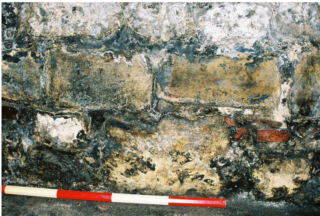
Fig. 119 3 Precentor's Court, north wall, detail.
