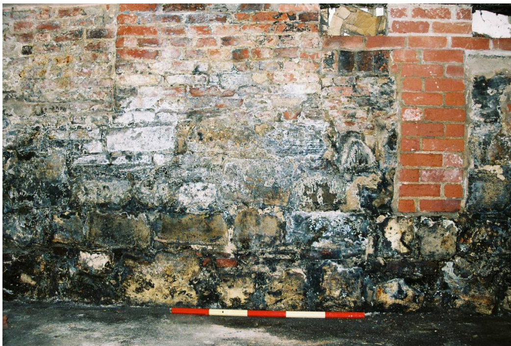
Fig. 117 3 Precentor's Court, north wall.
