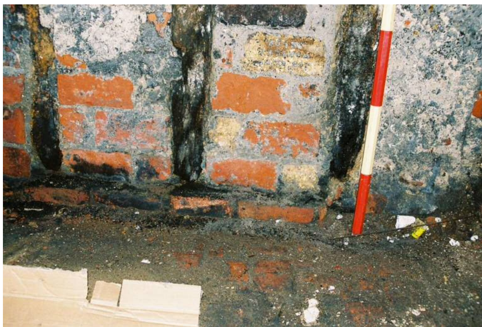
Fig. 116 2 Precntor's Court. West cellar, showing timber and tile partition.
