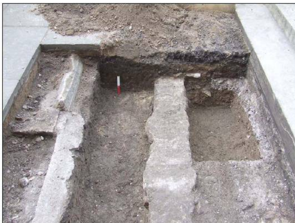
Fig. 21 Limestone wall of the bookshops to the east of the cathedral south door, facing south (in Dean, 'Minster Yard and Minster Gates', p. 17).
