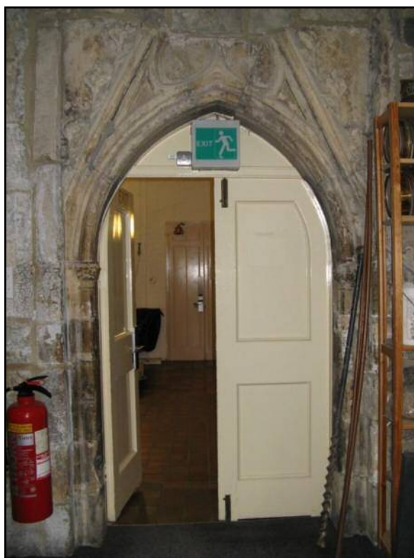
Fig. 93 King's Manor. Reused architectural sculpture in the undercroft.
