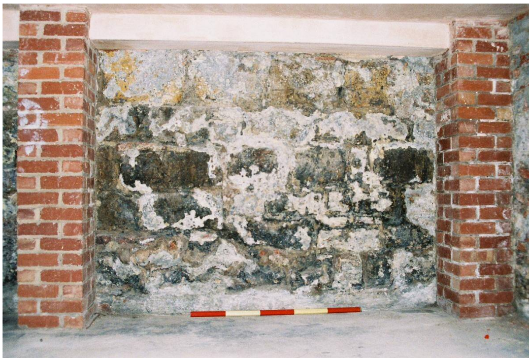
Fig. 121 3 Precentor's Court, south wall.
