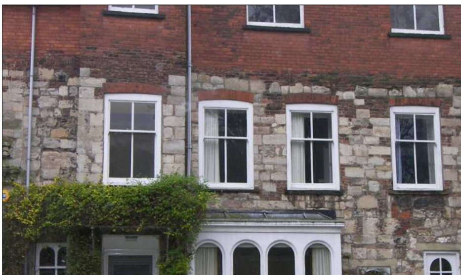
Fig. 15 Details of northern face of the house, showing two phases of brick construction.
