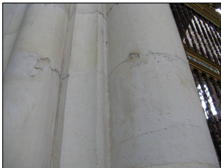
Fig. 102 The mortice and peg holes for the Consistory screen.
