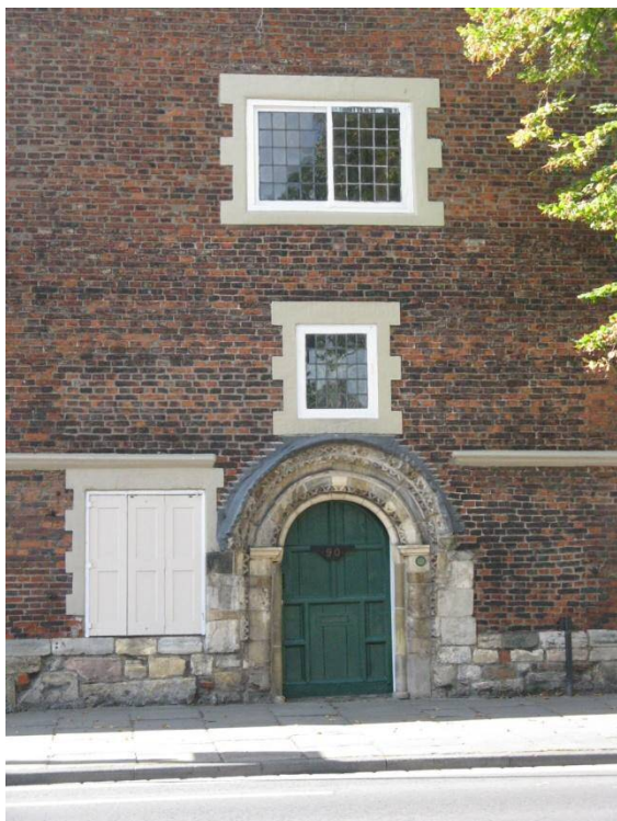
Fig. 109 York, Ingram Almshouses, Bootham, showing reused building material of Roman and medieval origin.
