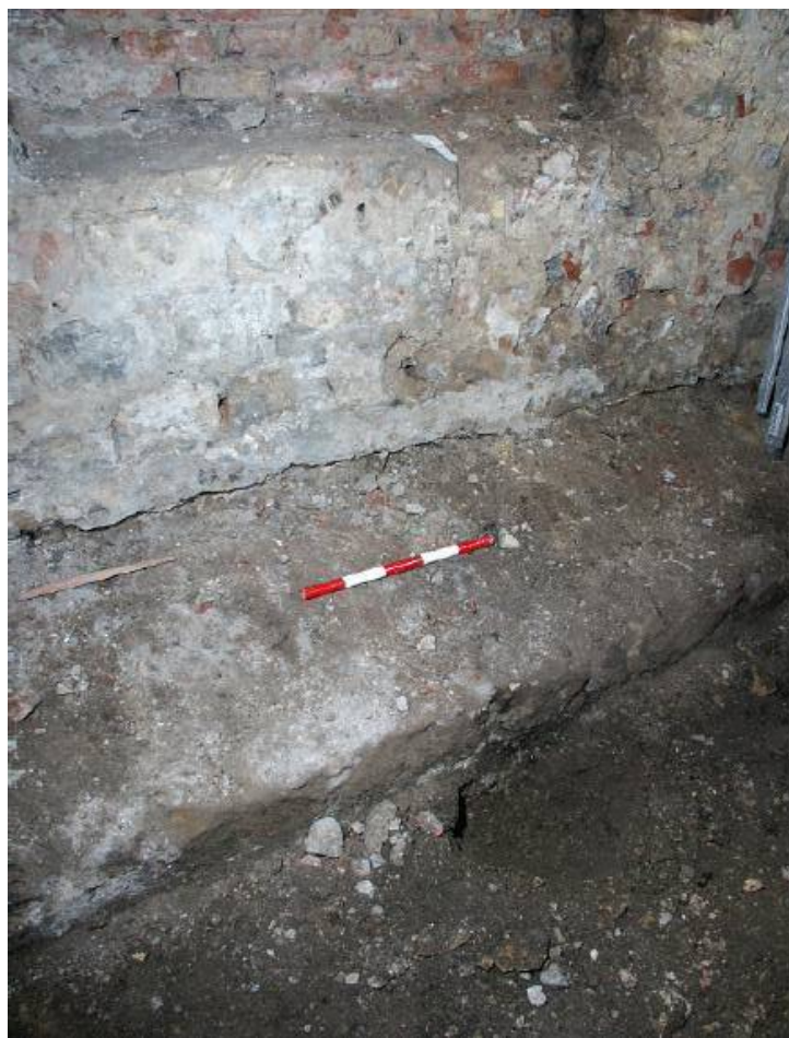
Fig. 24 12 Minster Yard. Magnesian limestone foundations of the Archbishop's Exchequer (in Dean, '12 Minster Yard', p. 17).
