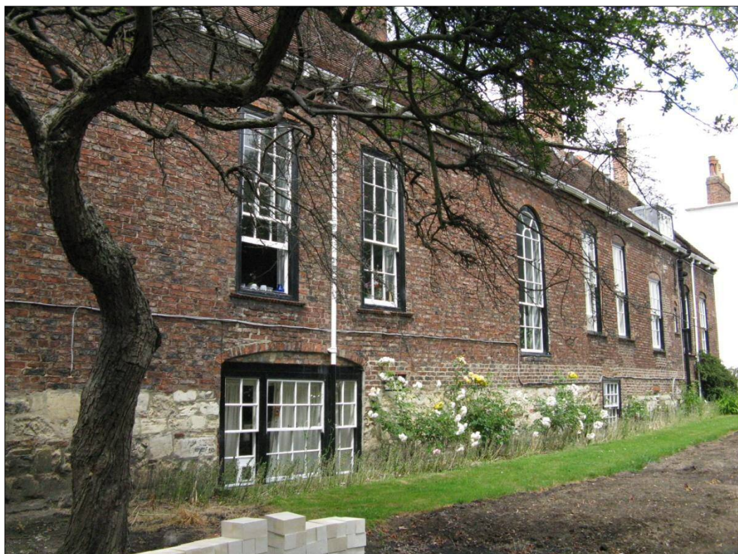
Fig. 53 N. 3 Minster Court , showing the south range of the Mansion of Ullerskelf, with medieval stone wall and a brick phase , visible right above the stone courses, possibly representing the 16 th C development.
