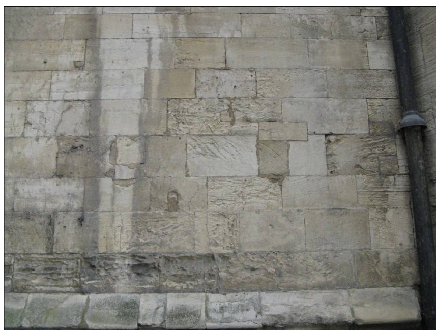
Fig. 32 Mortice scars on the eastern face of the second buttress of the Chapter House.
