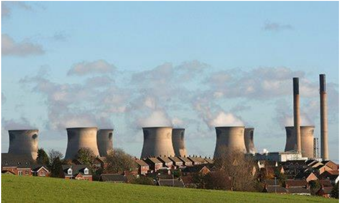
Figure 9 Iconic Ferrybridge C Power Station
