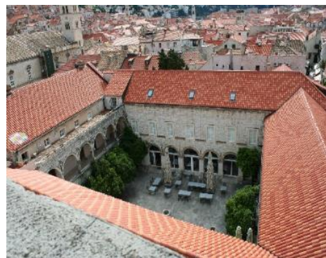
Figure 7.16 St Claire's Roof and Courtyard
