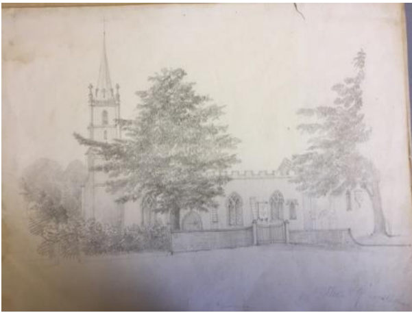
Figure 137 : 'All Saints', Stone, Drawn c1870. Photo: R Dellow. Source: Gloucestershire Archives (P315/MI/2).
