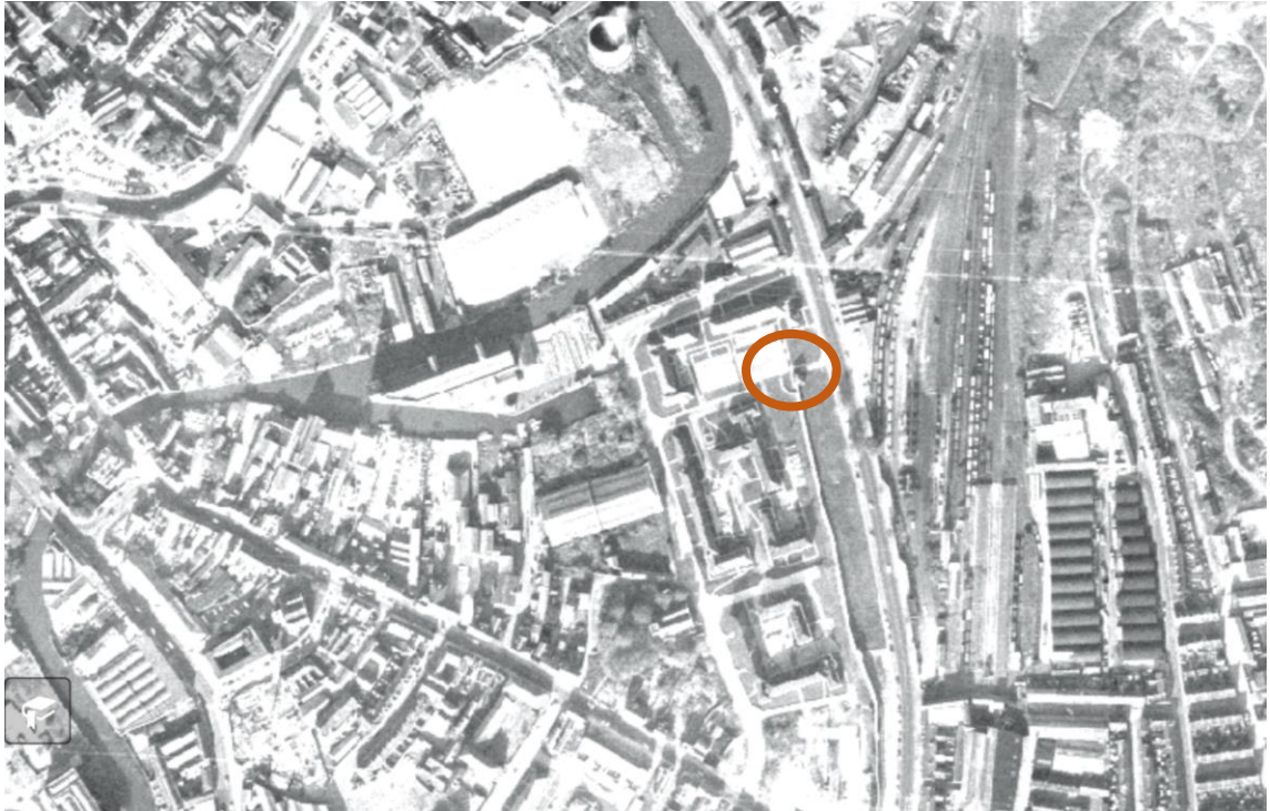
Figure 67. View of Red Tower, Walmgate and Foss Islands, 1962 Aerial photograph. York View (2017a). © OS 2017.
